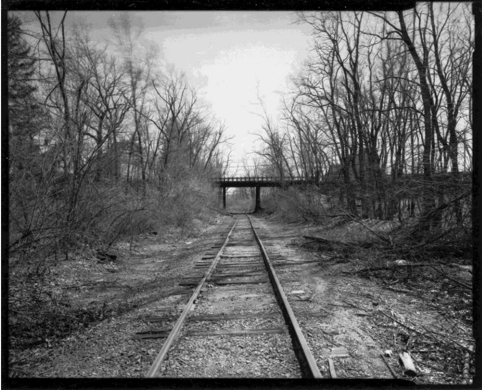
NH-714-3: North elevation and context from railroad tracks. Looking south.
