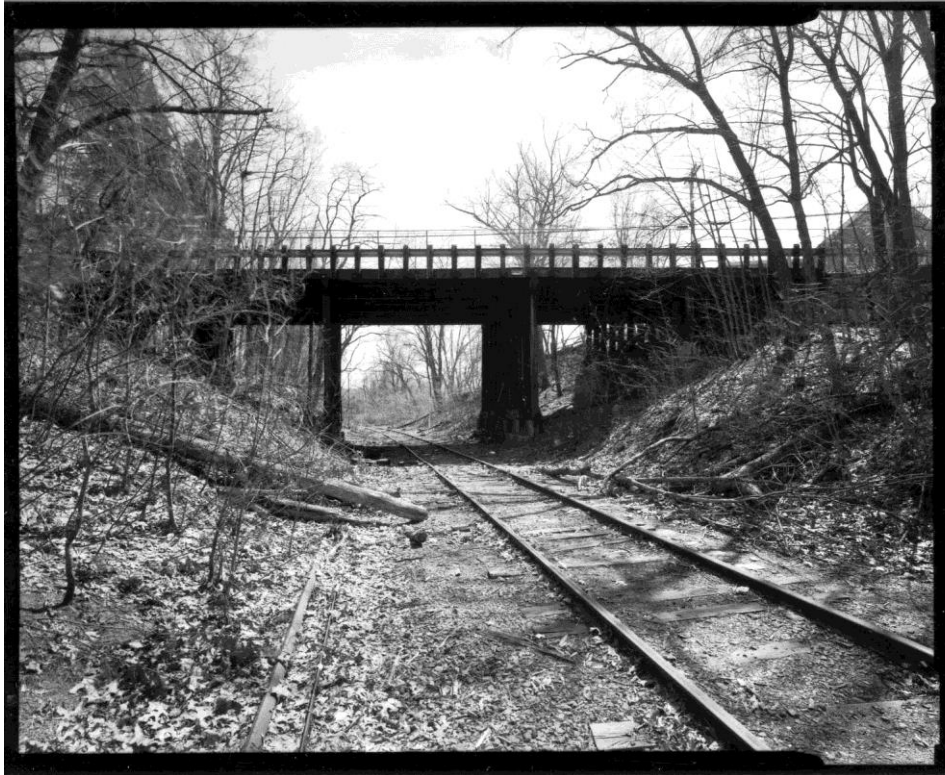
NH-714-6: North elevation. Looking south.
