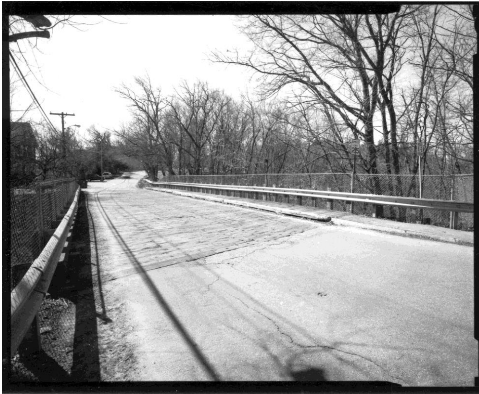
NH-714-4: Deck view. Looking west.
