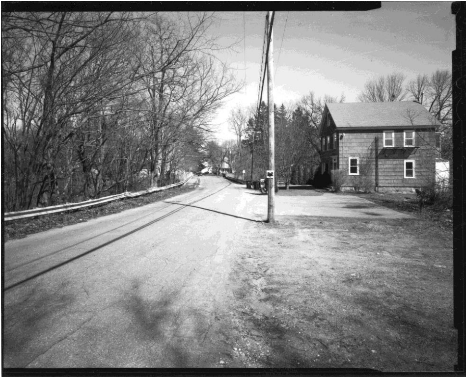
NH-714-1: West approach to bridge in context from Fairmount Street. Looking east.
