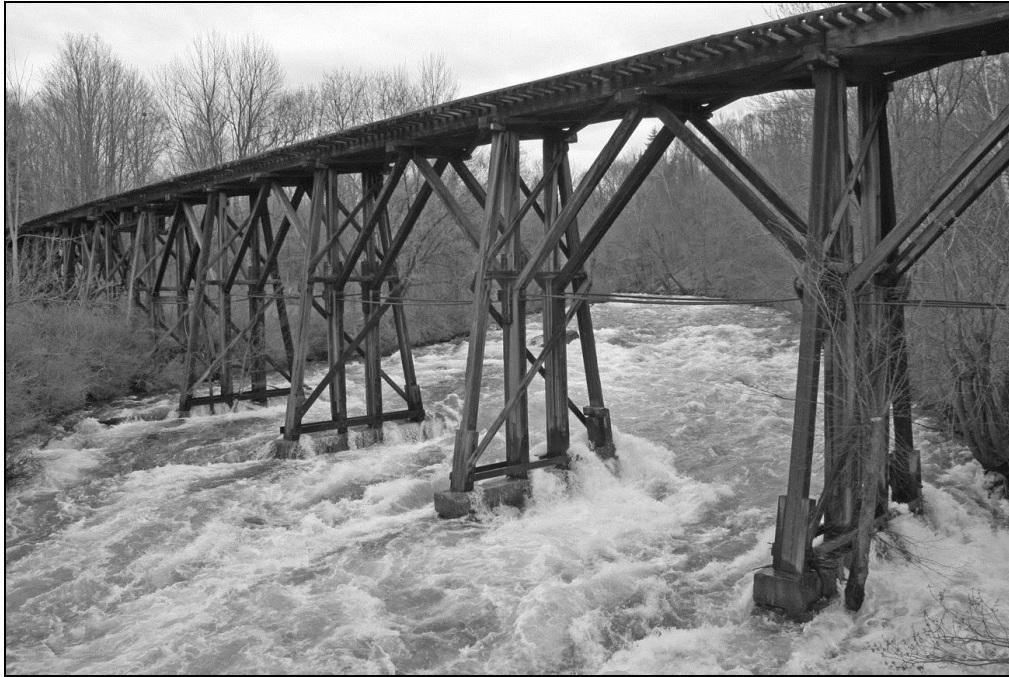
FIGURE 15: B&MRR Knee-braced railroad trestle over Winnepesaukee River, Franklin NH.
