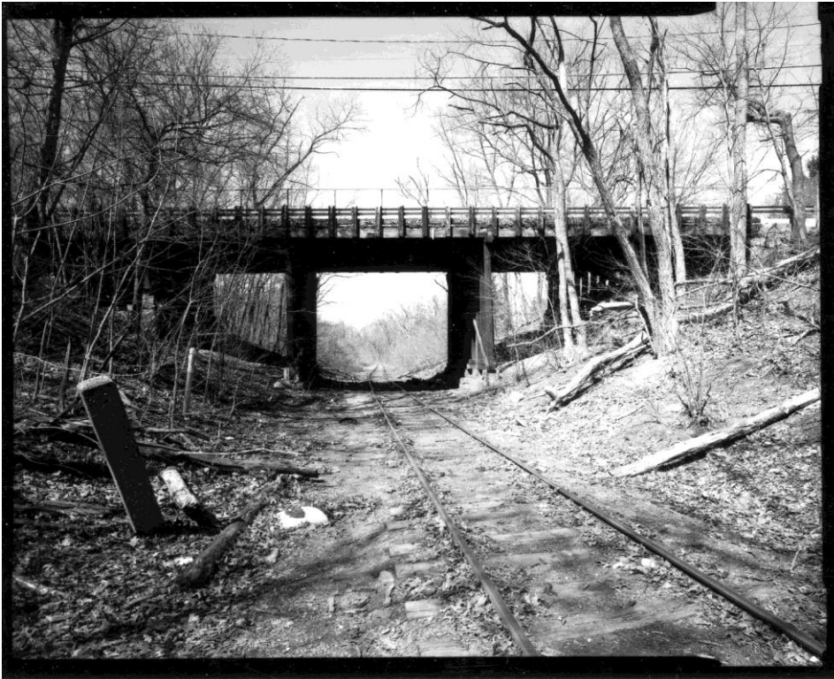
NH-714-5: South elevation. Looking north.
