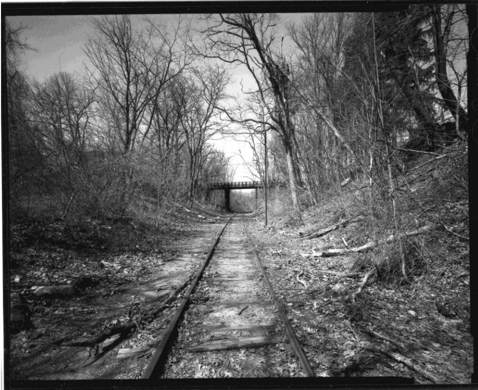
NH-714-2: South elevation and context from railroad tracks. Looking north.
