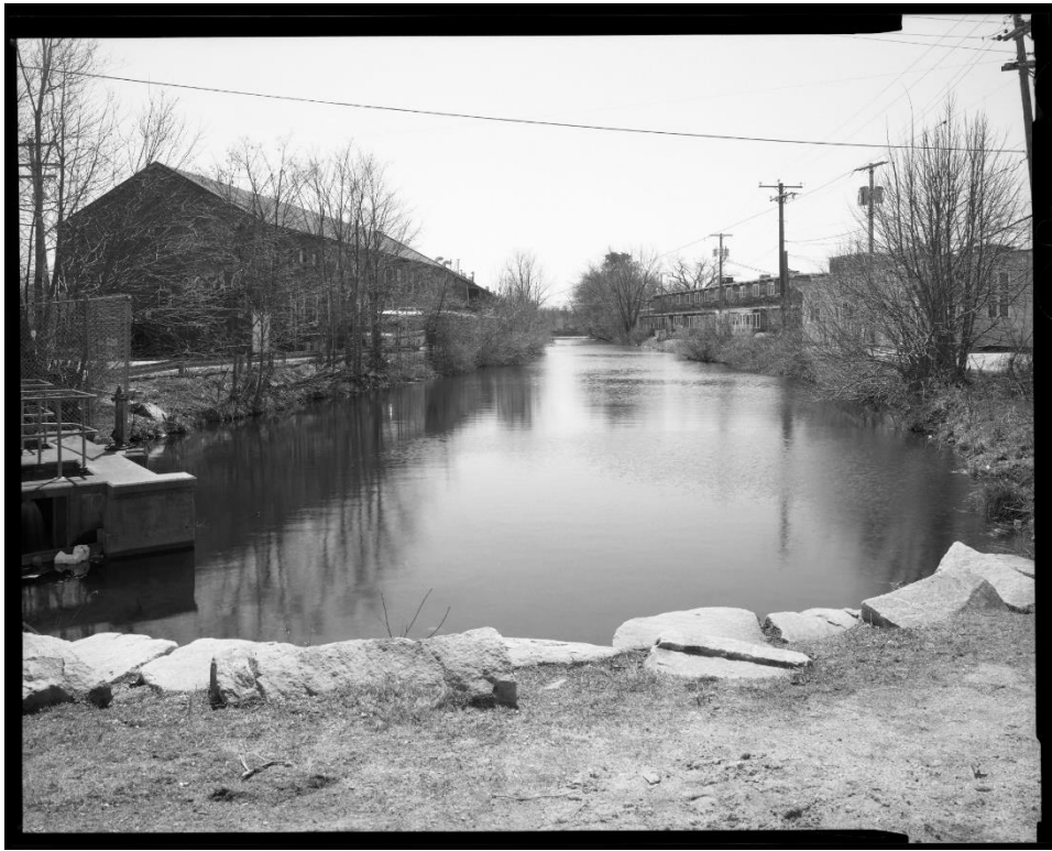
NH-538-G-2: North end of Power Canal with stone termination wall in foreground, overflow structure and Storehouse No. 2 at left, and canal channel running south. Looking south.
