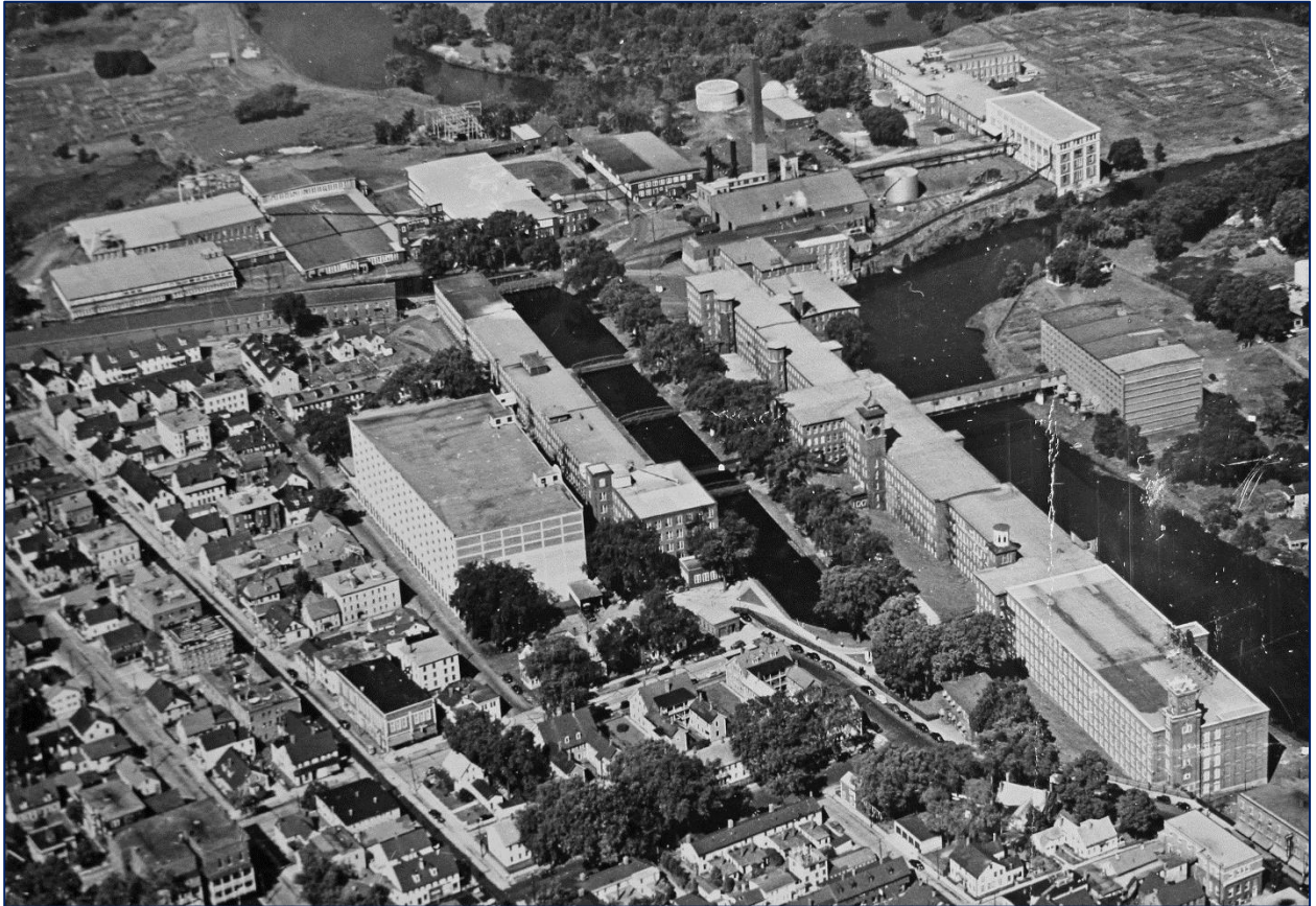
FIGURE 19: Aerial photograph of Nashua Manufacturing Co. circa 1940, showing Canal Basin before 1972 alterations to site that removed and or buried all of its features. Note bridges over Basin still extant at that time and massive eight story South Concrete Cloth Store House (near center of photo) occupying the open park area shown on the 1883 map (Figure 8). (Source: Nashua Historical Society photograph collection).
