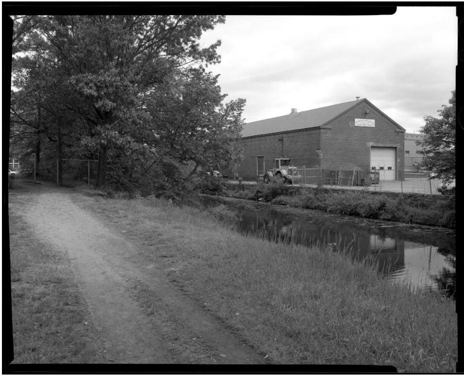
NH-538-G-3: Section of Power Canal at south end of Storehouse No. 2, showing earth bank on west side and stone wall along east side. Looking northeast.
