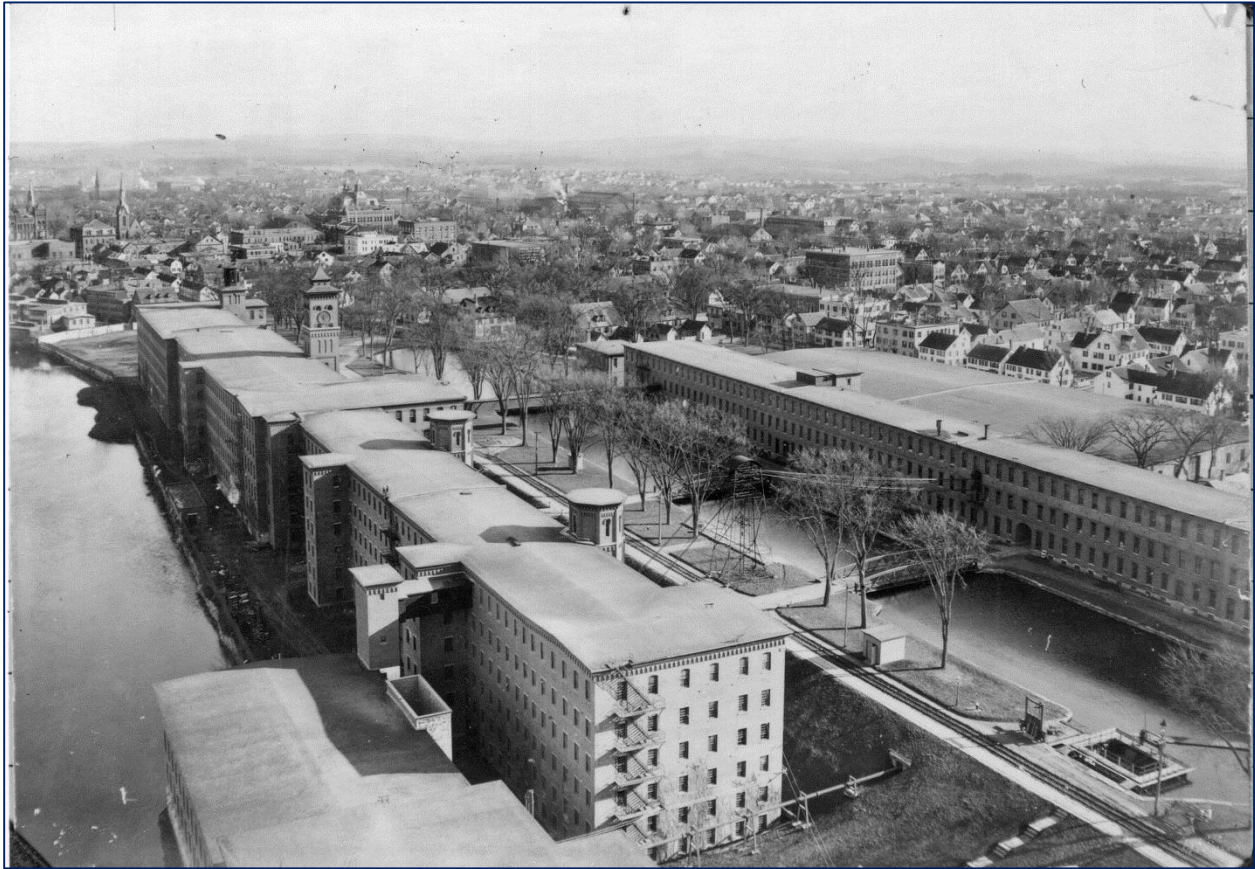
FIGURE 15: Photograph of Nashua Manufacturing Co. circa 1898, evidently taken from scaffolding for Boiler House chimney construction, looking east and showing: Canal Basin extending east in front of main mill buildings along Basin Street; bowstring truss bridges spanning Basin; original Waste Way overflow structure at lower right; land cleared and fenced at east end of main mill buildings for construction of Mill No. 7 and east end of Basin prior to construction of penstock and gate for Mill No. 7 (see Figures 17 and 18). (Source: Frank Ingalls, Photographer; Ingalls Photograph Collection, Nashua Historical Society).
