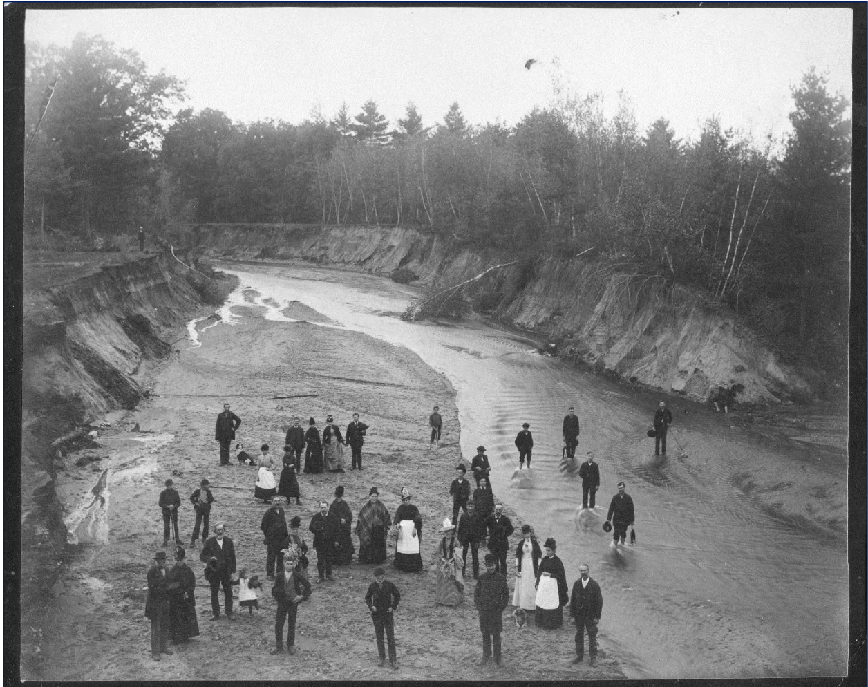
FIGURE 9: Photograph of canal break of 6 October 1887, showing hole in canal wall visible at far right, and curious folks posed in nearly dry canal bed. (Source: Nashua Historical Society photograph collection).
