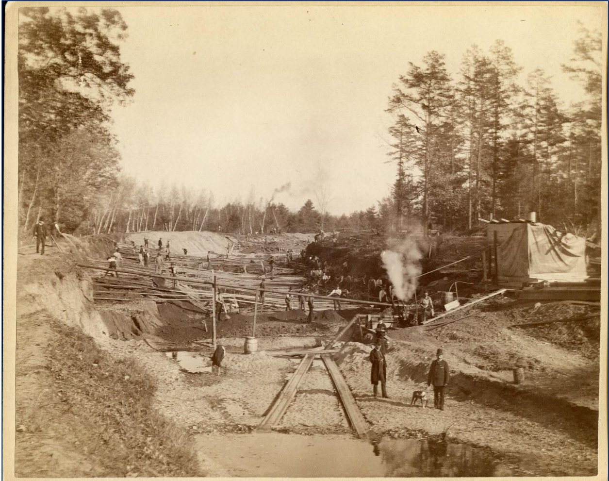
FIGURE 10: Photograph of repair work to canal following break of 6 October 1887, showing: work realigning canal, here reducing curvature by cutting fill from bank on inside of curve (on right) and filling opposite bank; use of steam engine (in tent) to power water pump (under steam plume) used to dewater canal and provide water to compact fill. (Source: Nashua Historical Society photograph collection).
