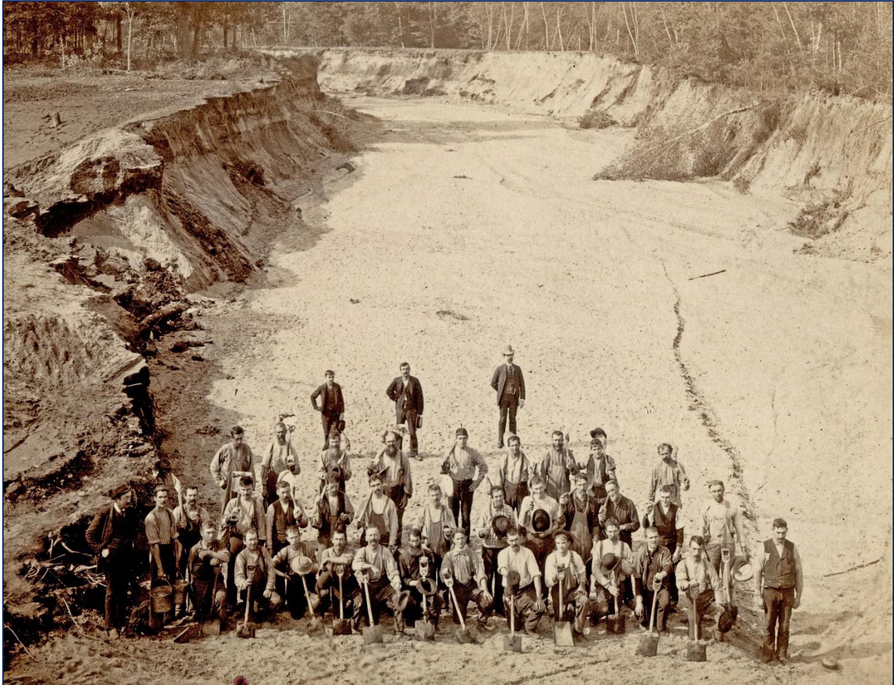
FIGURE 12: Photograph of repair work to canal following break of 6 October 1887, showing team of laborers all holding shovels posing in dry canal bed. (Source: Nashua Historical Society photograph collection).
