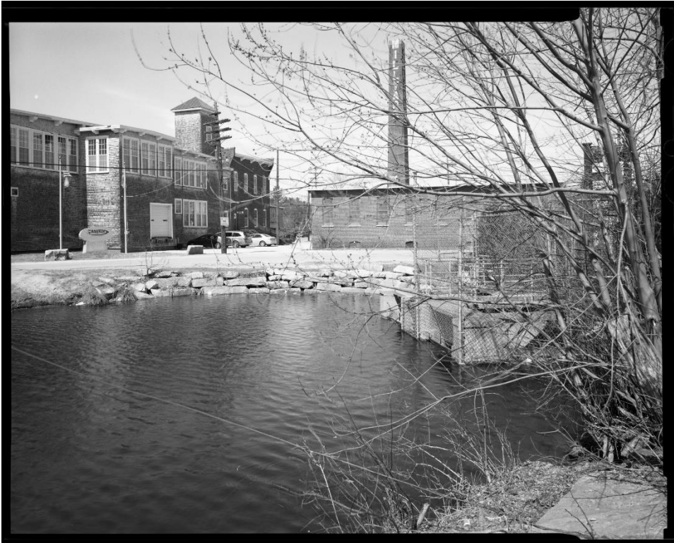
NH-538-G-1: North end of Power Canal showing stone termination wall and concrete overflow structure at right. Looking north.
