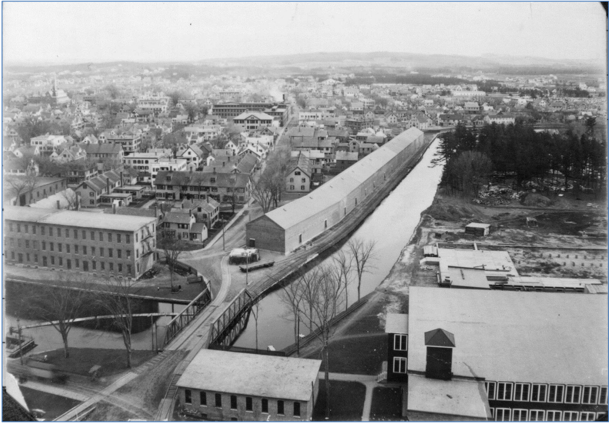
FIGURE 14: Photograph of Nashua Manufacturing Co. circa 1898, evidently taken from scaffolding for Boiler House chimney construction, looking south and showing: Canal alongside Storehouse No. 2; Pine Street spanning canal on pony truss bridge (replacing earlier pile bent bridge) and Waste House, in foreground; portion of original Waste Way overflow structure, located on north side of Canal Basin at west end, just visible in lower left. (Source: Frank Ingalls, Photographer; Ingalls Photograph Collection, Nashua Historical Society).
