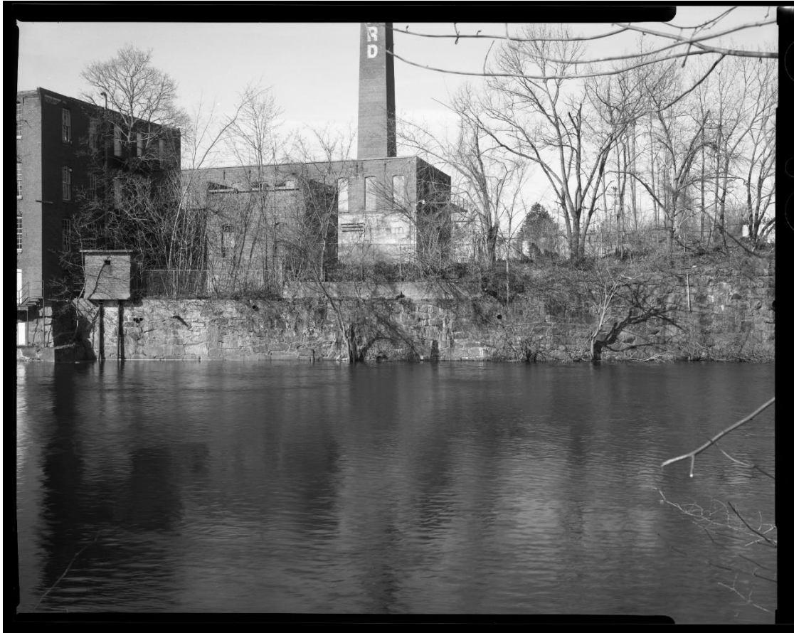
NH-538-F-3: Elevation of south section of wall. Looking west.
