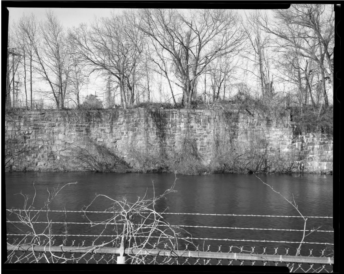
NH-538-F-4: Elevation of middle section of wall. Looking west.
