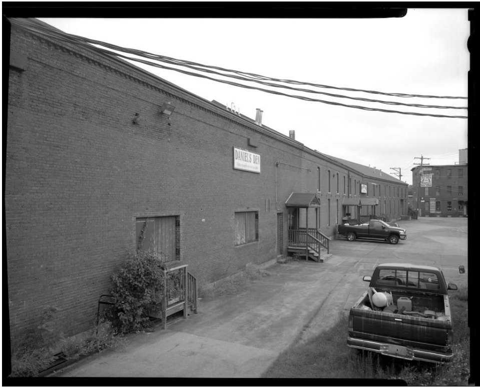
NH-538-H-3: Oblique view of east side of Store House No. 2, showing Sections 2, 1, and 4, left to right. Looking north.
