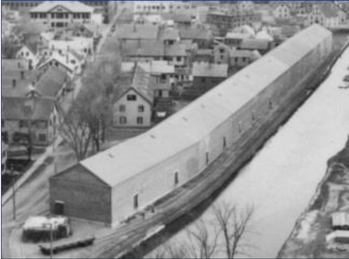
FIGURE 7: Photograph of Nashua Manufacturing Co. circa 1898, evidently taken from scaffolding for Boiler House chimney construction, showing fully completed Storehouse No. 2 prior to installation of windows in Sections 1 and 4. (Source: Nashua Historical Society).
