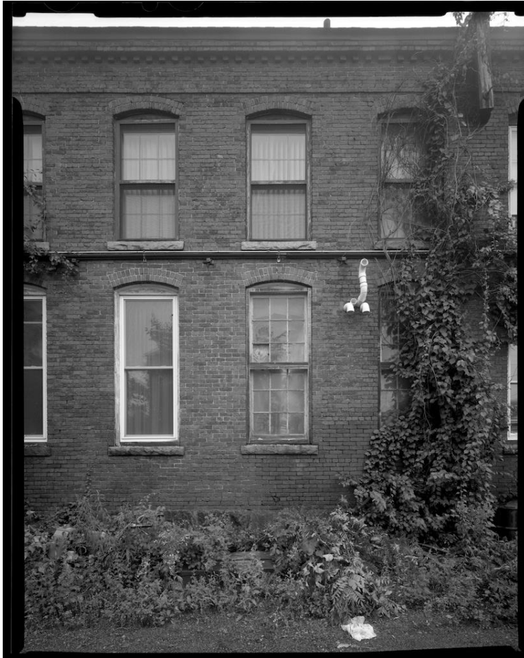
NH-538-H-8: West (Canal side) elevation of portion of Store House No. 2, Section 4. Looking east.
