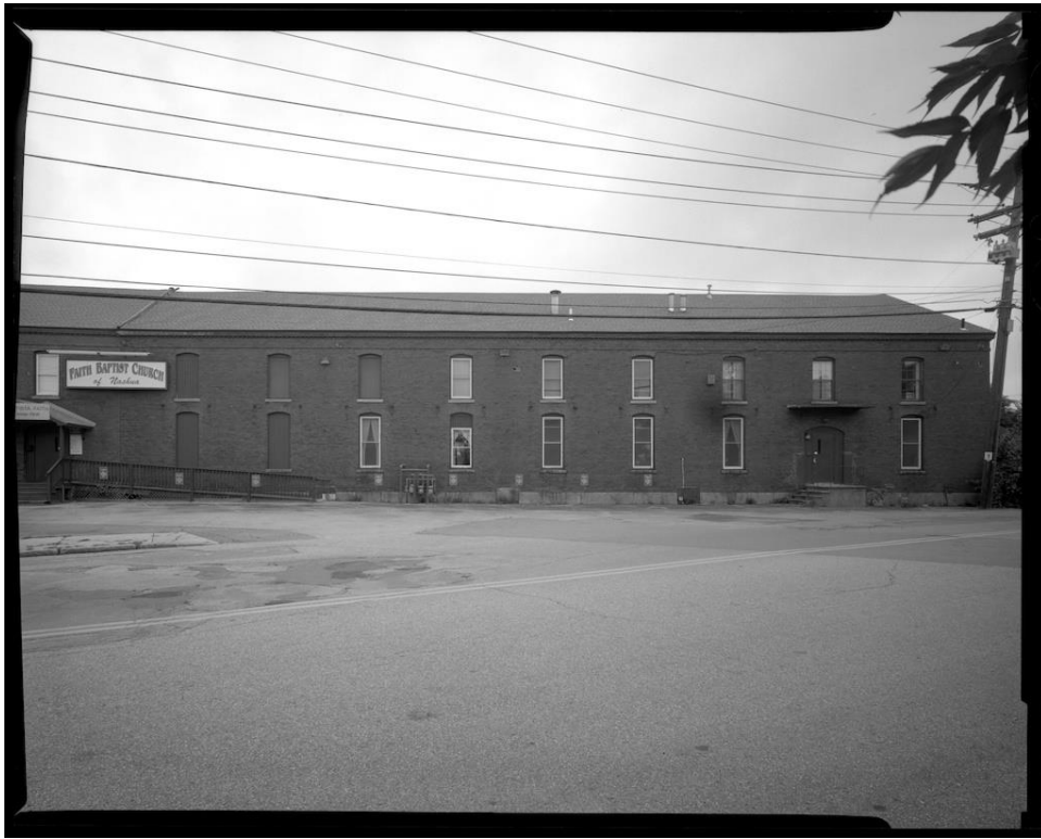
NH-538-H-4: East (Pine Street) elevation of Section 4. Looking west.
