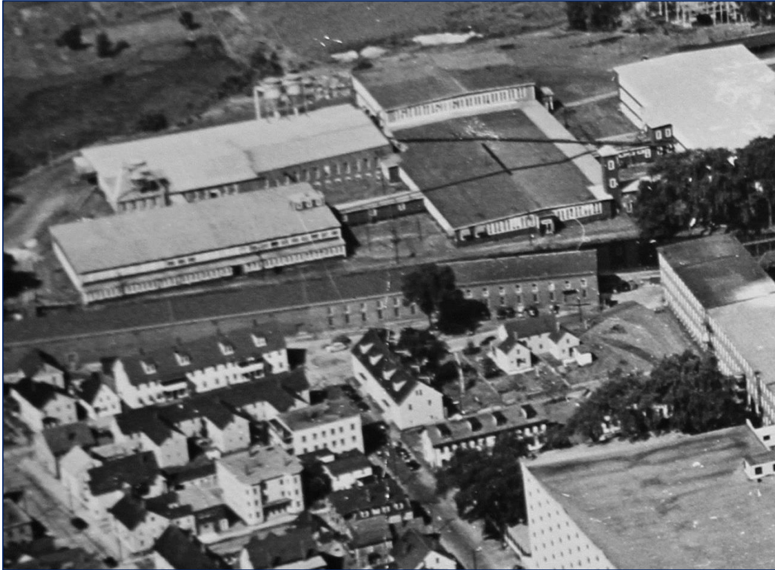
FIGURE 12: Aerial photograph of Nashua Manufacturing Co. circa 1940, showing windows installed in Storehouse No. 2, Sections 1 and 4. (Source: Nashua Historical Society).
