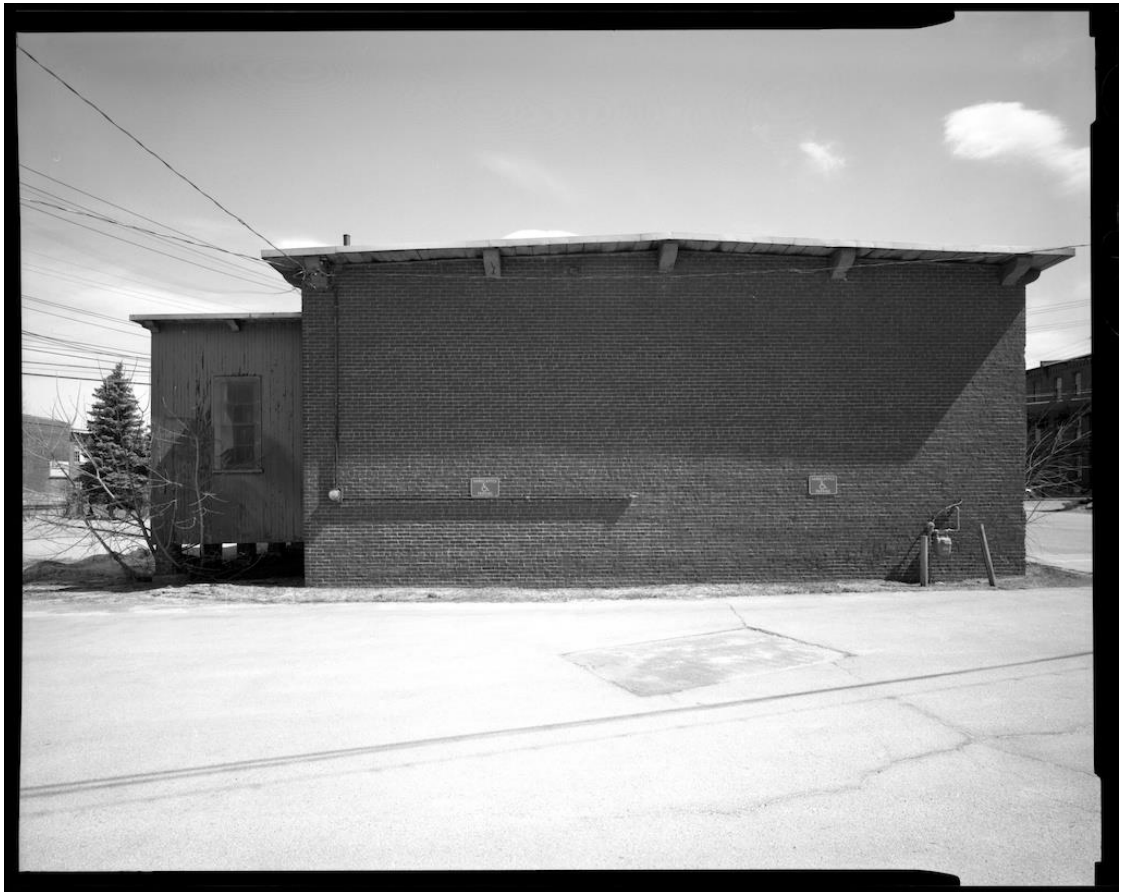
NH-538-J-5: Rear elevation (west). Looking east.
