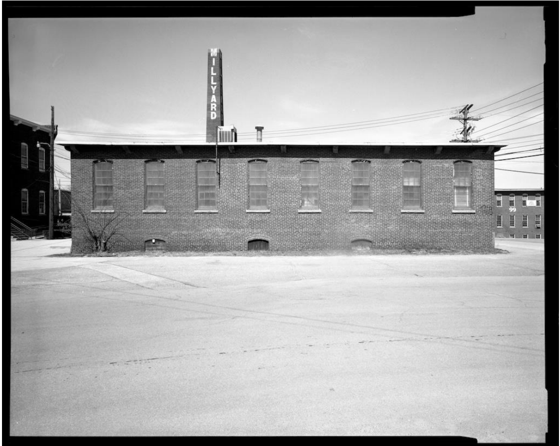
NH-538-J-6: South side elevation. Looking north.
