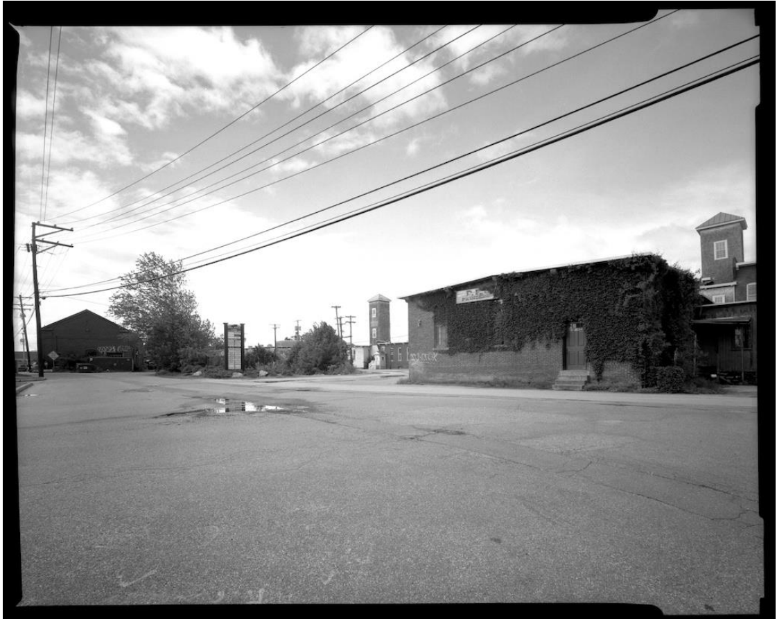
NH-538-J-1: Context with Pine Street. Looking southwest.
