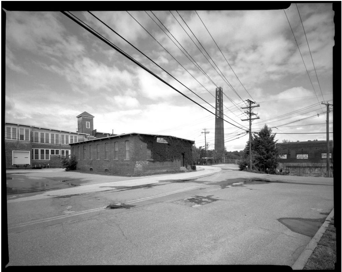
NH-538-J-2: Context, showing Pine Street Extension and Boiler House Smokestack in background. Looking northwest.
