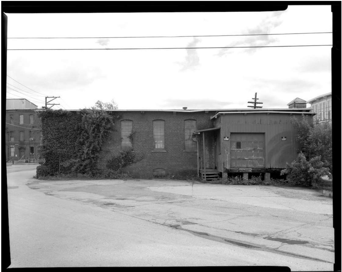
NH-538-J-4: North side elevation, showing loading dock. Looking south.
