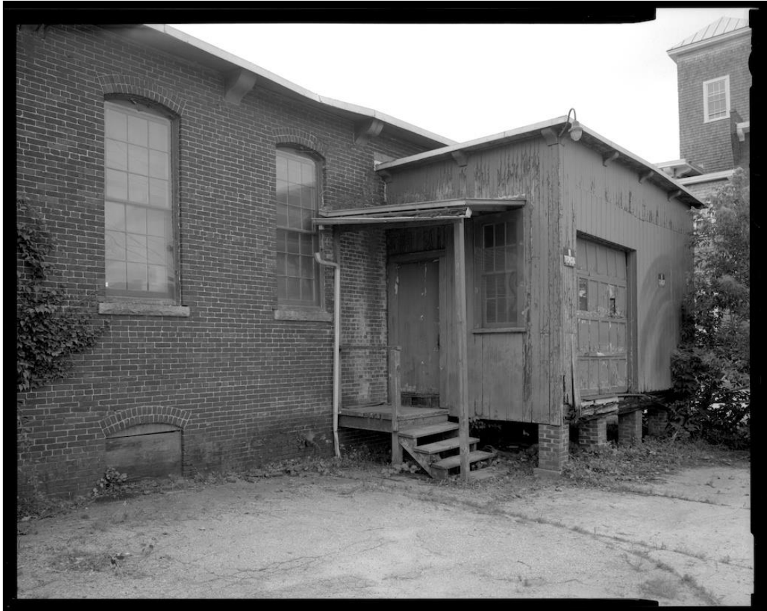
NH-538-J-7: North side, showing detail of loading dock. Looking southwest.
