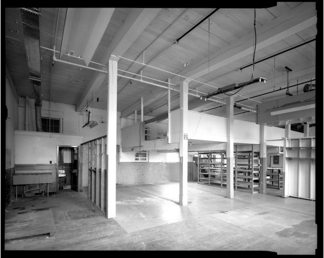
NH-538-J-8: Interior view from southwest corner. Looking northeast.
