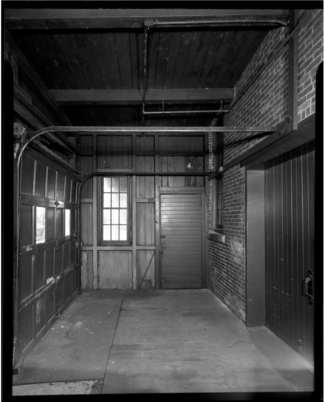
NH-538-J-10: Interior view of loading dock from west end. Looking east.
