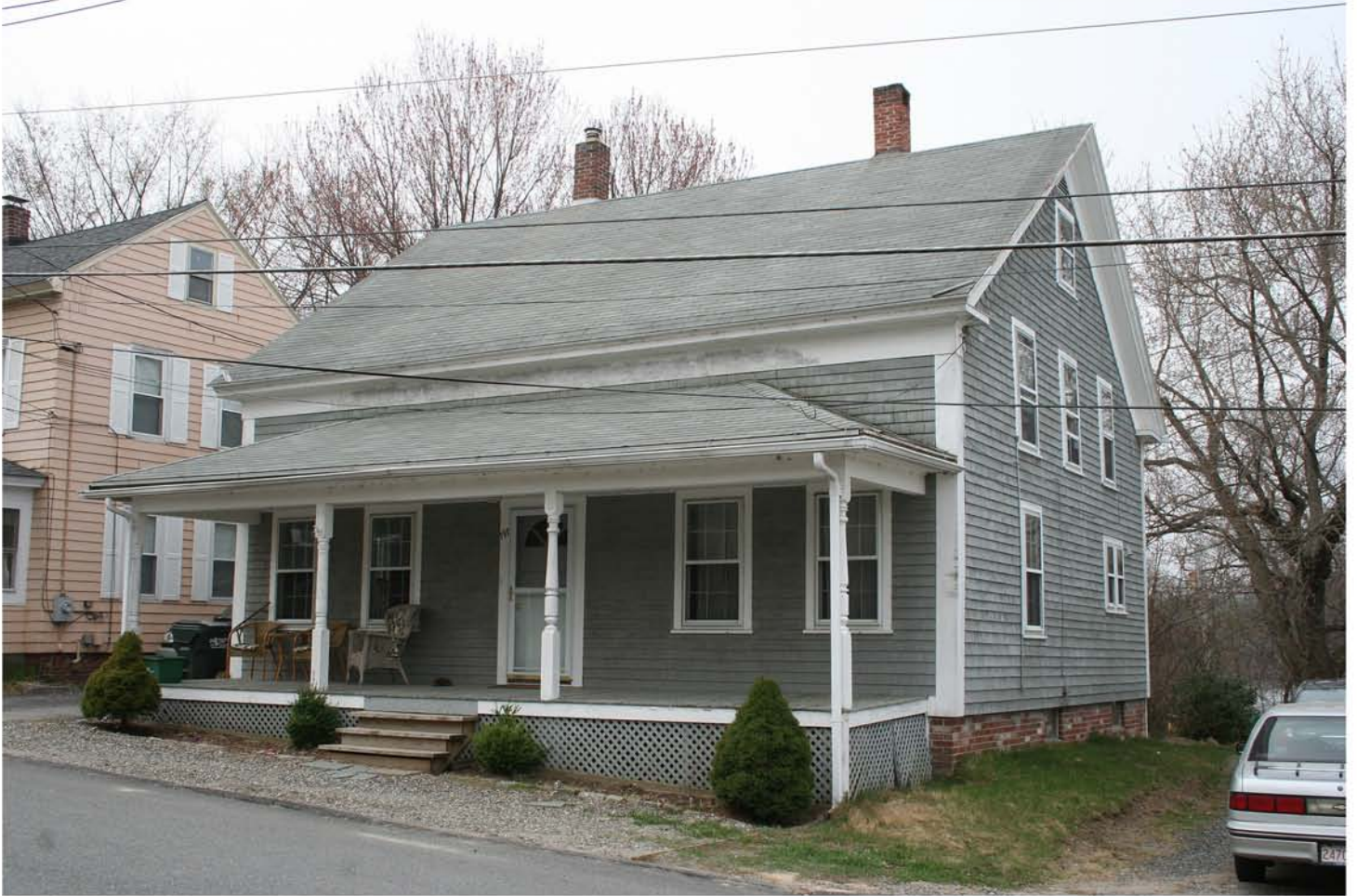
14. Mill Housing 197 High Street, view west
