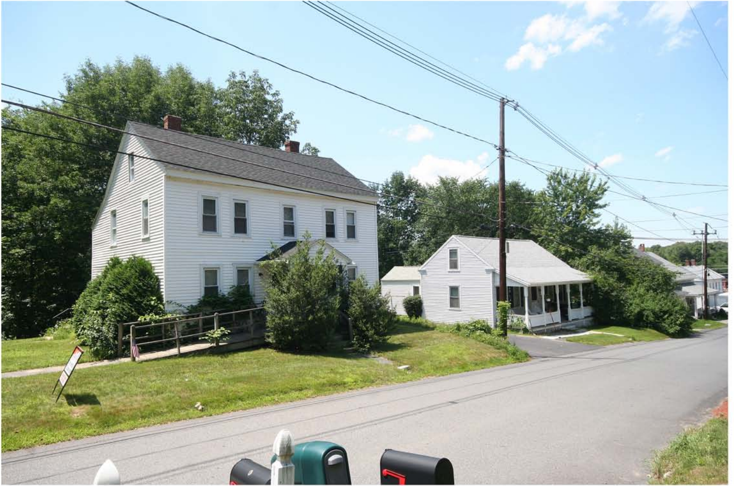
3. Context, High Street, view west
