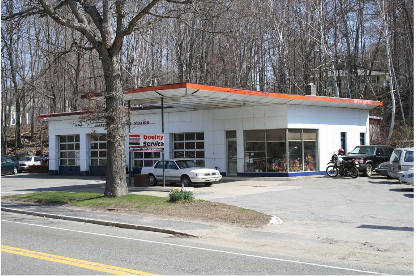
22. Jefferson Service Station, view northeast
