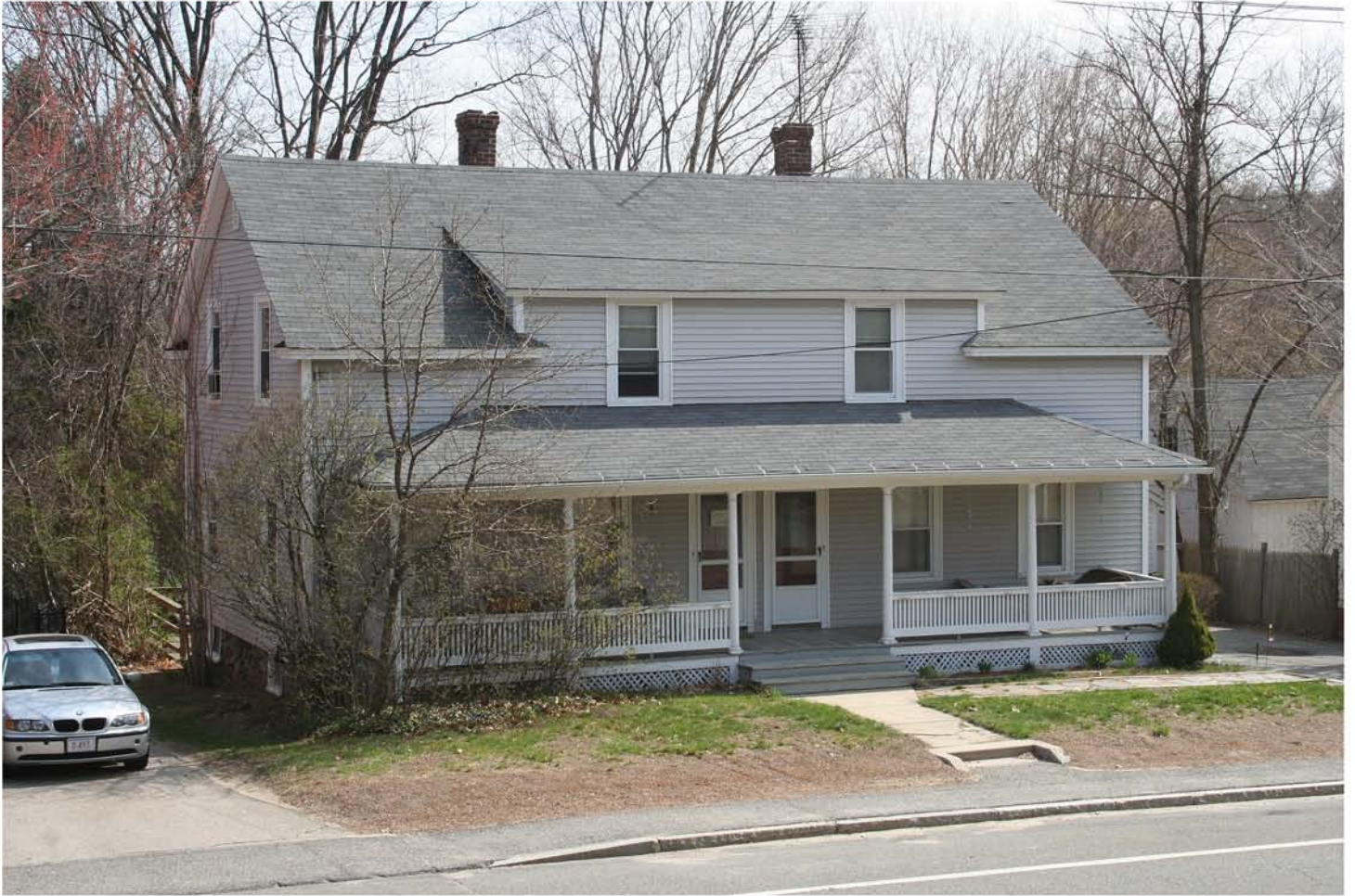
17. Duplex Mill Housing 1712-14 Main Street, view northeast
