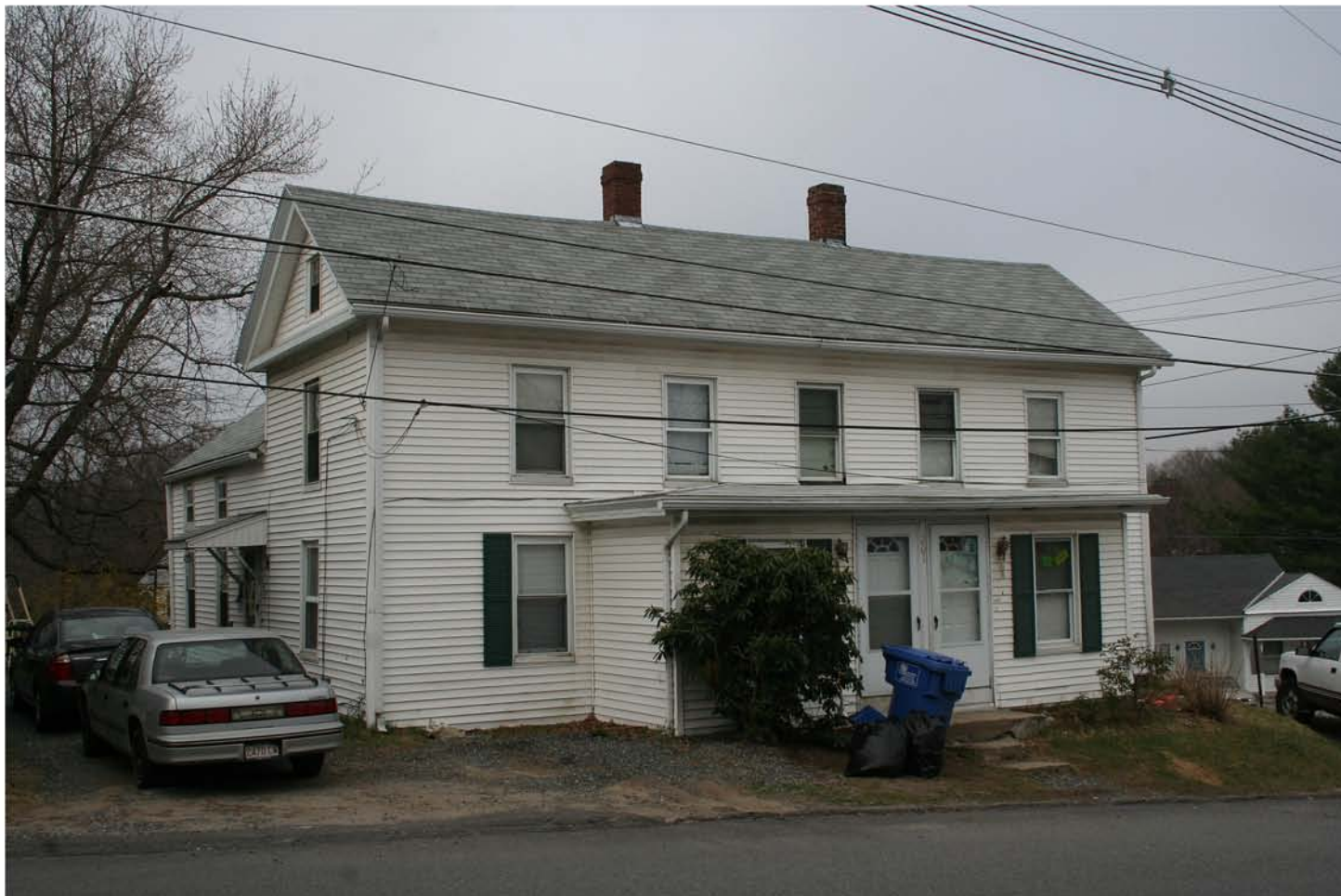
13. Mill Housing 201 High Street, view west
