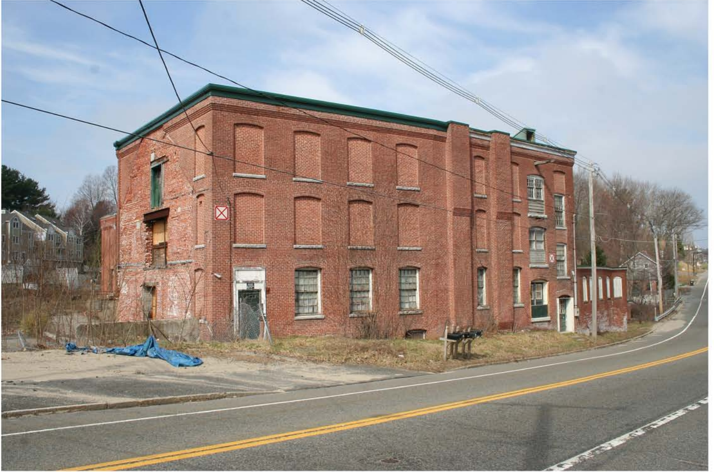
9. Jefferson Mfg. Co. Building No. 3, view northwest
