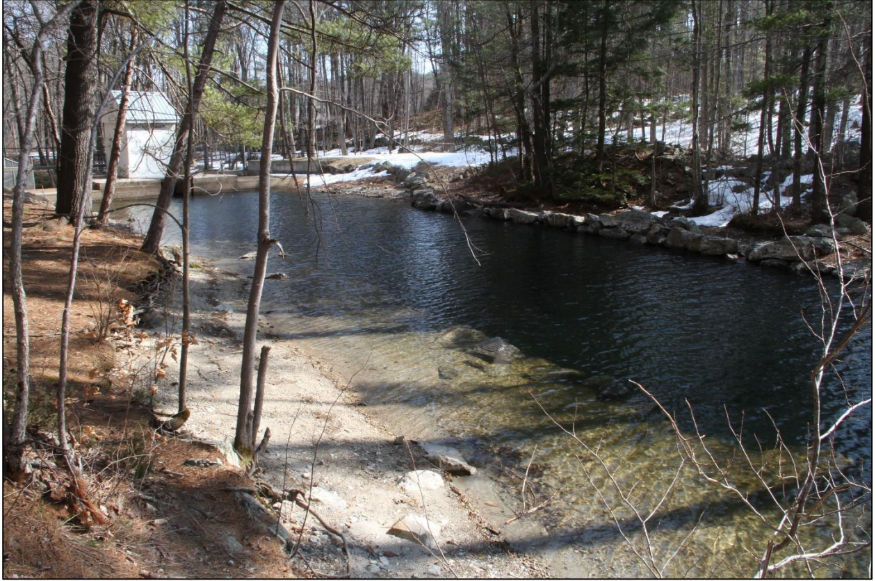
Photo No. 8: Upper Canal and Great East Lake Dam. Looking S.
