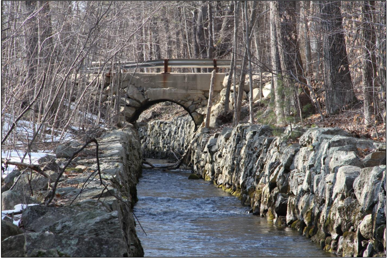
Photo No. 2: Lower Canal and Stone Arch Bridge. Looking NW.
