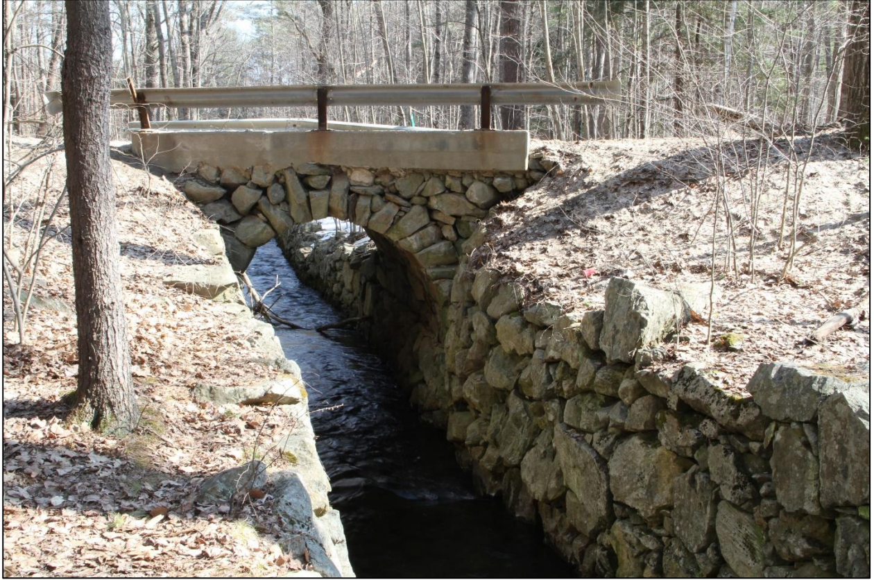
Photo No. 3: Stone Arch Bridge. Looking S.
