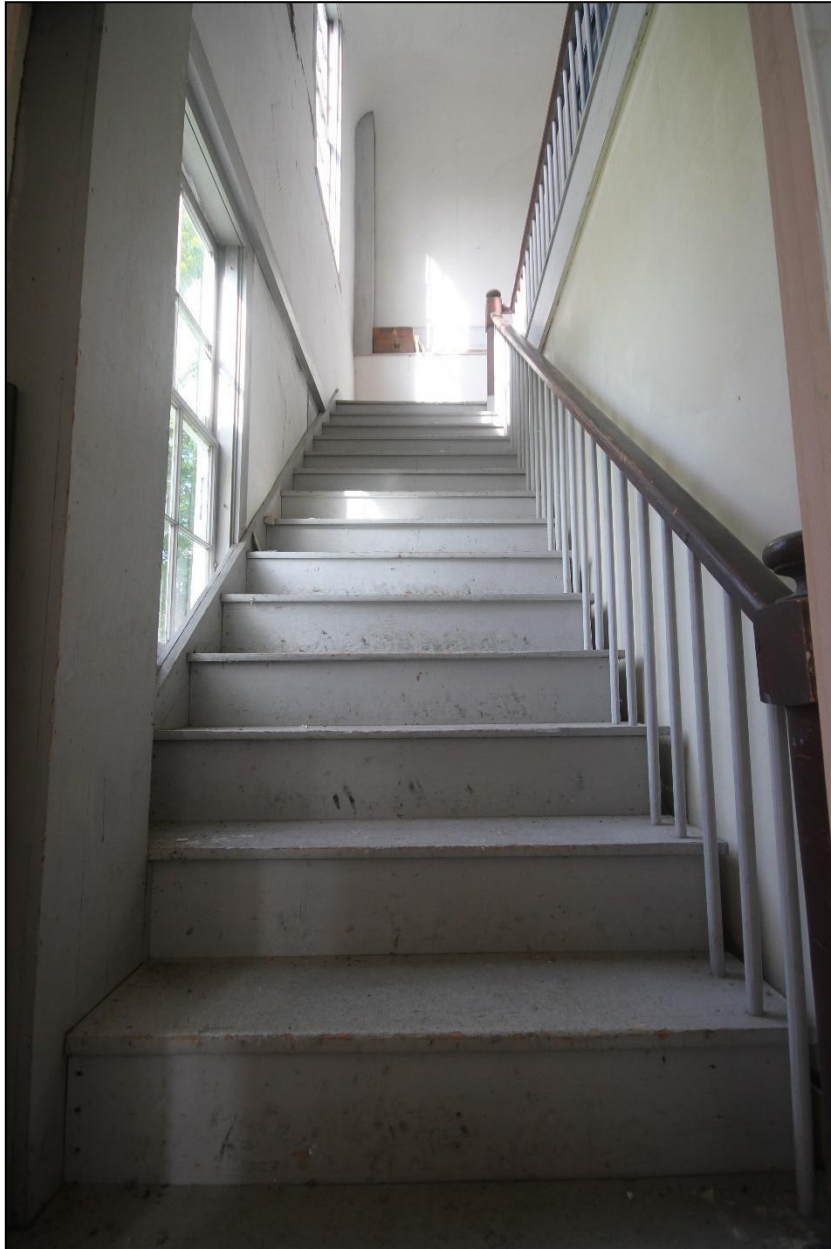
NH_Langdon_SullivanCo_LangdonMeetingHouse_0013: Interior, first floor, north staircase. Looking North.
