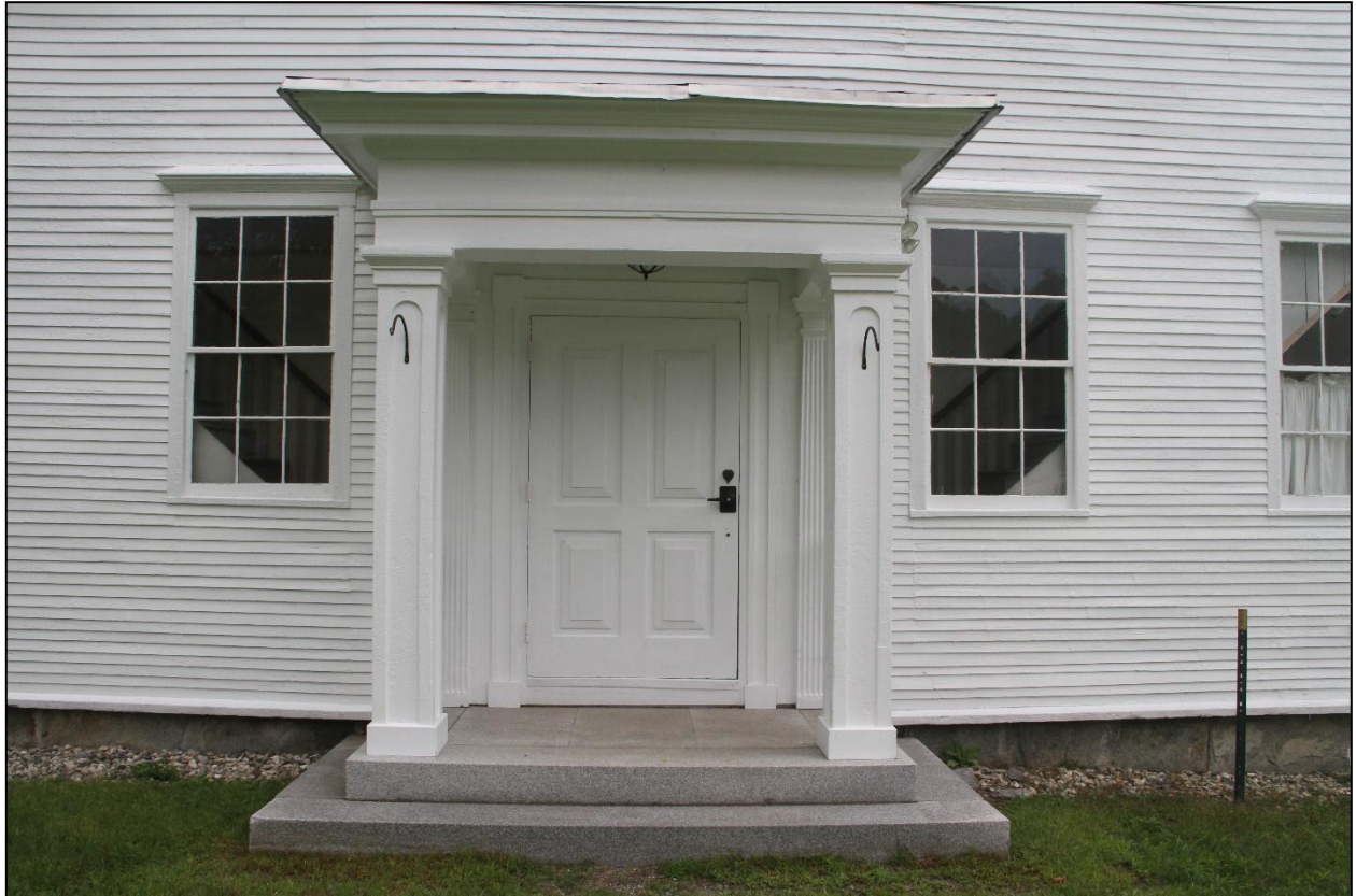
NH_Langdon_SullivanCo_LangdonMeetingHouse_0009: West entry. Looking East.
