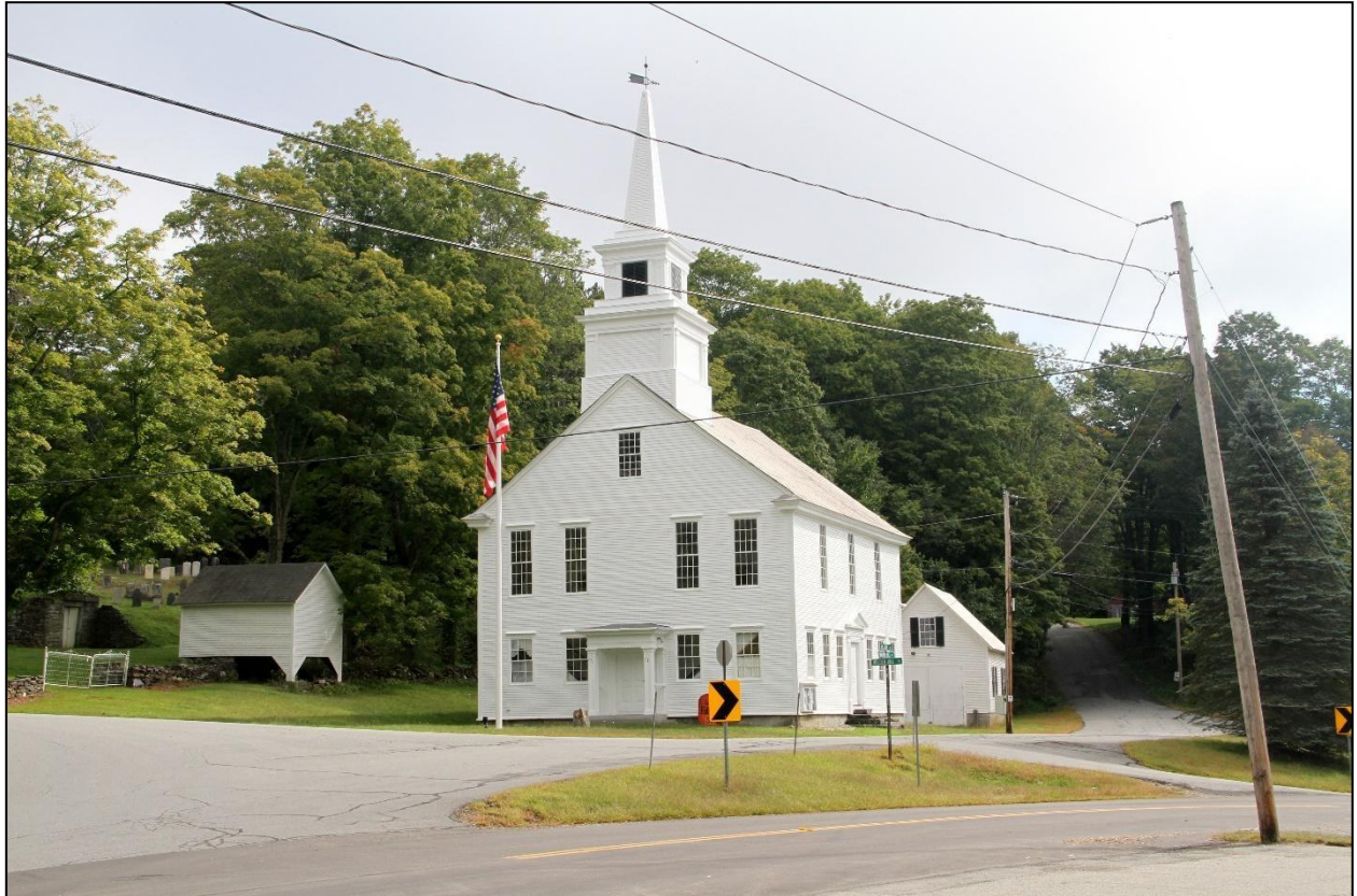
NH_Langdon_SullivanCo_LangdonMeetingHouse_0002: Overview of south and west sides. Looking East.
