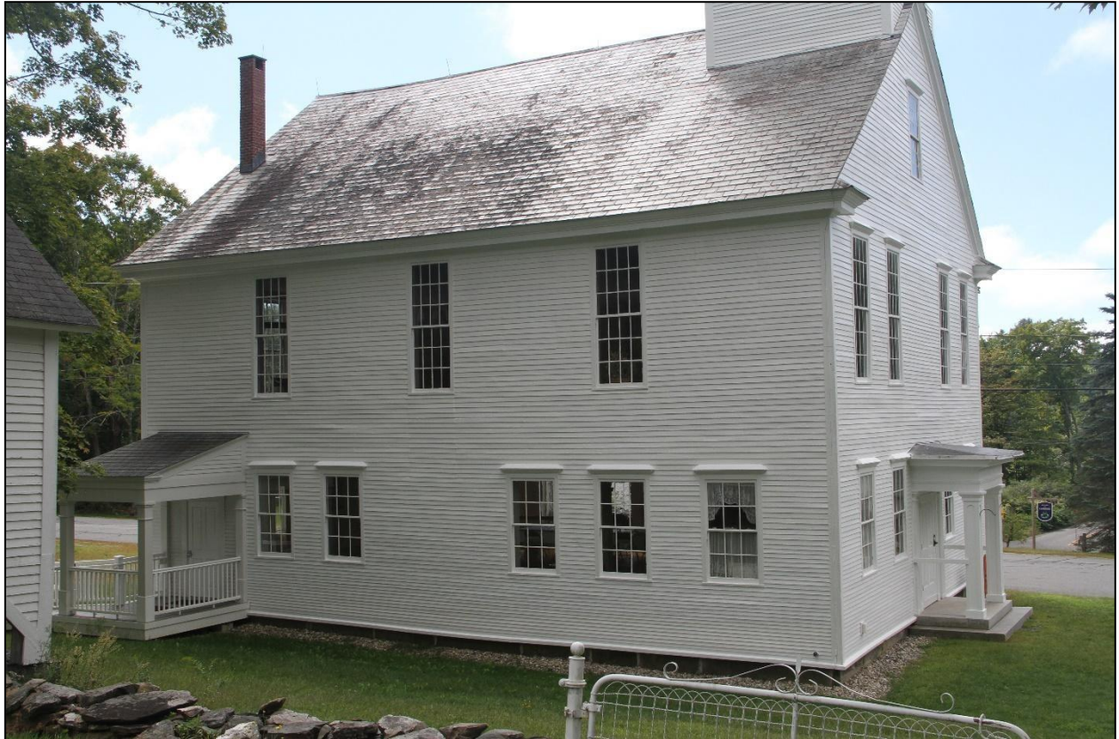
NH_Langdon_SullivanCo_LangdonMeetingHouse_0005: North side, showing ADA accessible sheltered entry at left. Looking South.
