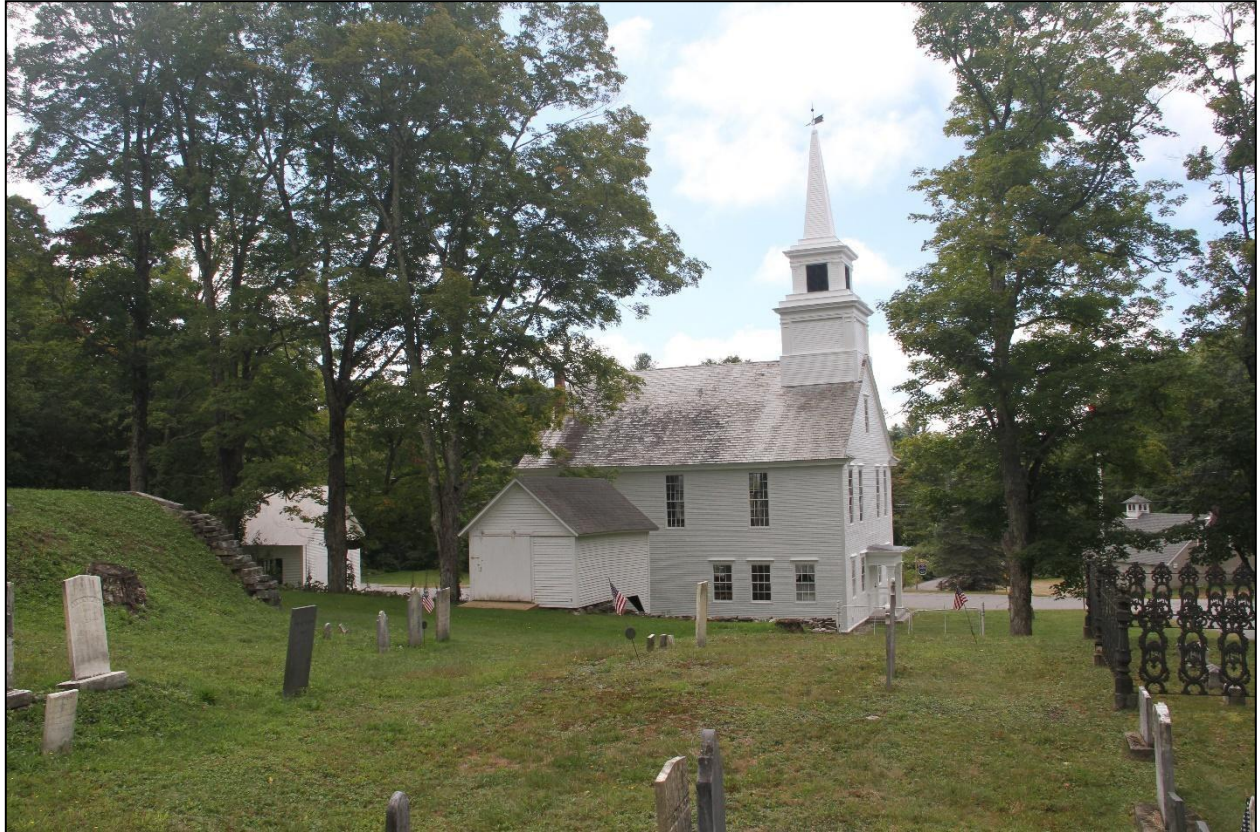
NH_Langdon_SullivanCo_LangdonMeetingHouse_0004: Overview of west and north sides from cemetery. Looking South.
