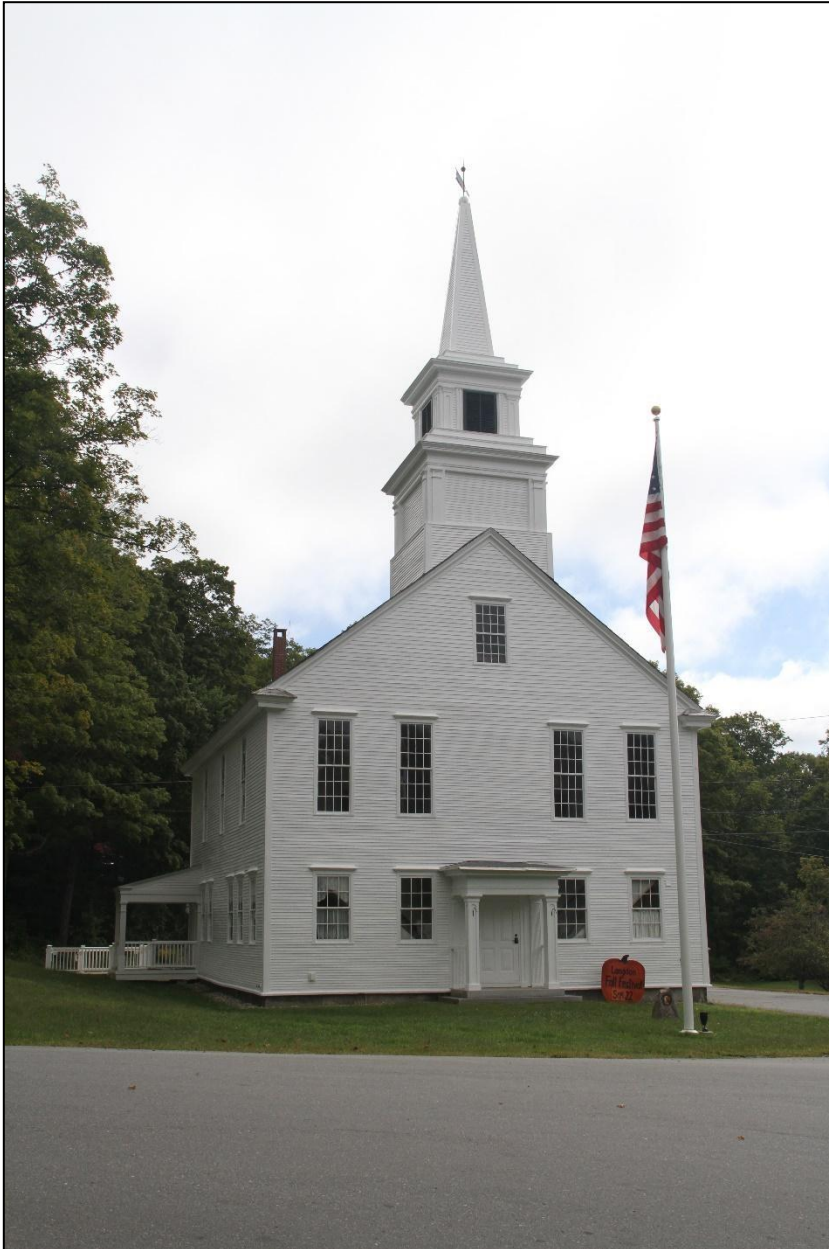
NH_Langdon_SullivanCo_LangdonMeetingHouse_0003: West side. Looking East.
