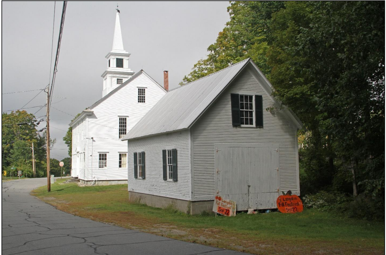
NH_Langdon_SullivanCo_LangdonMeetingHouse_0007: Salt Shed, east and south sides, with Meeting House in background. Looking West.
