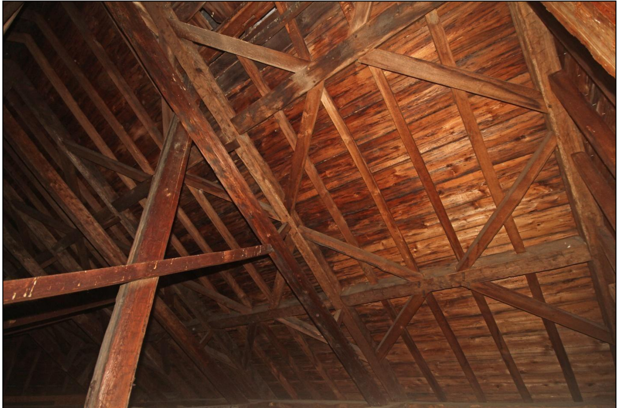
NH_Langdon_SullivanCo_LangdonMeetingHouse_0020: Attic, showing timber roof framing. Looking East.
