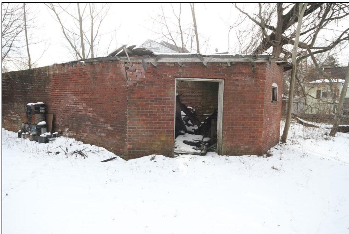
Photo No. 14: Storehouse (c.1893), west and north elevations. Looking SE.
