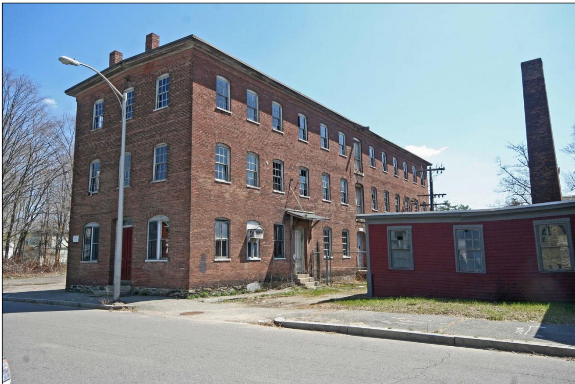
Photo No. 6: Factory (1880), West (Porter St.) and south elevations. Looking E.
