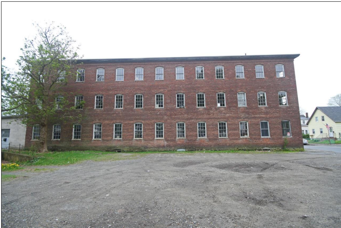
Photo No. 8: Factory, north elevation. Looking SW.
