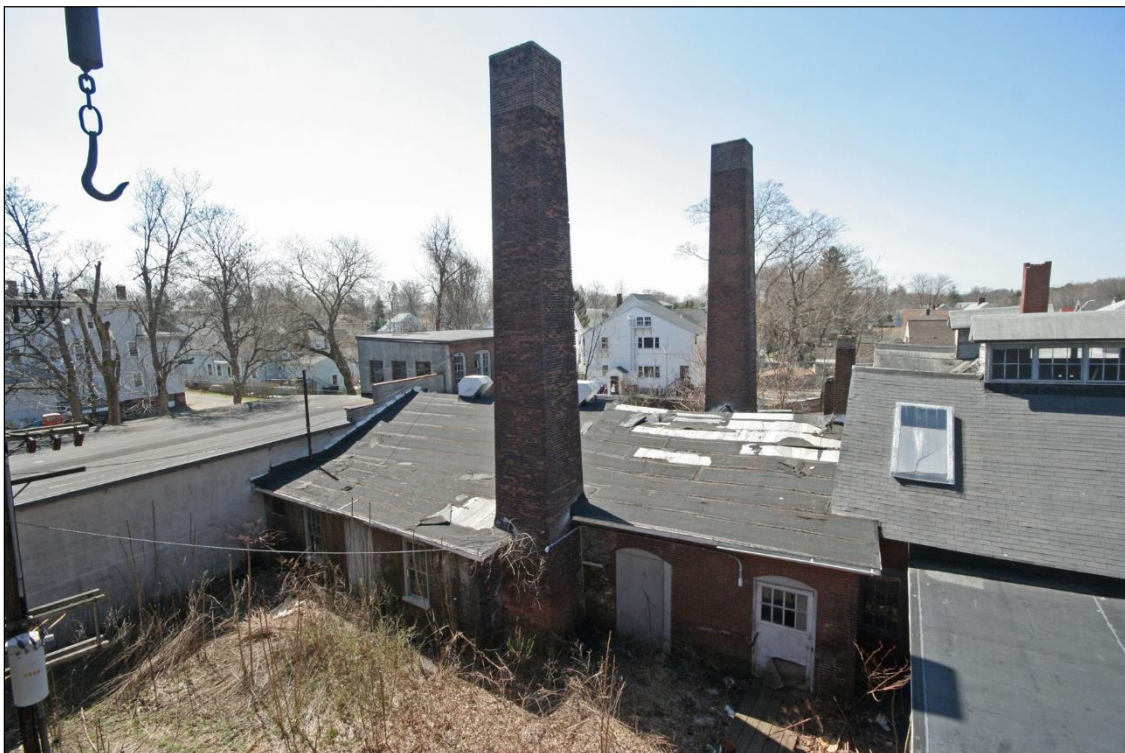
Photo No. 10: Engine House (c.1880) center, north elevation, attached to Shipping/Receiving & Machine Shop, left, and Paint Shop, right, from 3 rd floor of Factory. Looking S.
