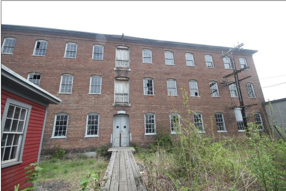
Photo No. 9: Factory, south elevation. Looking NE.
