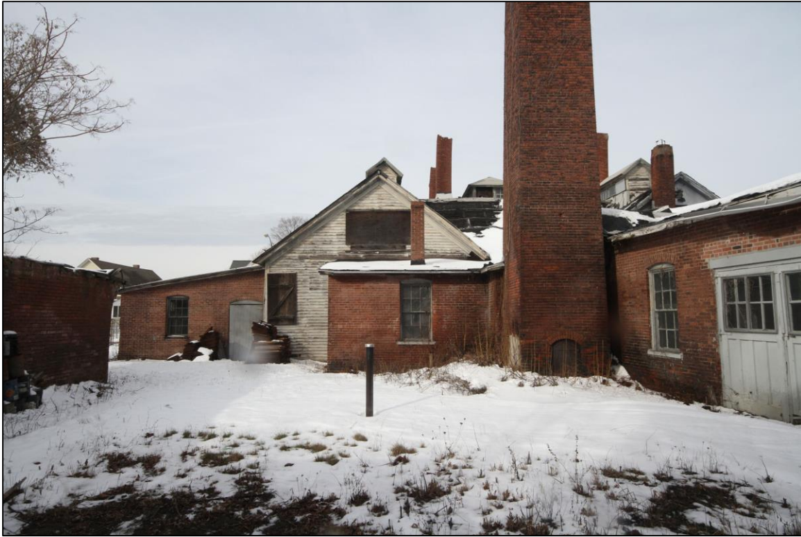
Photo No. 5: Paint Shop, rear elevation. Looking W.
