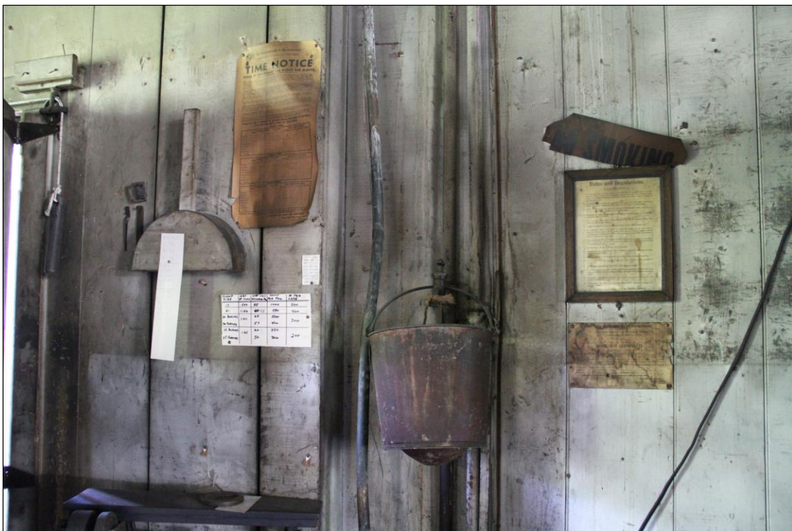
Photo No. 20: Factory, interior, Button Machine Shop, close-up detail of Photo 14, showing original rules, notices and water bucket fire extinguisher. Looking W.
