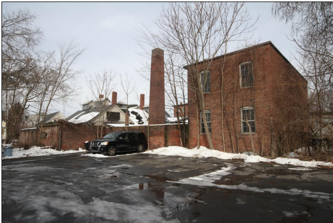
Photo No. 13: Nail Cutting and Polishing Shop (1893) at right; Sawdust House, center, Storehouse, left. South elevations viewed from adjacent property. Looking N.
