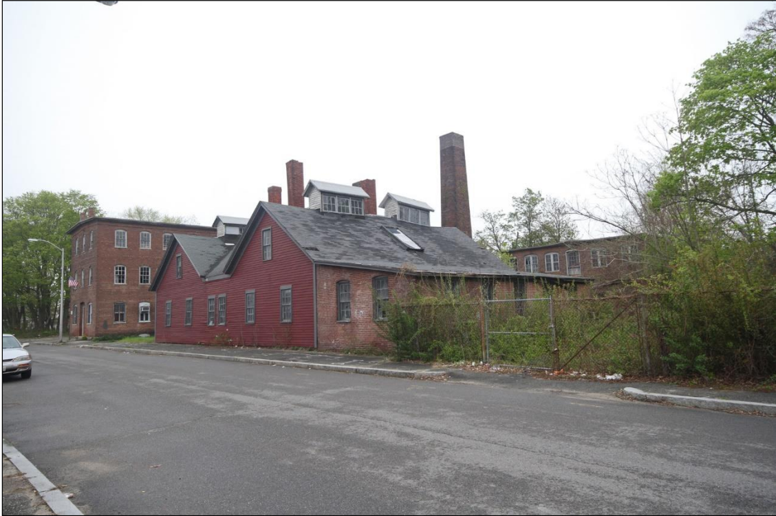
Photo No. 1: Entire complex view fronting Porter Street (west elevations), showing Paint Shop (c.1850) center and Factory (1880) at left in distance. Looking NE.
