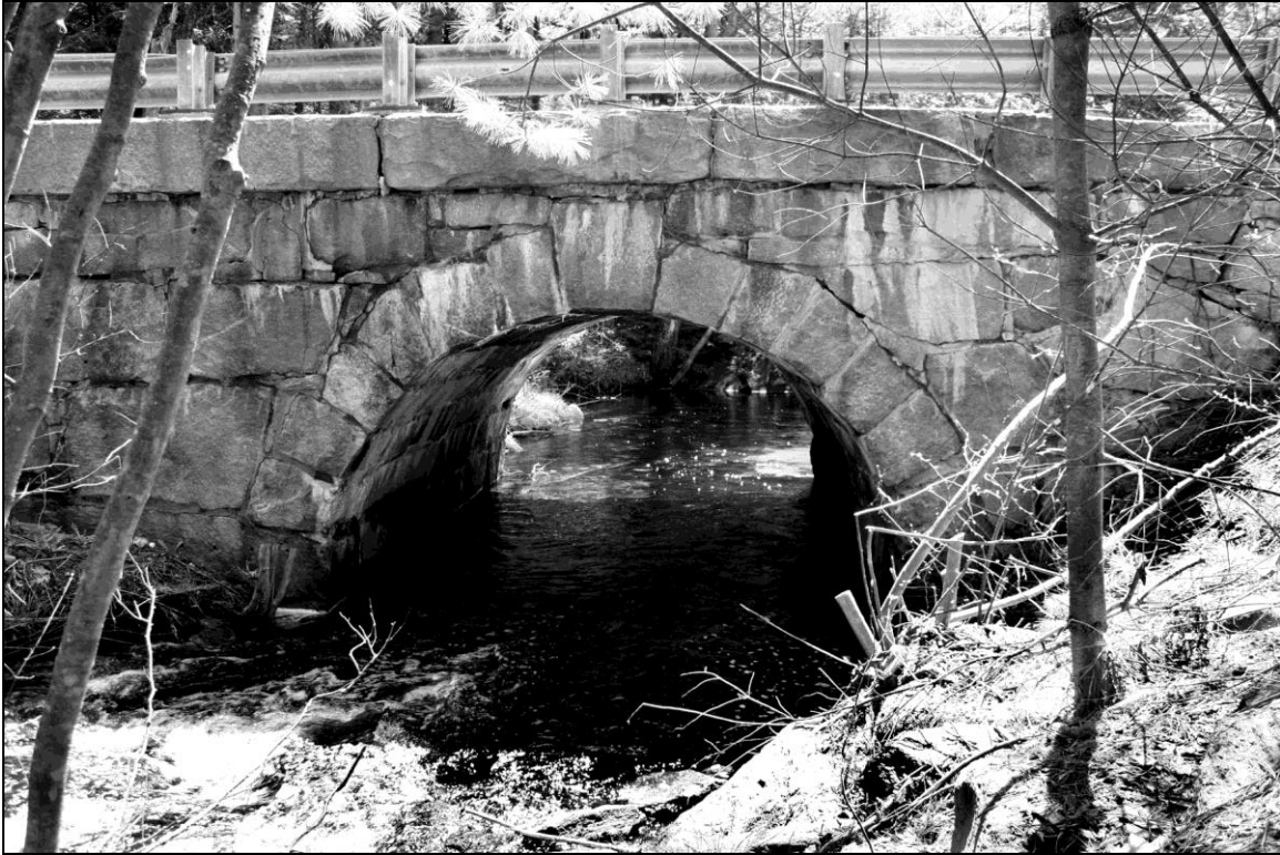
Photo No. 9: Culvert JAF0464 (Jaffrey)
