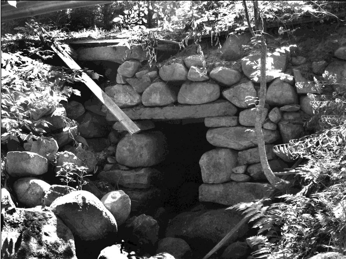
Photo No. 7: Culvert WOL0026 (Wolfeboro)
