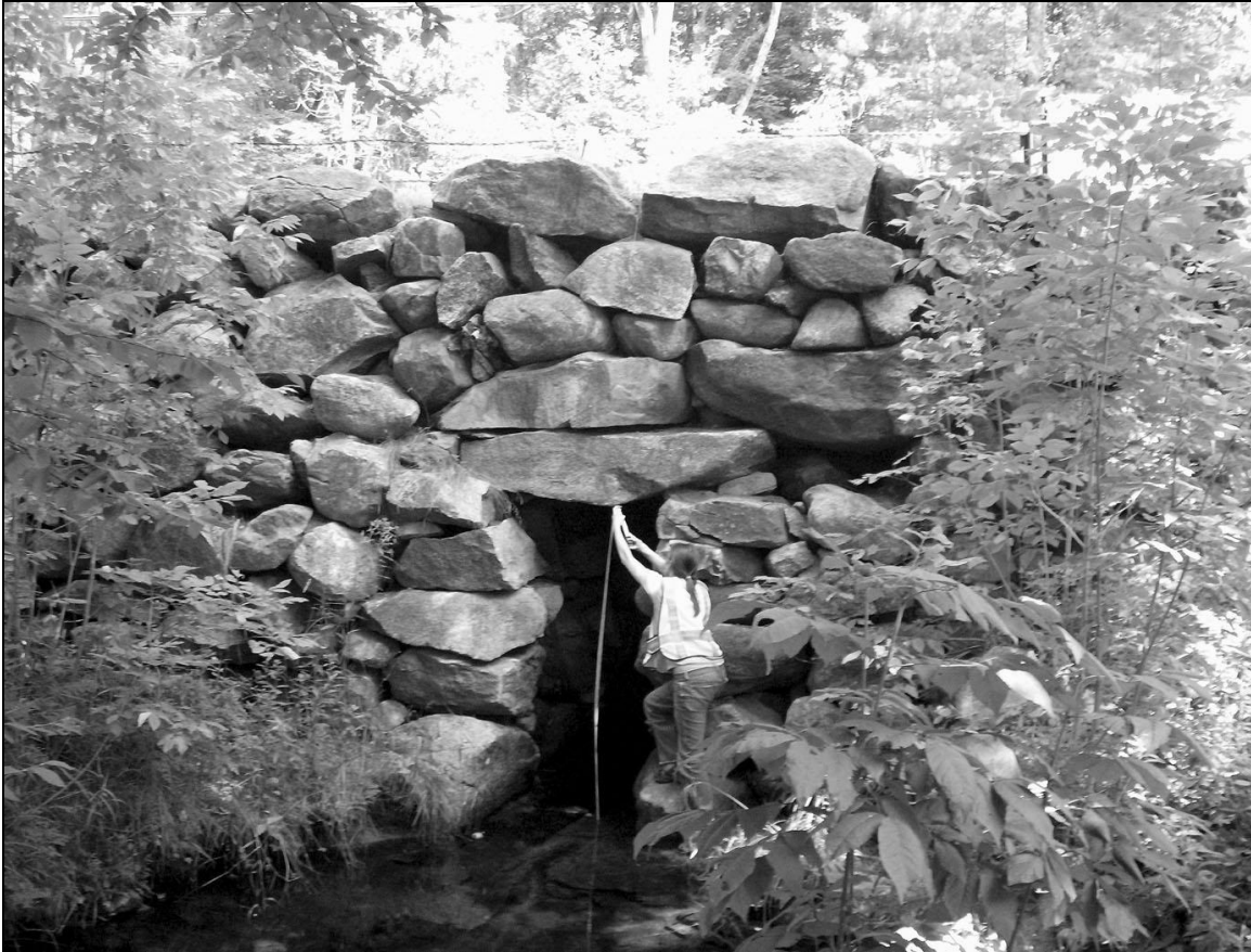
Photo No. 3: Culvert TUF0007 (Tuftonboro)
