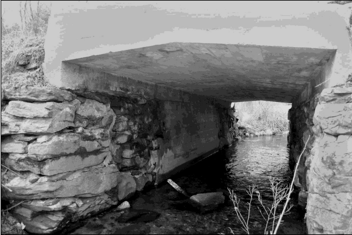
Photo No. 22: Culvert LON0112 (Londonderry)
