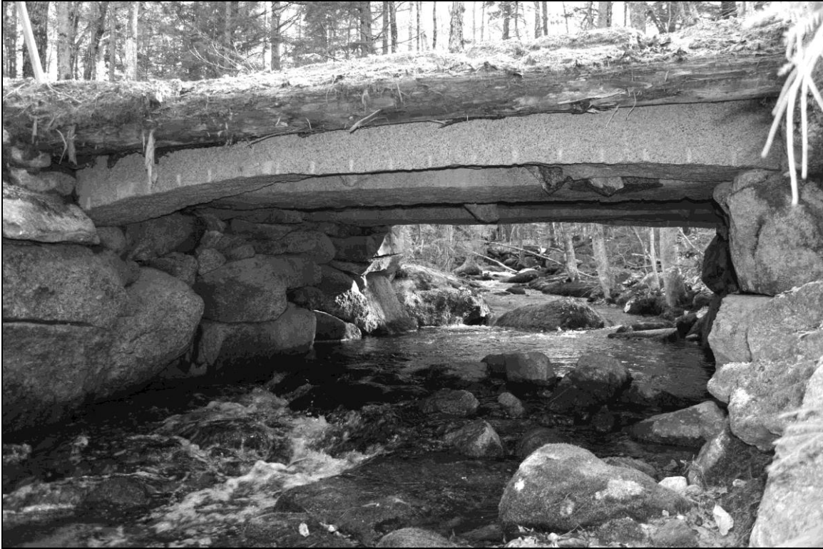
Photo No. 1: Culvert HIL0019 (Hillsborough)
