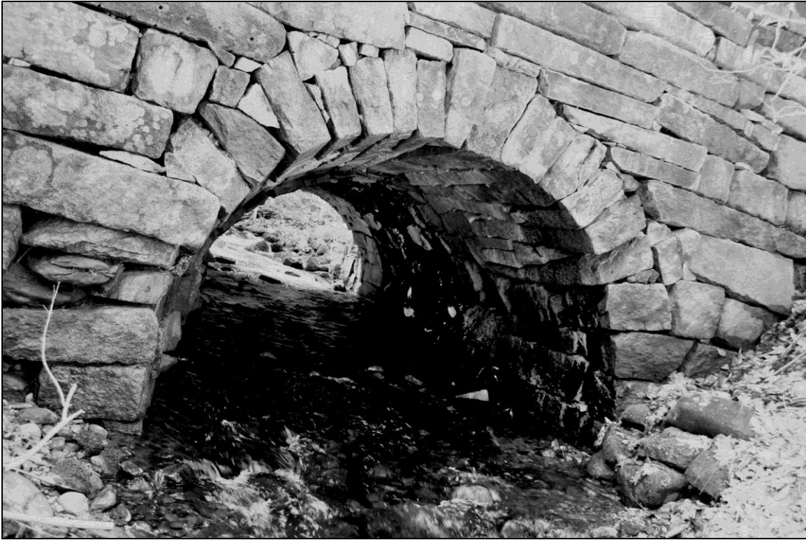
Photo No. 12: Culvert WIL0006 (Wilton)
