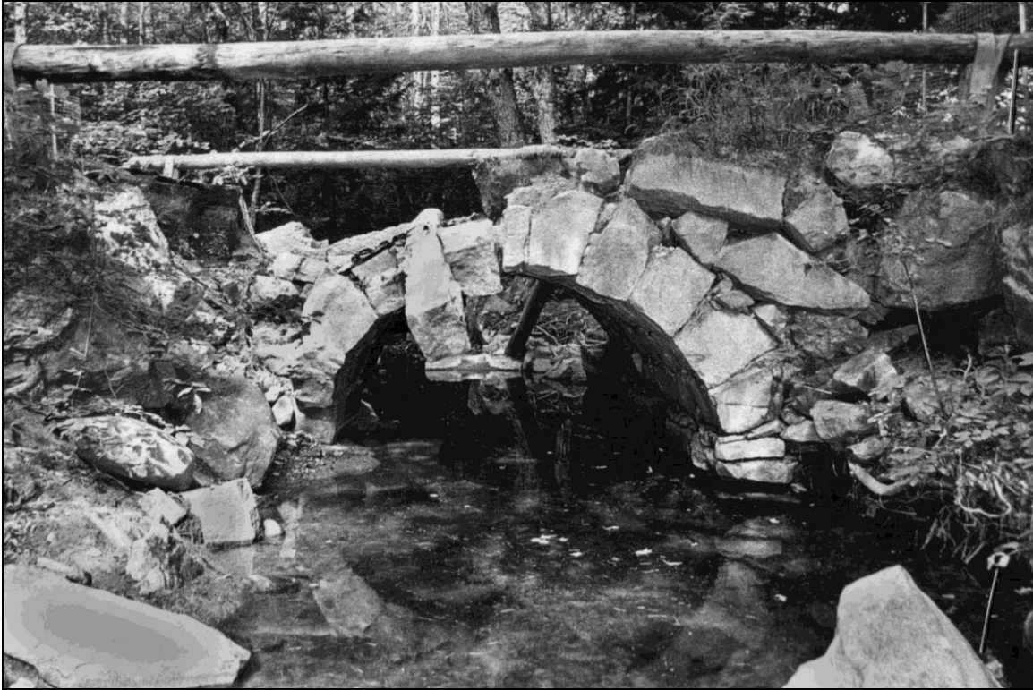
Photo No. 15: Culvert TEM0002 (Temple)
