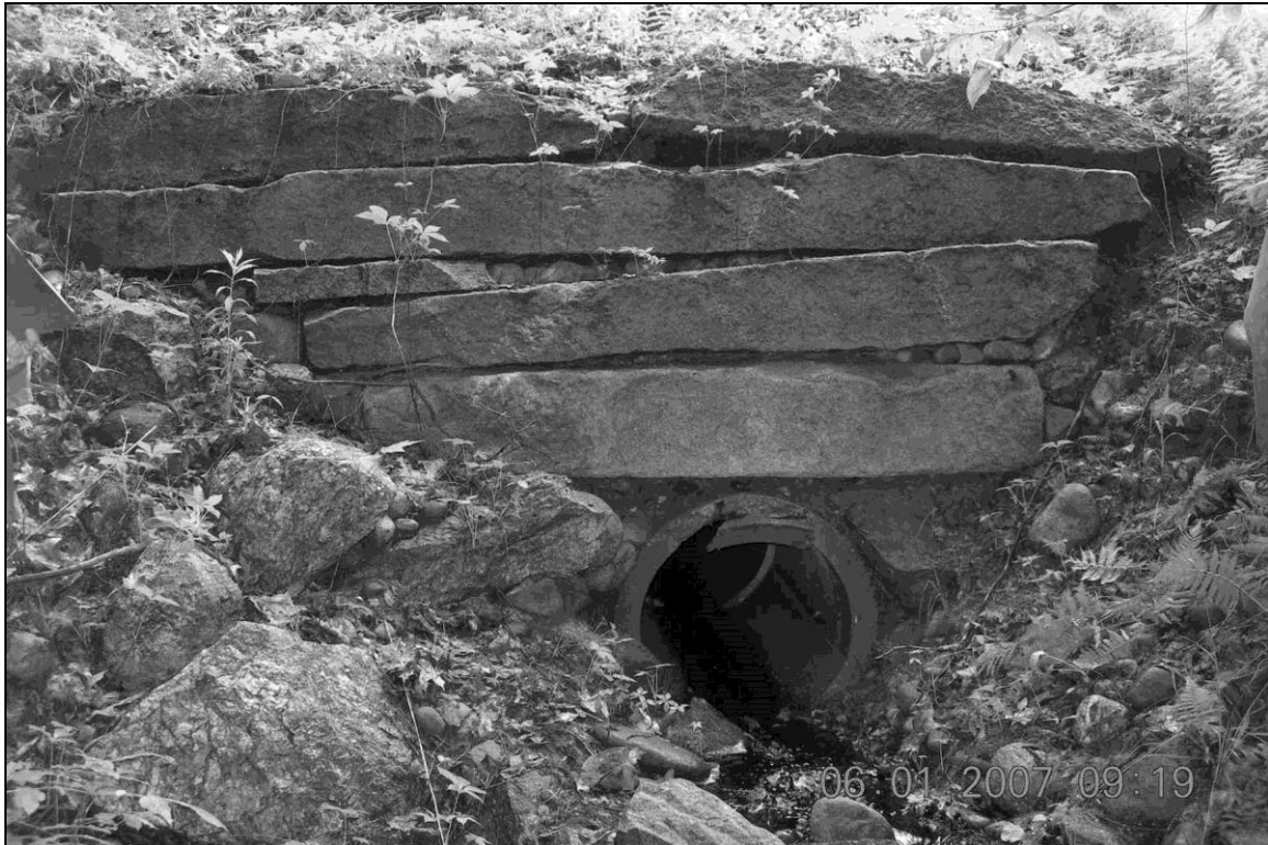
Photo No. 18: Culvert PEM0040 (Pembroke)
