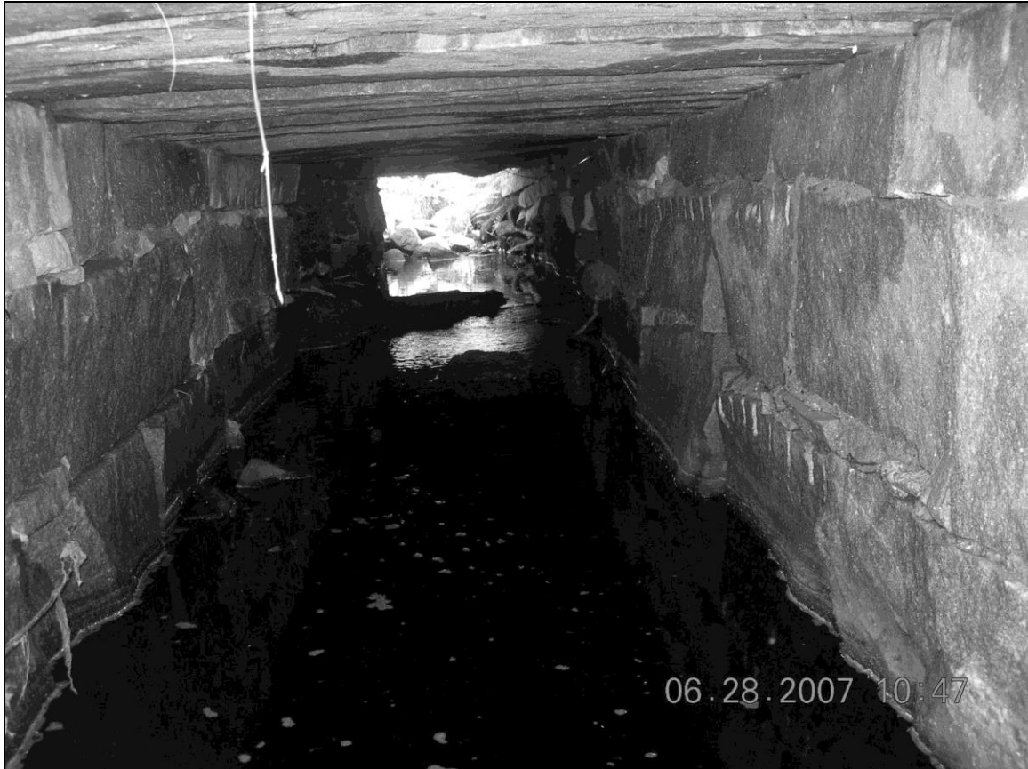
Photo No. 23: Culvert FIT0015 (Fitzwilliam)
