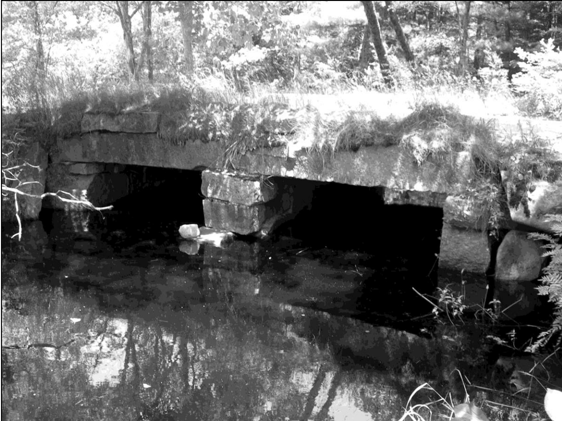
Photo No. 4: Culvert FIT0017 (Fitzwilliam)
