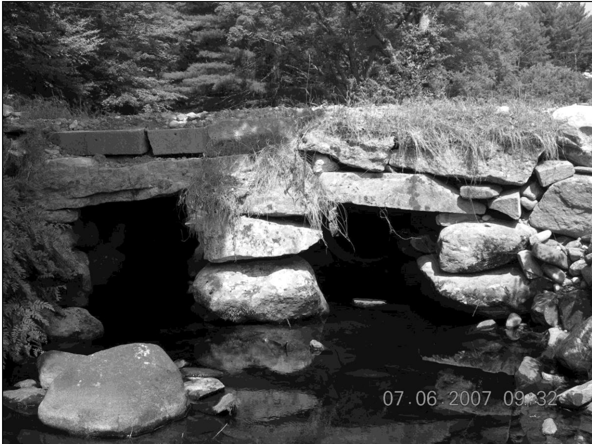
Photo No. 5: Culvert CNT0007 (Canterbury)
