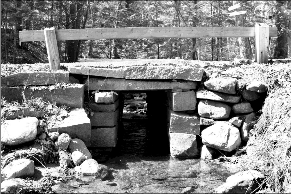
Photo No. 8: Culvert MAR0015 (Marlborough)
