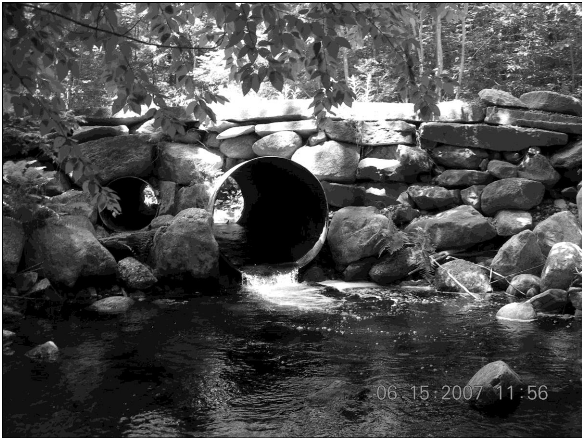
Photo No. 17: Culvert SWA0019 (Swanzy)
