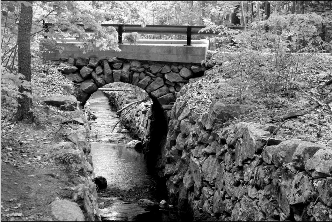
Photo No. 21: Culvert WAK0010 (Wakefield)
