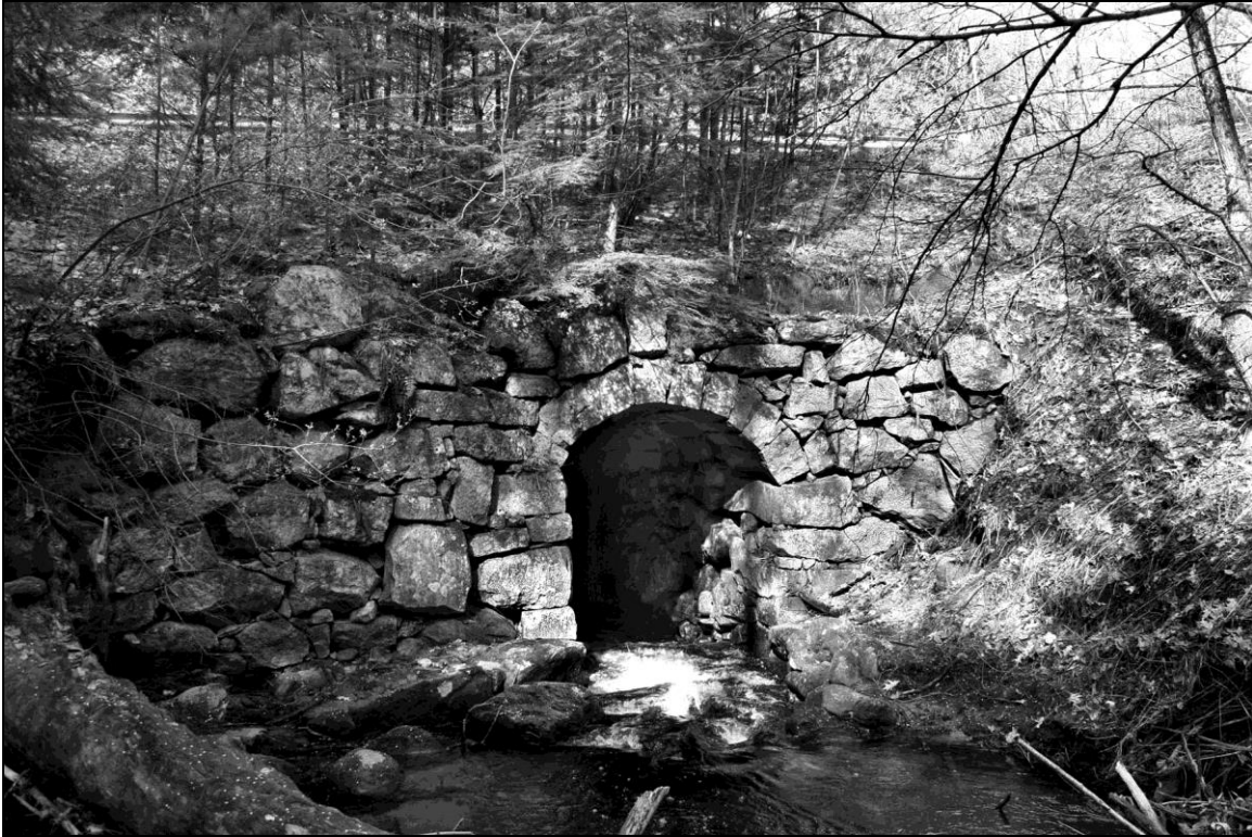
Photo No. 10: Culvert LIT0010 (Litchfield)
