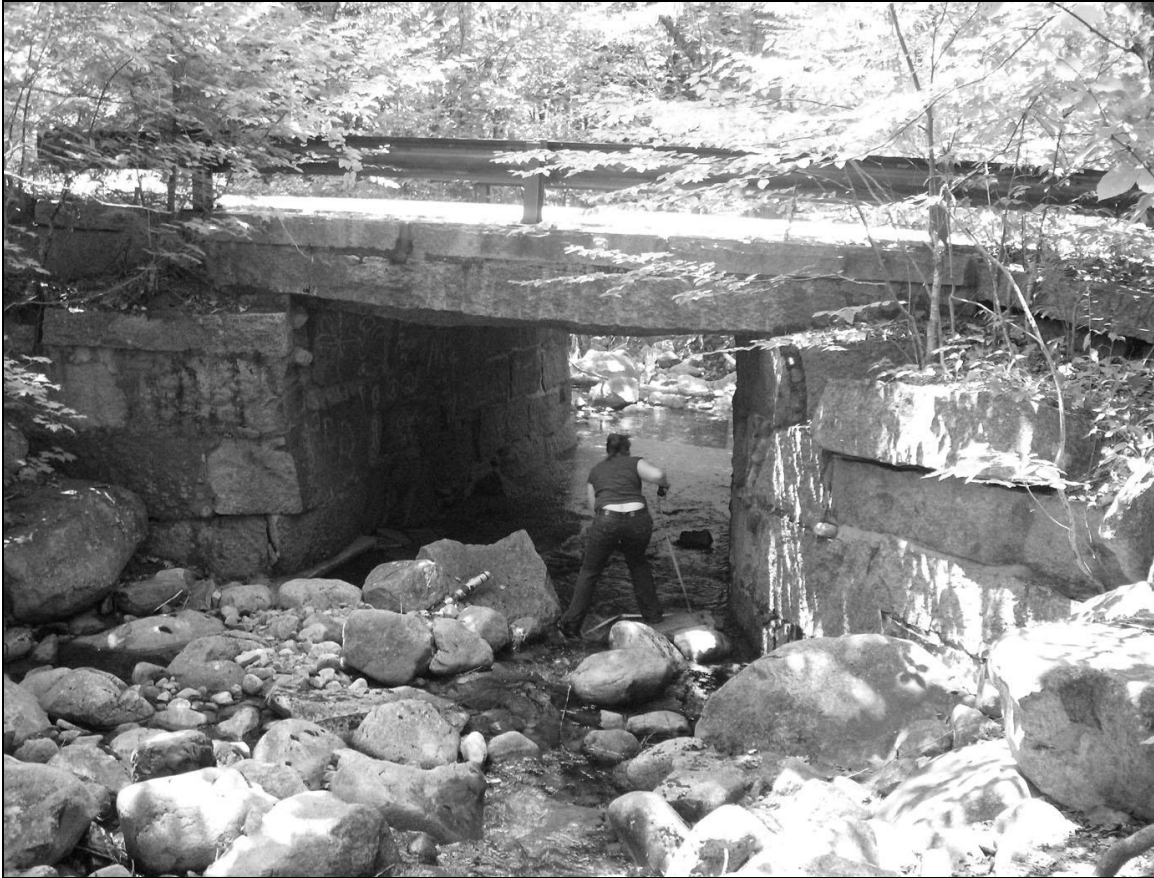
Photo No. 2: Culvert ALB0045 (Albany)
