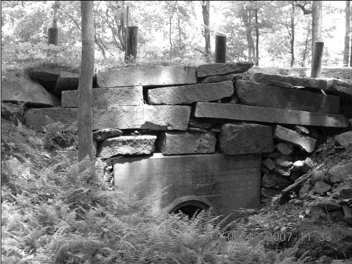
Photo No. 20: Culvert TRO0344 (Troy)
