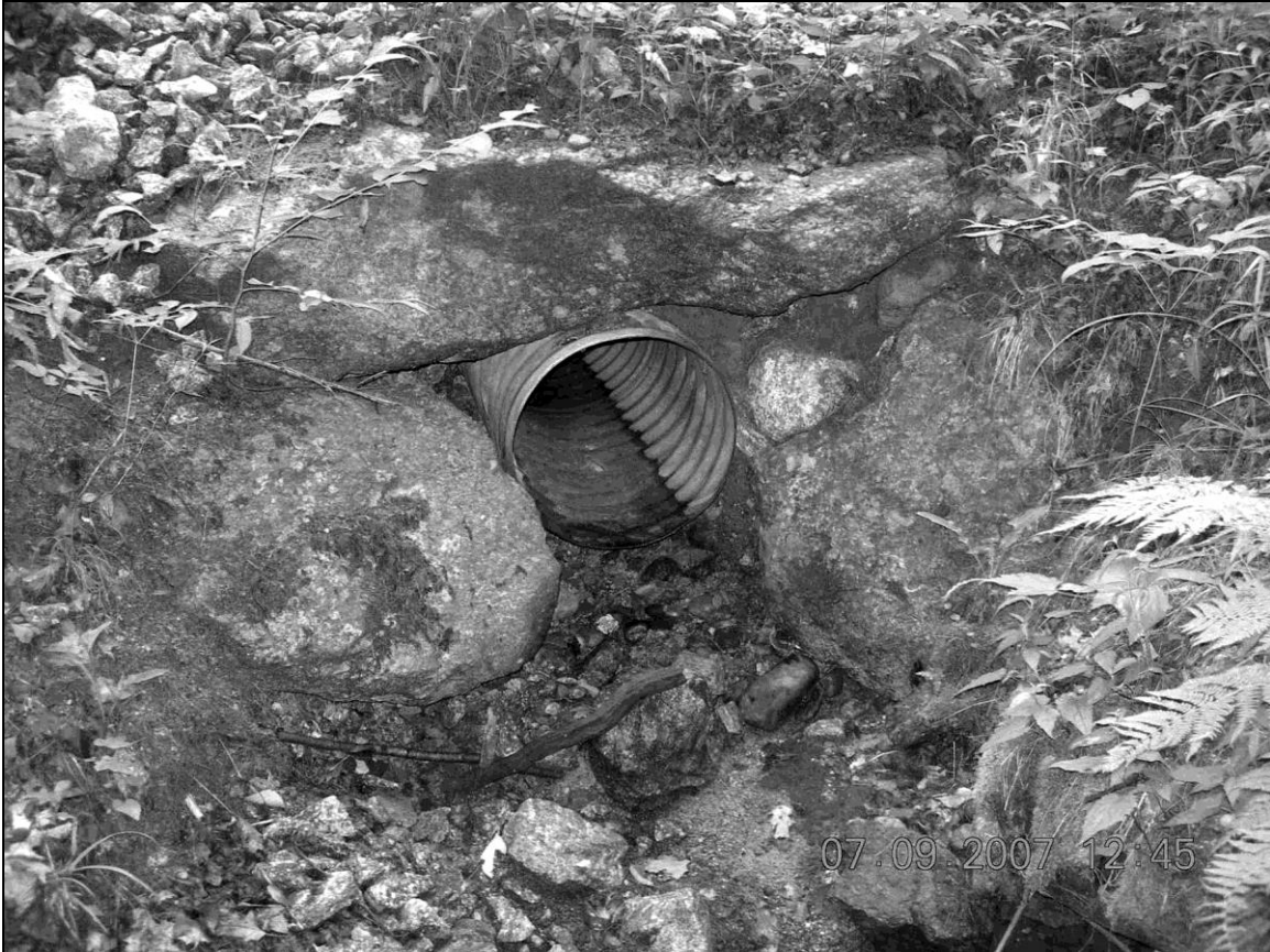
Photo No. 19: Culvert NBR0004 (Newbury)
