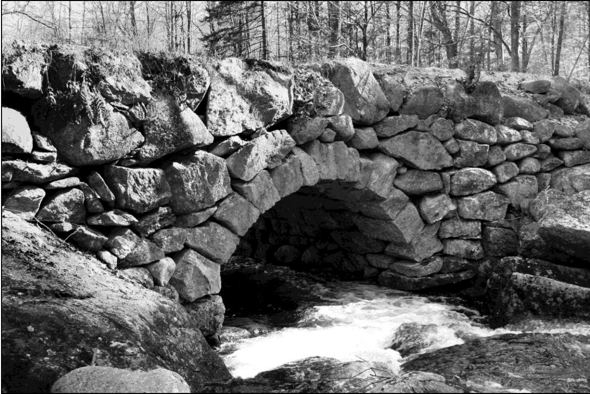
Photo No. 11: Culvert HIL0022 (Hillsborough)
