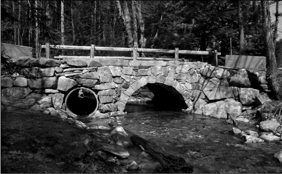
Photo No. 24: Culvert TEM0002 (Temple)
