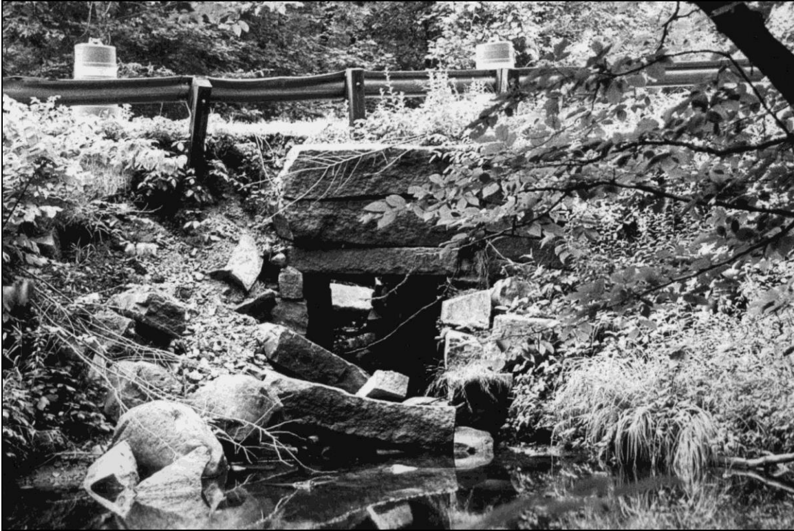
Photo No. 14: Culvert HIL0144 (Hillsborough)
