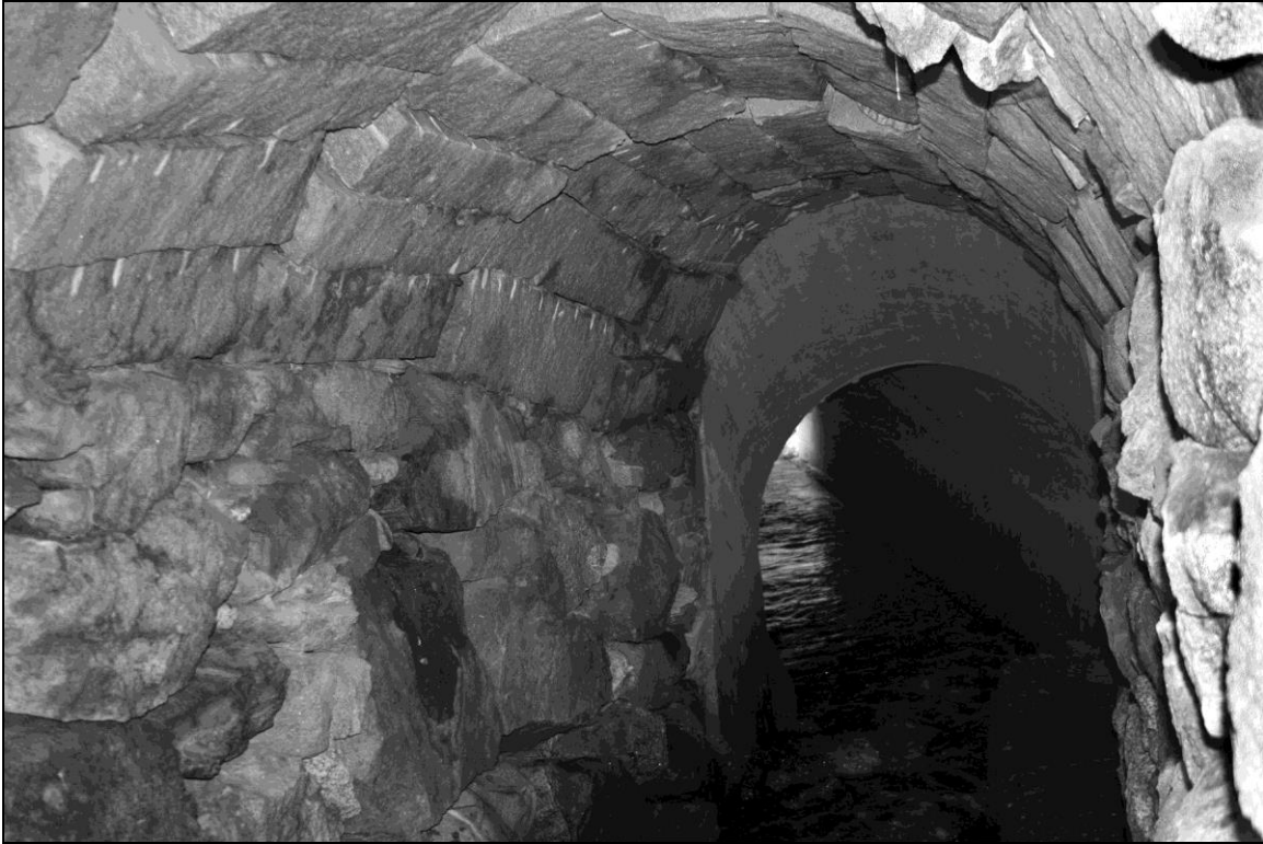
Photo No. 16: Culvert LIT0010 (Litchfield)
