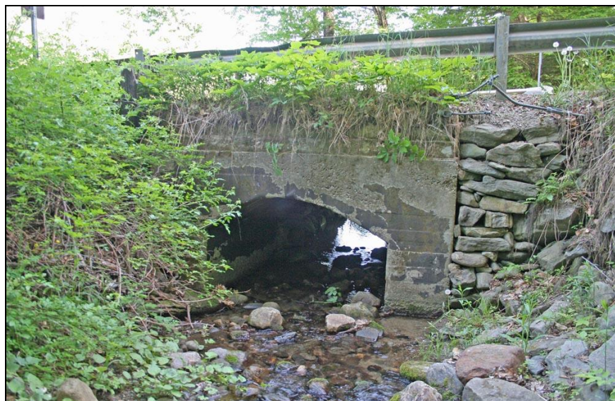
FIGURE 16: Hill Road, Brookline (WI-BRO-001). This is the upstream end of the one arch culvert surveyed in Vermont (see Figure 13) showing the lengthening of the culvert with cast-in-place concrete.
