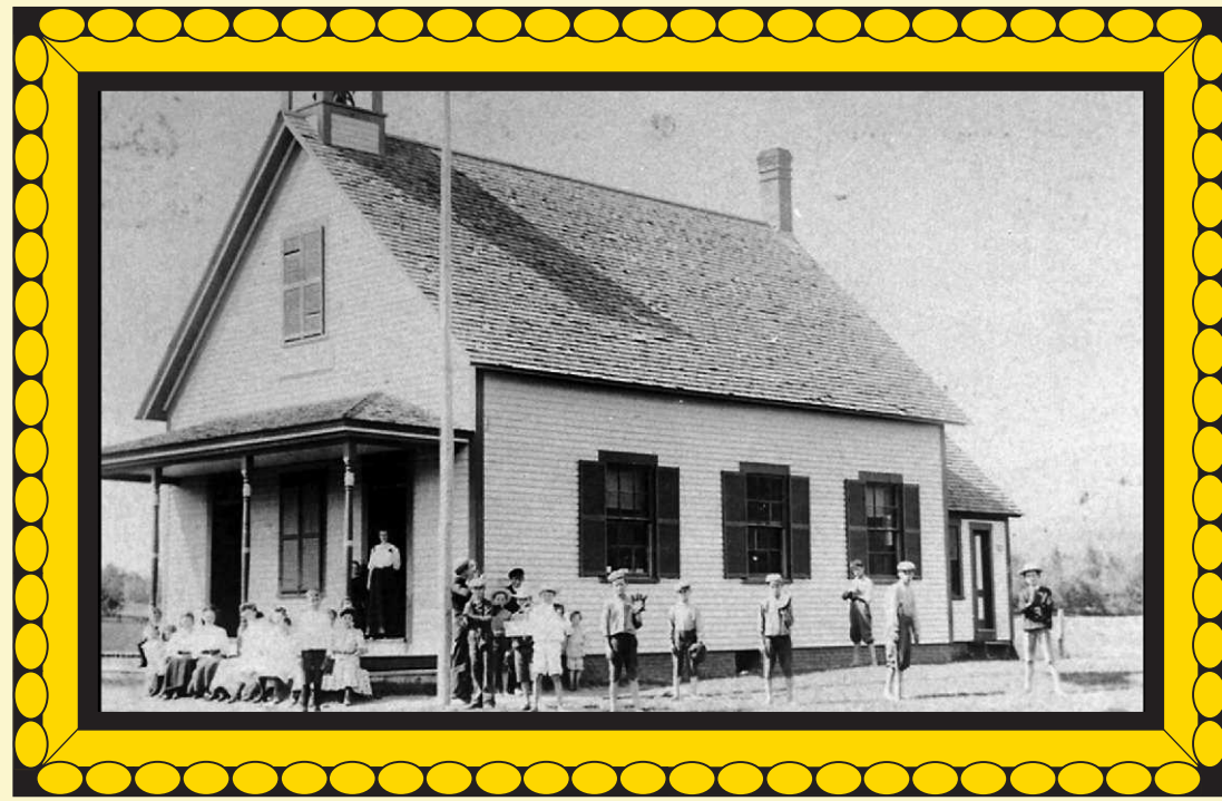
Montview School 3628 Route 25 - West Rumney
