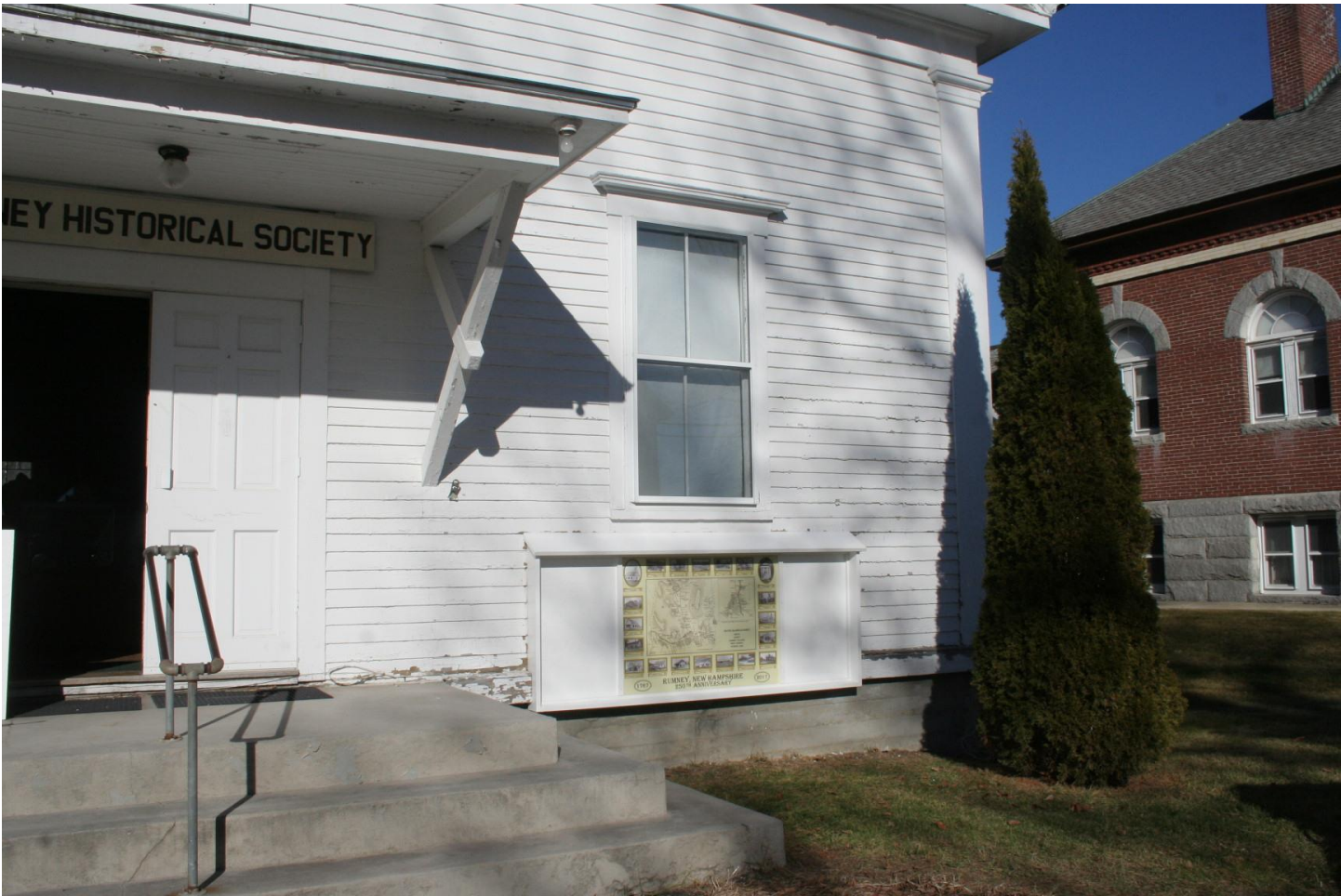
Rumney, New Hampshire. Sign Installed on Message Board on front of Rumney Historical Society Building
