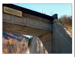
This concrete deck slab bridge (above) was built in 1937 by the Canadian National Railway to carry the line over Route 110 in Northumberland. The grade separation project was noted in the engineering press at the time as an uncommonly heavy pre-cast slab bridge, consisting of two 108-ton slabs set in place by two 150-ton locomotive cranes. Dismantling the old bridge and completing the new one was done in 4-1/2 hours without interruption of scheduled train service.
