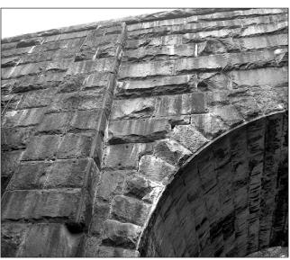
The ashlar granite stonework along the line is of exceptional quality, as shown by this 19th century stone arch bridge over the North Branch of the Ammonoosuc River a short distance north of the former Copperville station in Milan. The impressive arch is 20' wide, 50' high with stone abutments extending about 100' to each side.
