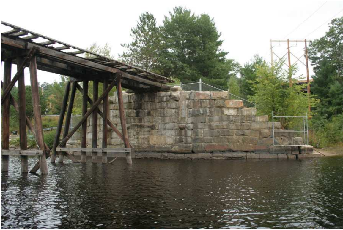
Photo # 6 description: South side of Manchester abutment.
