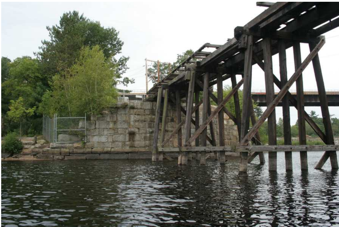
Photo # 7 description: Pile bents and north side of Manchester abutment.
