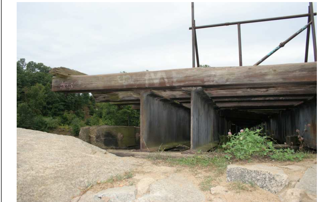
Photo # 11 description: Detail of double steel I-beam stringers supporting wood ties.
