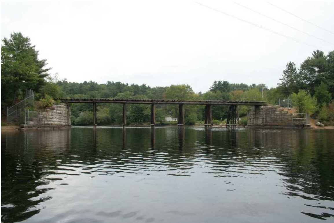
Photo # 3 description: Overall view of south (downstream side of bridge).
