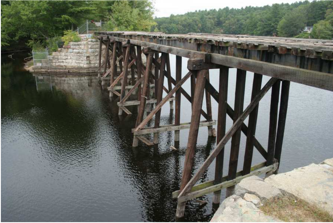
Photo # 8 description: Oblique view of pile bents .
