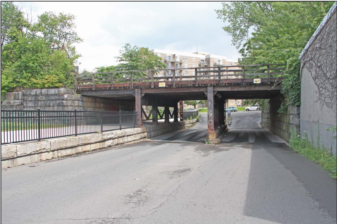
Photo No. 4: West elevation and approach from Main St. Looking E.
