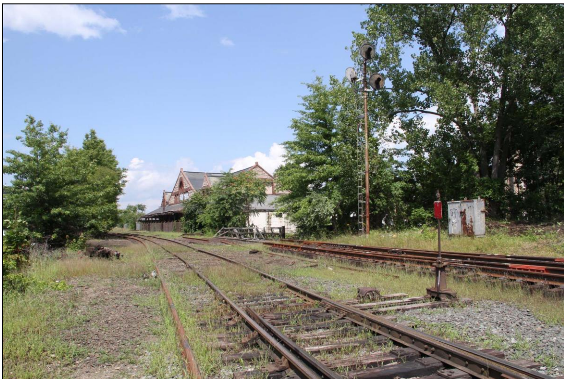
Photo No. 8: Bridge deck, showing rail approach from south and former railroad station in background. Looking N.
