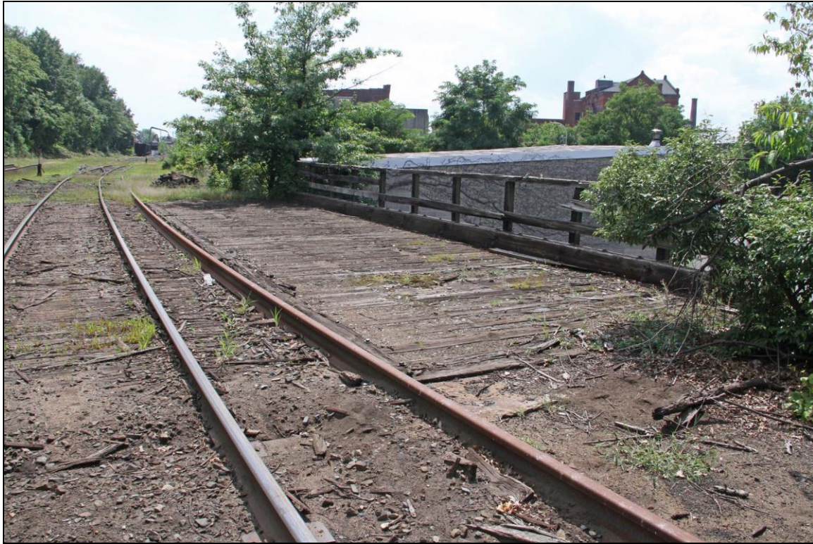
Photo No. 7: Bridge deck, showing solid wood tie construction. Looking SW.
