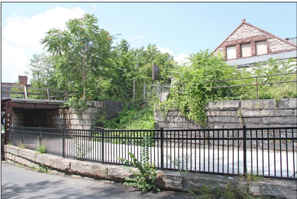
Photo No. 2: Sidewalk, retaining wall, and stone stairs to Train Station, visible at right. Looking N.
