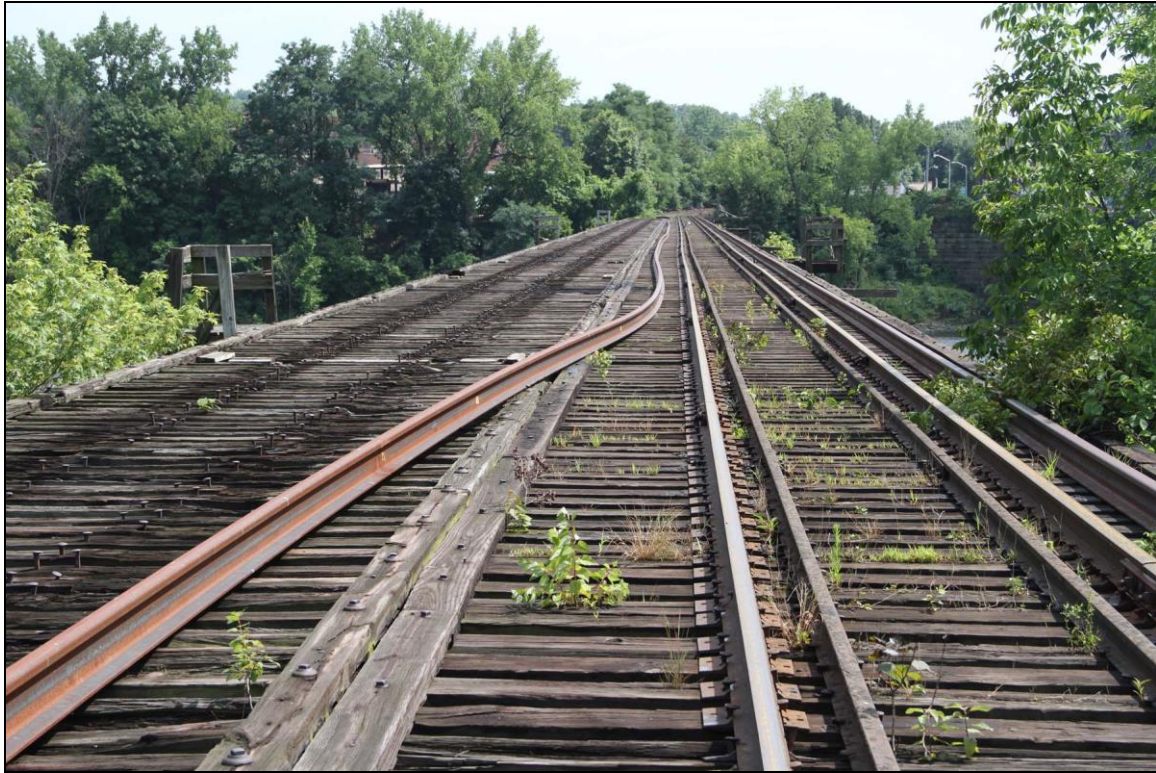
Photo No. 7: Detail of bridge deck, looking SE.
