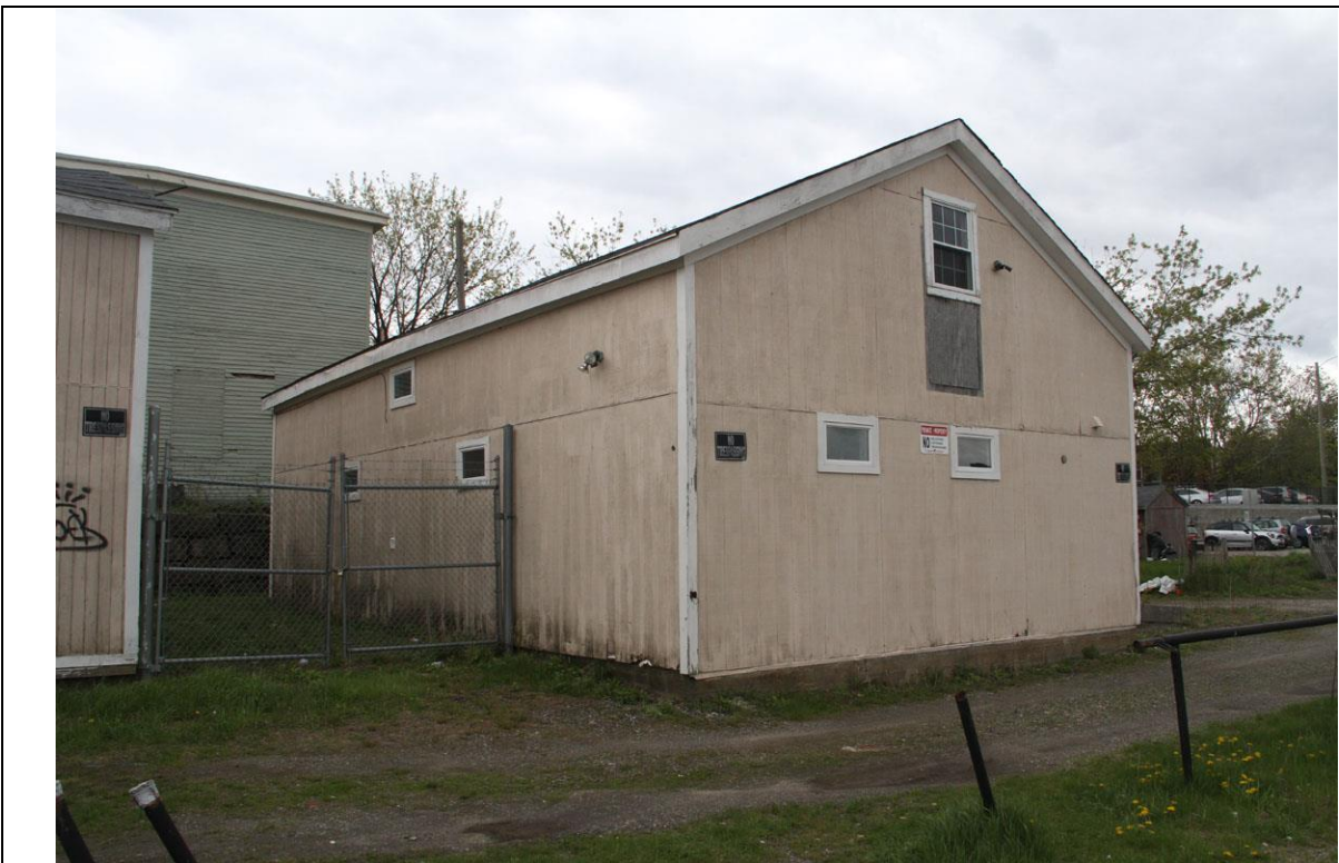
Photo #: 24 Description: Building B, Portsmouth Foundry Co., c.1915
