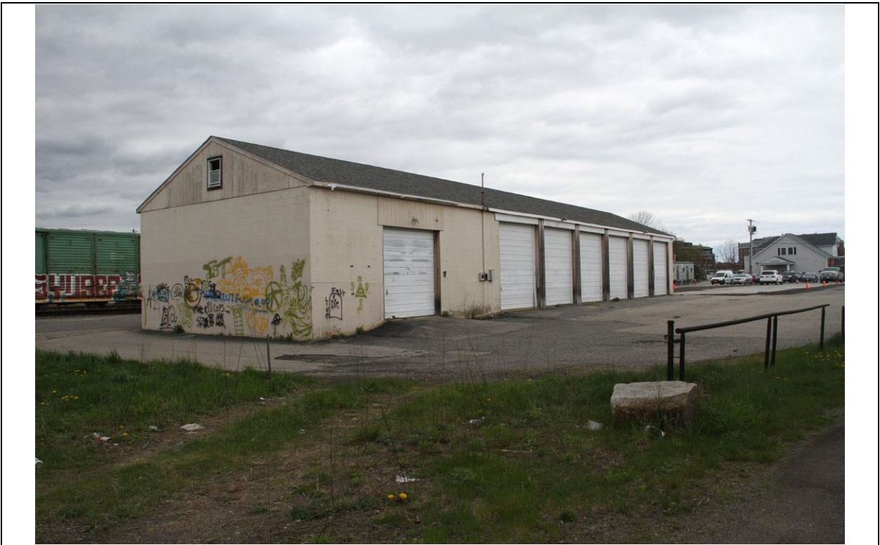
Photo #: 27 Description: Building D, Storehouse, 1990, SW & SE sides. Reference (file name): PDSE_027 Direction: N Date taken: 5/9/2017 Negative stored: n/a
