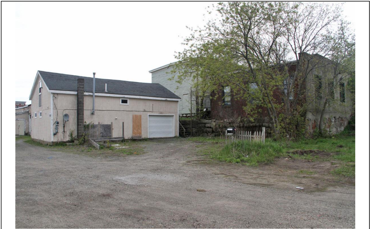
Photo #: 11 Description: Building B, Portsmouth Foundry Co., c.1915, at left. Rear of brick Industrial Building, c.1870 (HD#426) abutting PA, at right. Reference (file name): PDSE_011 Direction: E Date taken: 5/9/2017 Negative stored: n/a
