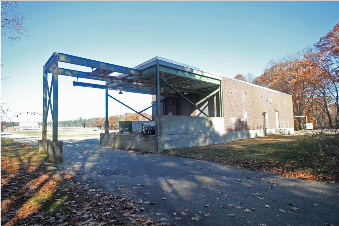
Photo :# 19 Description: Chlorinator Building, south side, showing chlorine loading dock on west end of building. Reference (file name or frame #): MER0168_019 Direction: NE
