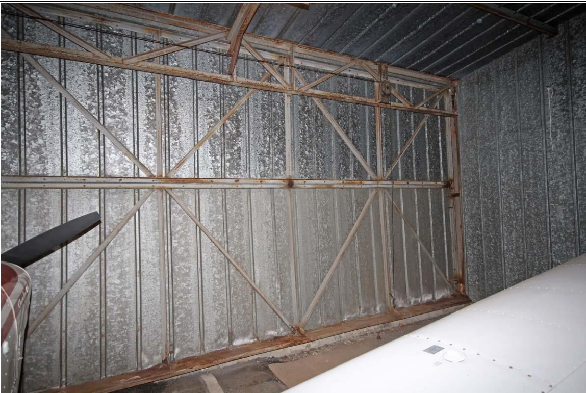
Photo # 7: Interior view of bi-fold canopy hangar door
