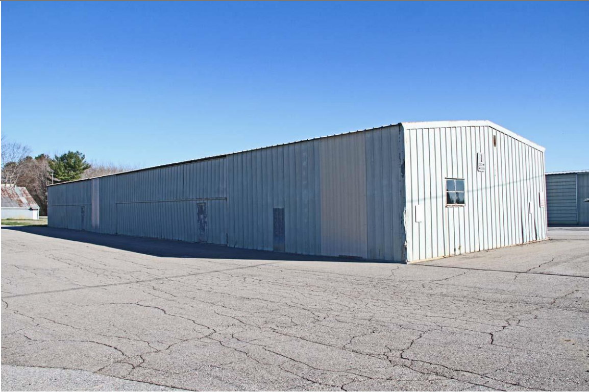
Photo # 2: Hangar 1, south and east elevations.
