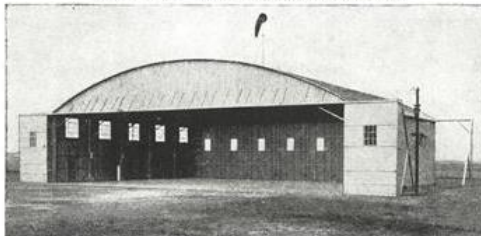
Fig. 464. Butler (All-Steel) Type RT-100 Hangar 100' wide x 70' long x 25' high. Conventional type regular Butler construction.
