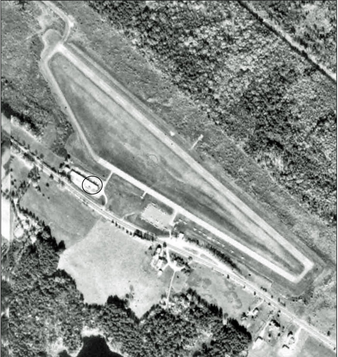
FIGURE 5: Aerial photograph, 1974. New runway built by state can be seen along with Hangar 1 (circled) with open pole-barn hangar added off its west end. Hangar 1/10 is also visible just west of pole barn (Source: Historic Aerials).
