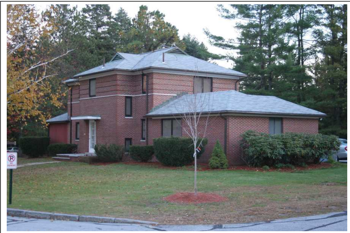
Photo #15: Bldg 2, Manager's Home (1948), front (NE elevation) and right side. Direction: S
