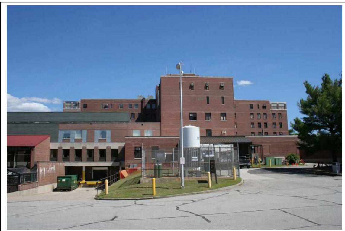
Photo #7: Bldg 1, rear, showing Bldg 15 attached at left. Direction: SE
