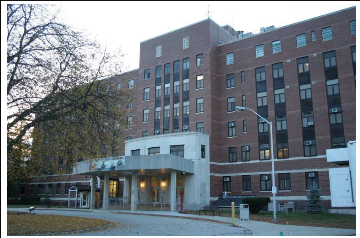
Photo #2: Bldg 1, Hospital, front, showing main entrance pavilion. Direction: W
