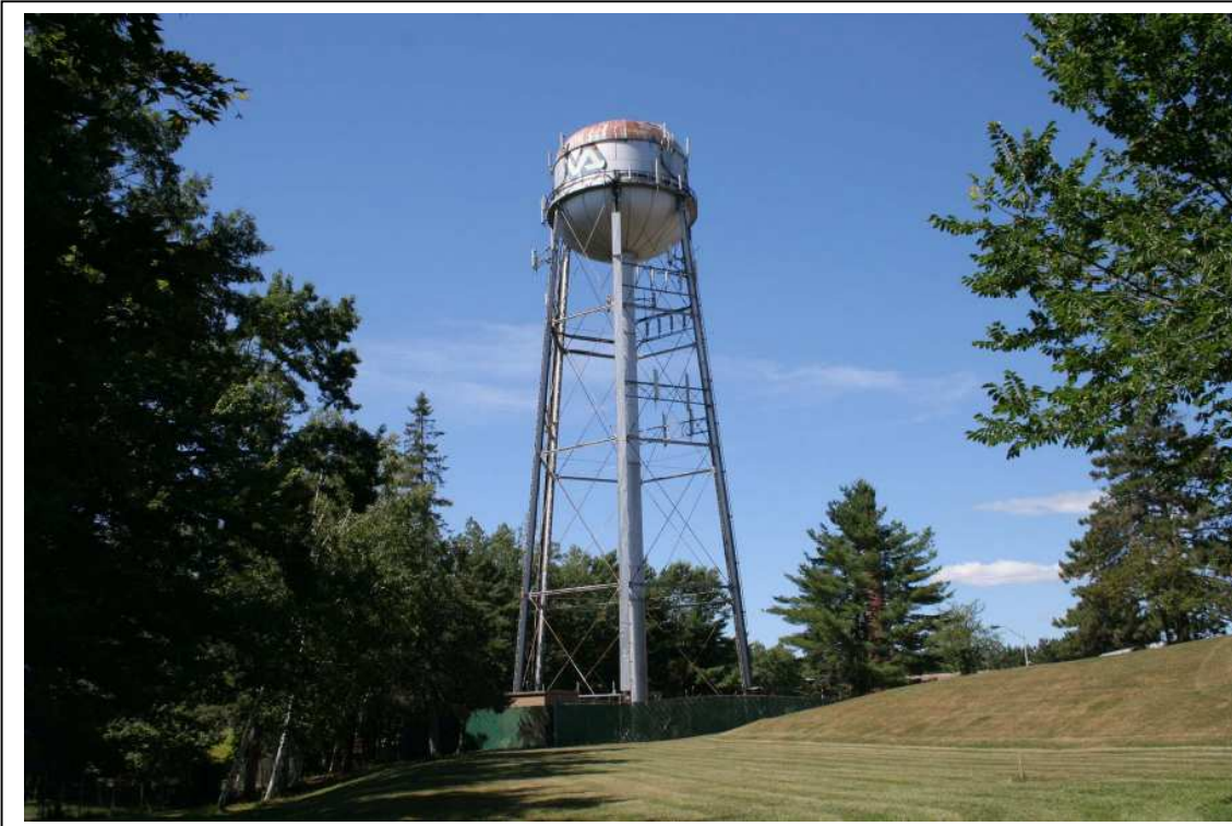
Photo #26: Water Tower (Bldg 9, 1948). Direction: N
