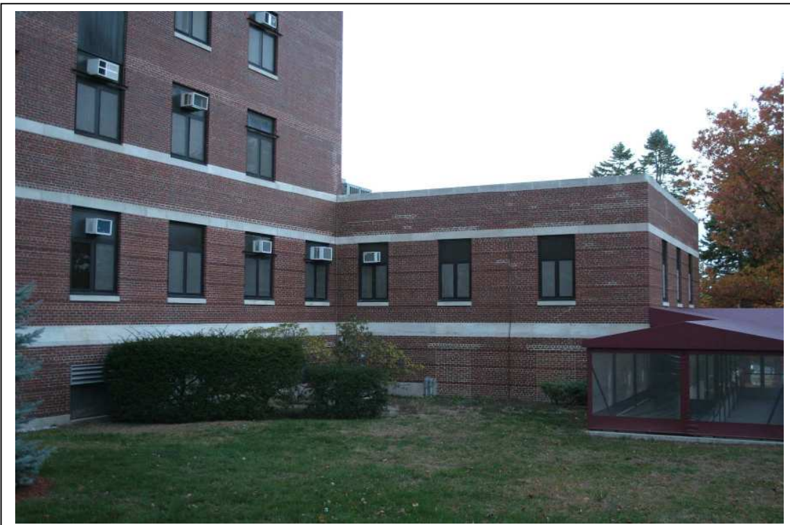
Photo #5: Bldg 1, right front corner, showing brick details and limestone belt coursing; brick infilled window openings on ground floor; new covered H/C access ramp on right. Direction: SW
