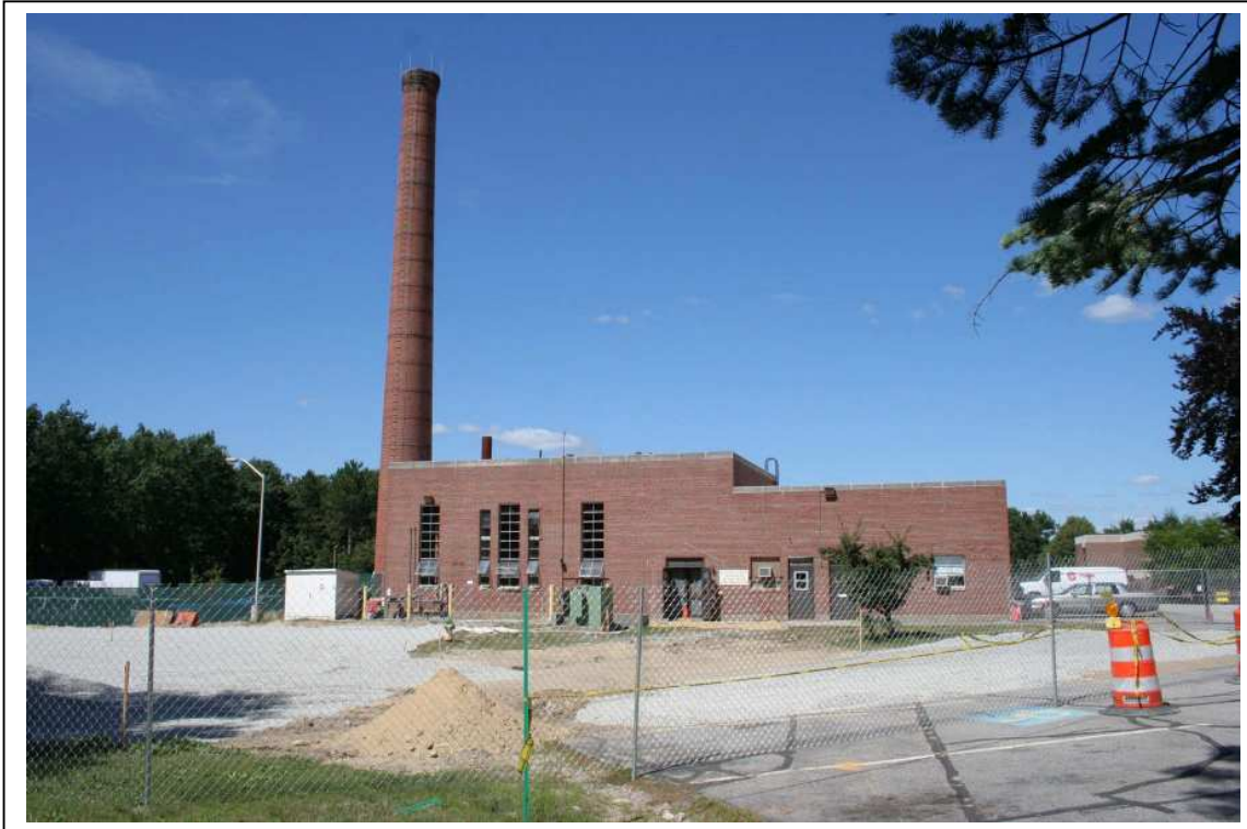
Photo #24: Boiler Plant & Garage (Bldg 7) southwest side elevation, also showing the chimney Stack (Bldg 20). Direction: NE
