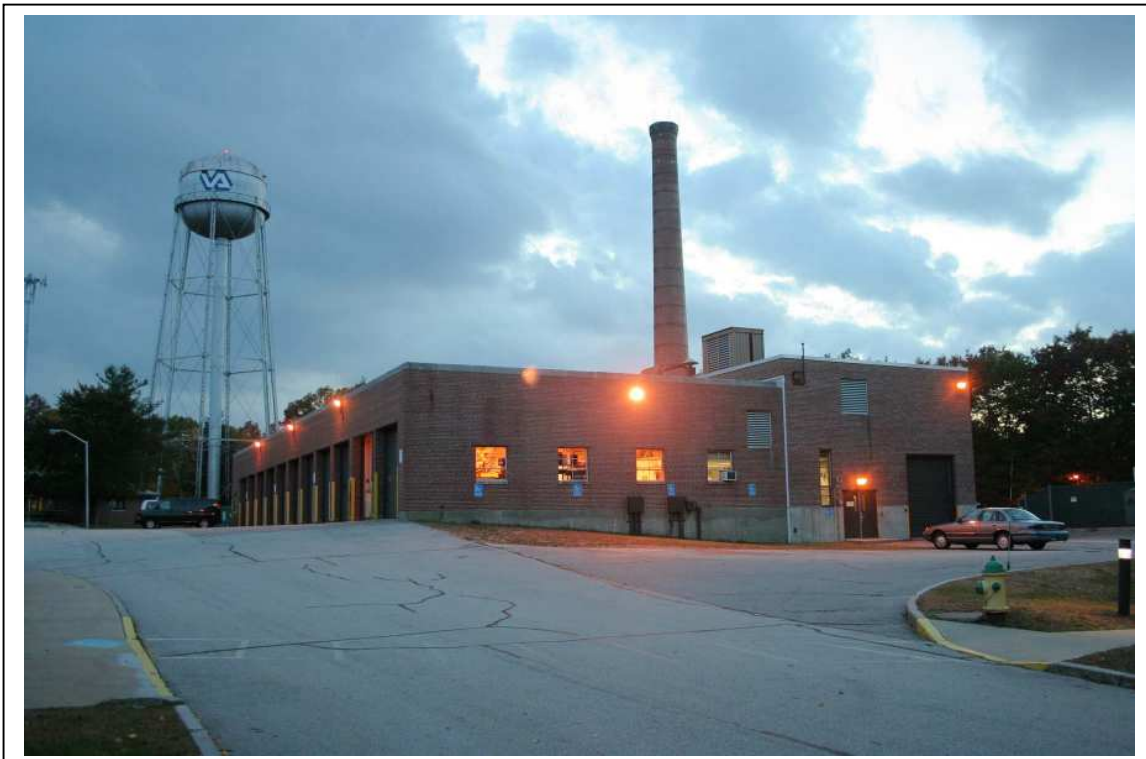
Photo #23: Boiler Plant & Garage (Bldg 7, 1948) southeast elevation with garage doors facing back of Hospital and northeast side facing camera. Direction: W
