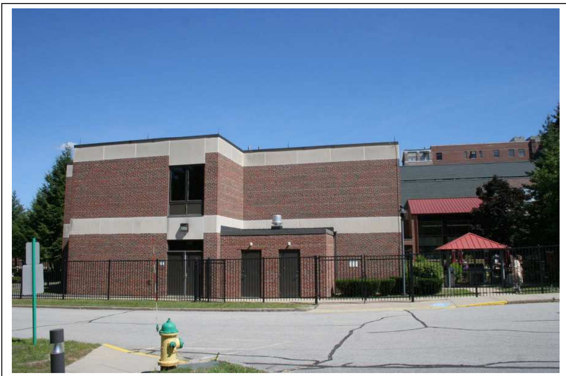
Photo #29: Bldg 15, Nursing Home Care Unit, rear; Bldg 1, rear, visible at upper right. Direction: SE
