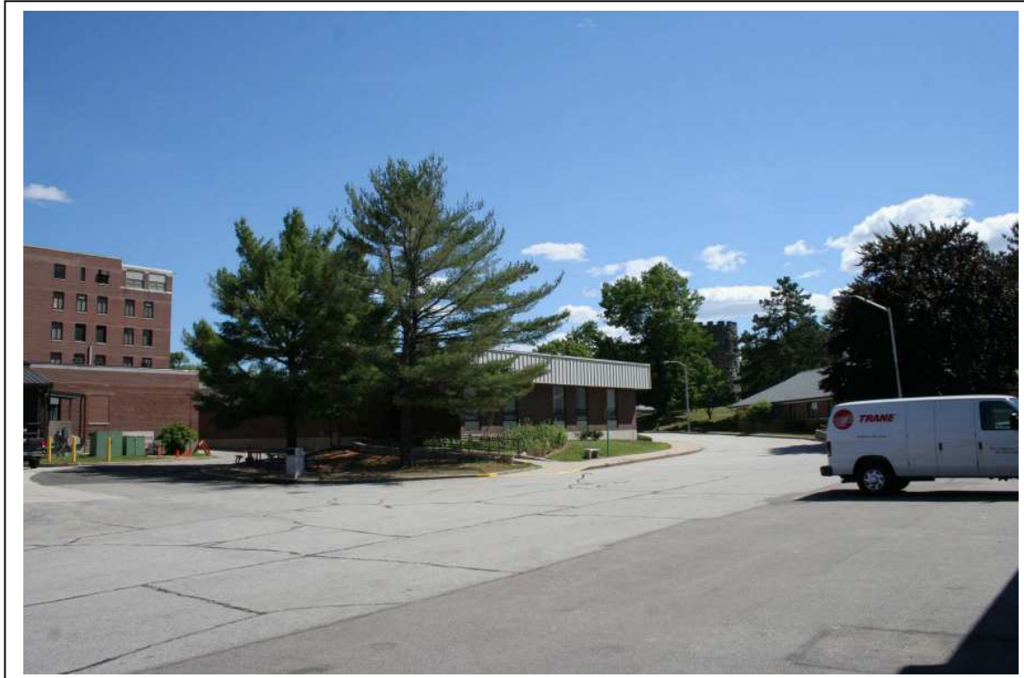
Photo #8: General view of rear driveway, showing rear of Bldg 1 at left, rear corner of Bldg 18, Primary Care Unit (built 1973) at center, and roof of Bldg 6 (1948) visible behind van. Direction: S
