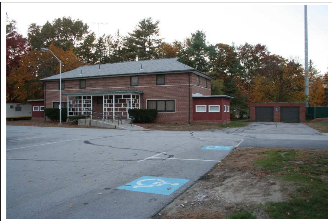
Photo #17: Bldg 4, Staff Quarters (1948), front (SE elevation) and right side, showing Garage (Bldg 14) at right. Direction: NW
