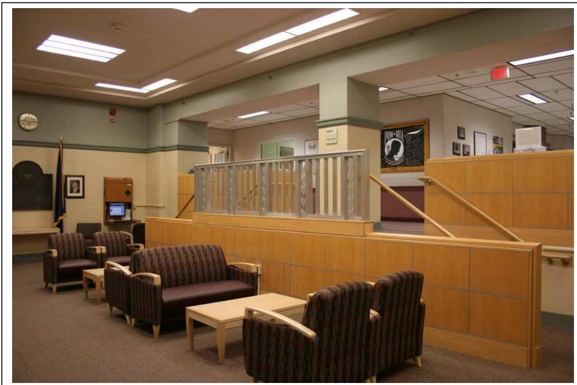
Photo #13: Bldg 1, interior, front lobby, showing original finish including concrete walls and columns, aluminum balustrade, veneer plywood with inlaid aluminum trim paneling. Direction: W
