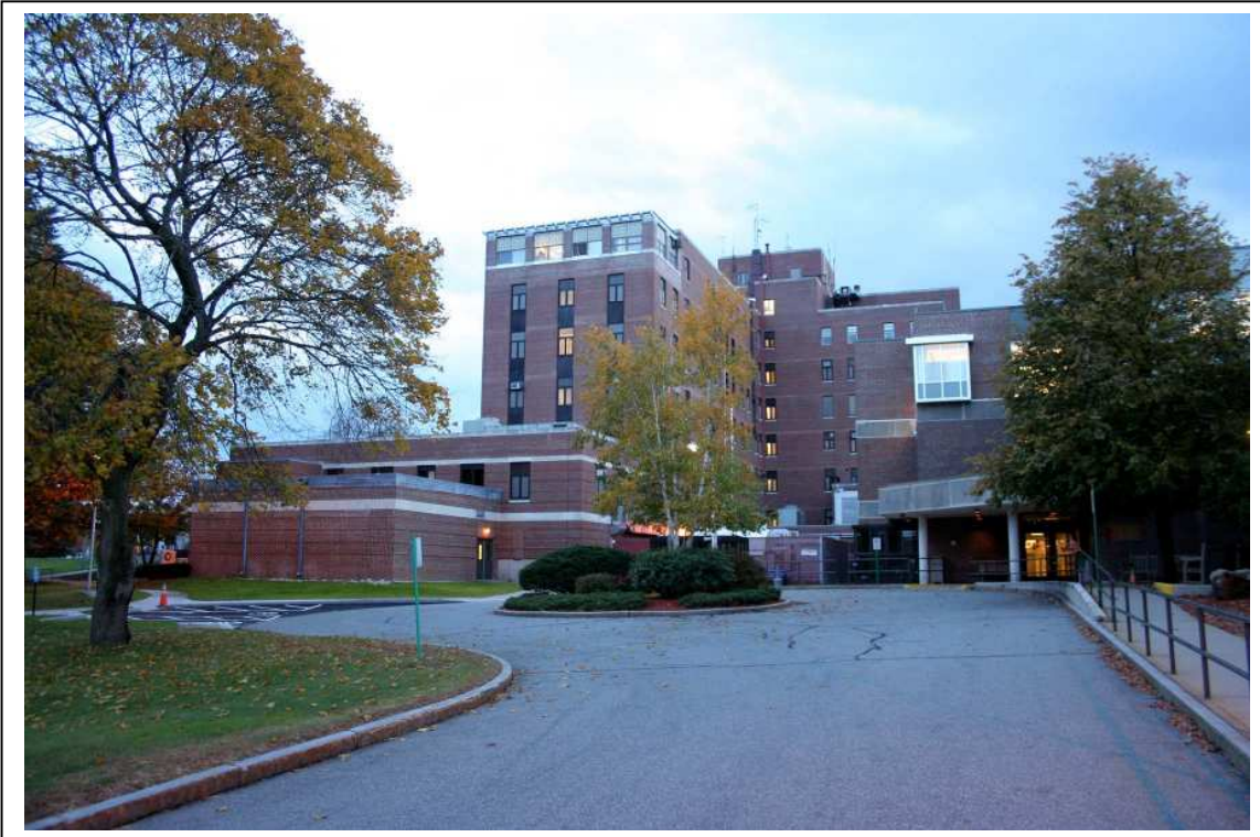
Photo #6: Bldg 1, right side (NE elevation); Bldg 15, Nursing Home Care Unit (1978), at right. Direction: SW
