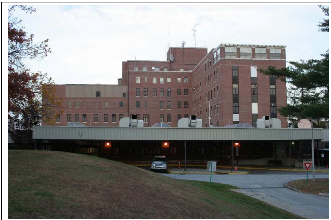
Photo #9: Bldg 1, left side (SW elevation) showing later attached drive-under patient drop-off shelter in foreground. Direction: NE
