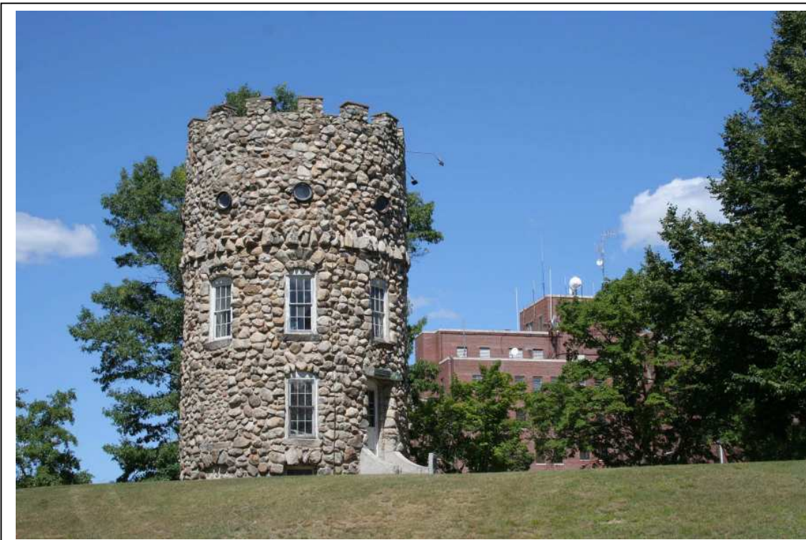
Photo #27: Smyth Tower (Bldg 11, 1888); Hospital (Bldg 1) visible in background. Direction: E
