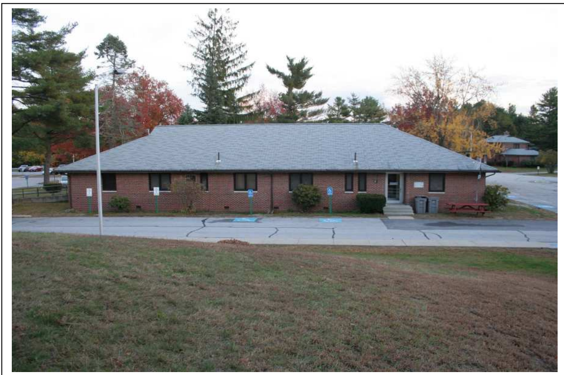
Photo #19: Bldg 5, Nurses Quarters (1948), NW elevation. Direction: SE
