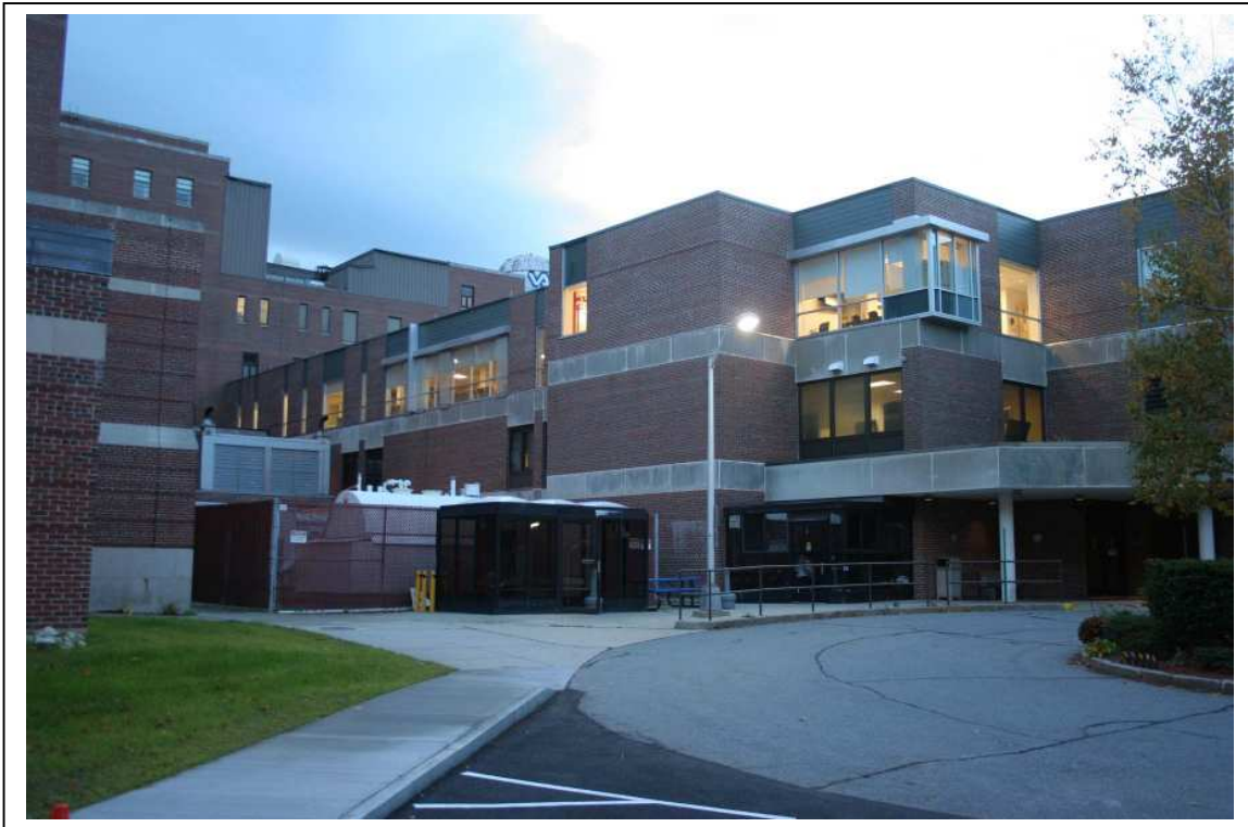
Photo #28: Bldg 15, Nursing Home Care Unit, built 1978, attached to rear wing of Bldg 1. Direction: NW
