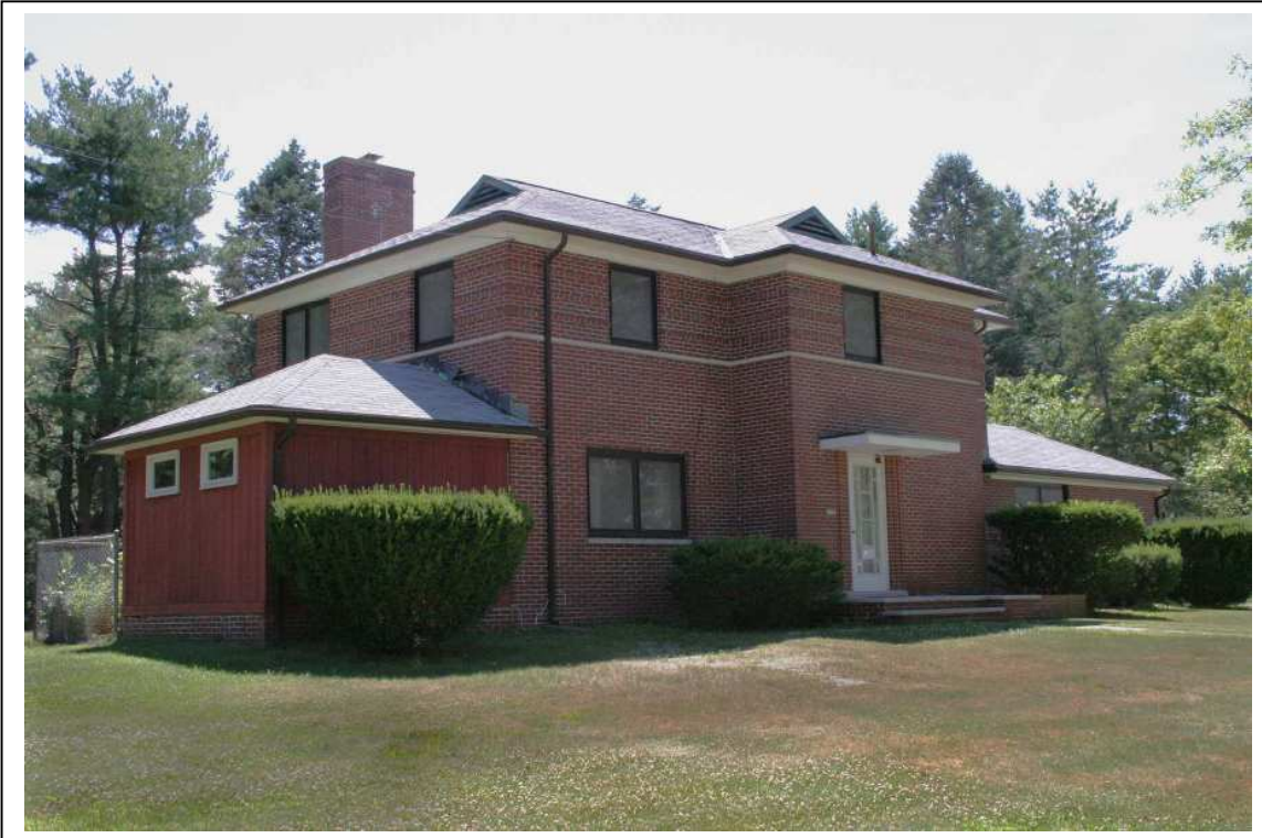
Photo #14: Bldg 2, Manager's Home (1948), front (NE elevation) and left side. Direction: W
