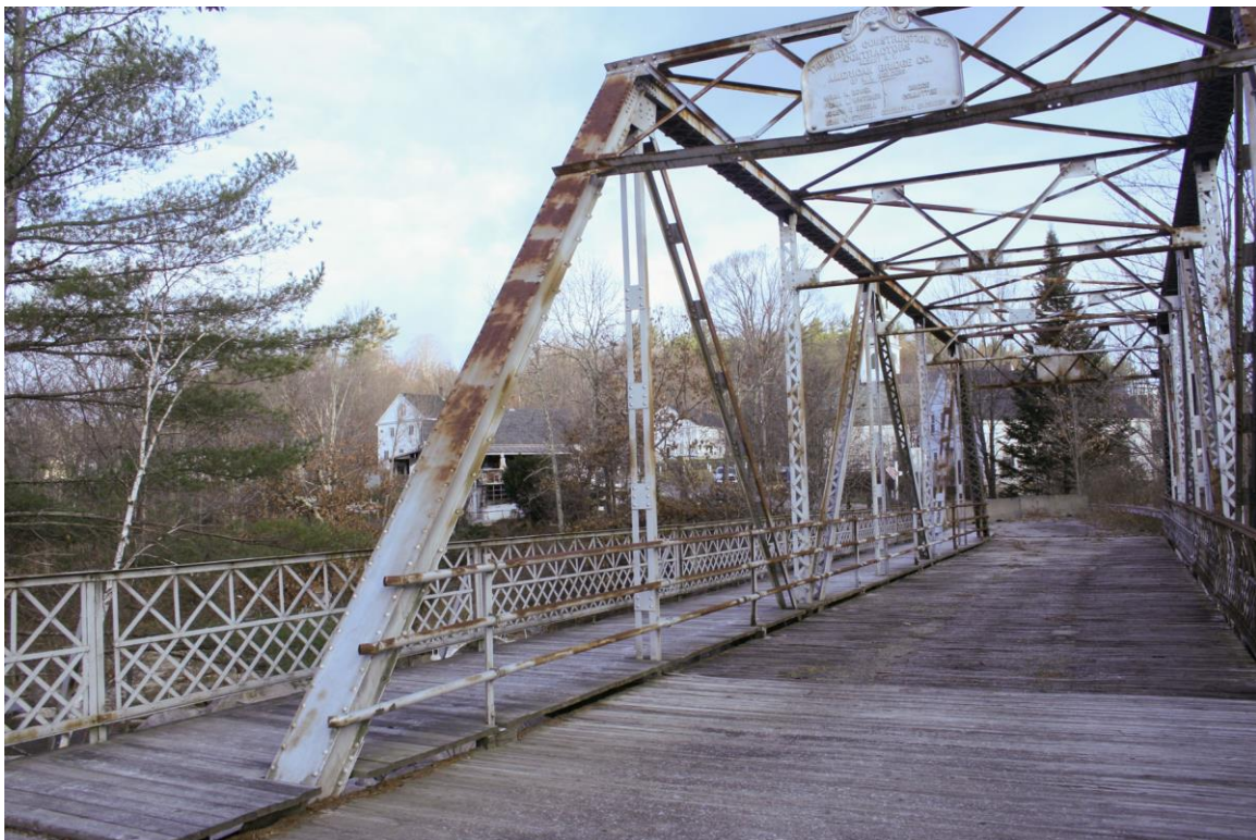
Photo # 5 description: Bridge deck, sidewalk, railing and truss frame details.
