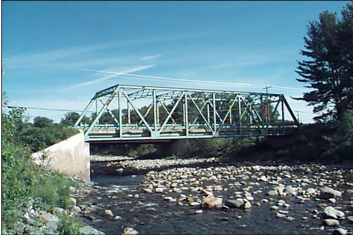
FIGURE 10: COMPARABLE BRIDGE. Bath 134/074, BYPASSED over Ammonoosuc River, built 1928, Repaired 1936. South side of truss, looking north (Source: NHDOT Inspection File Photo, 06/16/1999).
