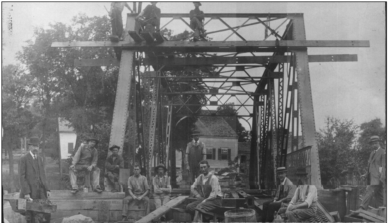
FIGURE 4: Existing steel truss bridge (Wentworth 148/121) shown under construction in 1909 (Source: Wentworth Town Scrap Book).
