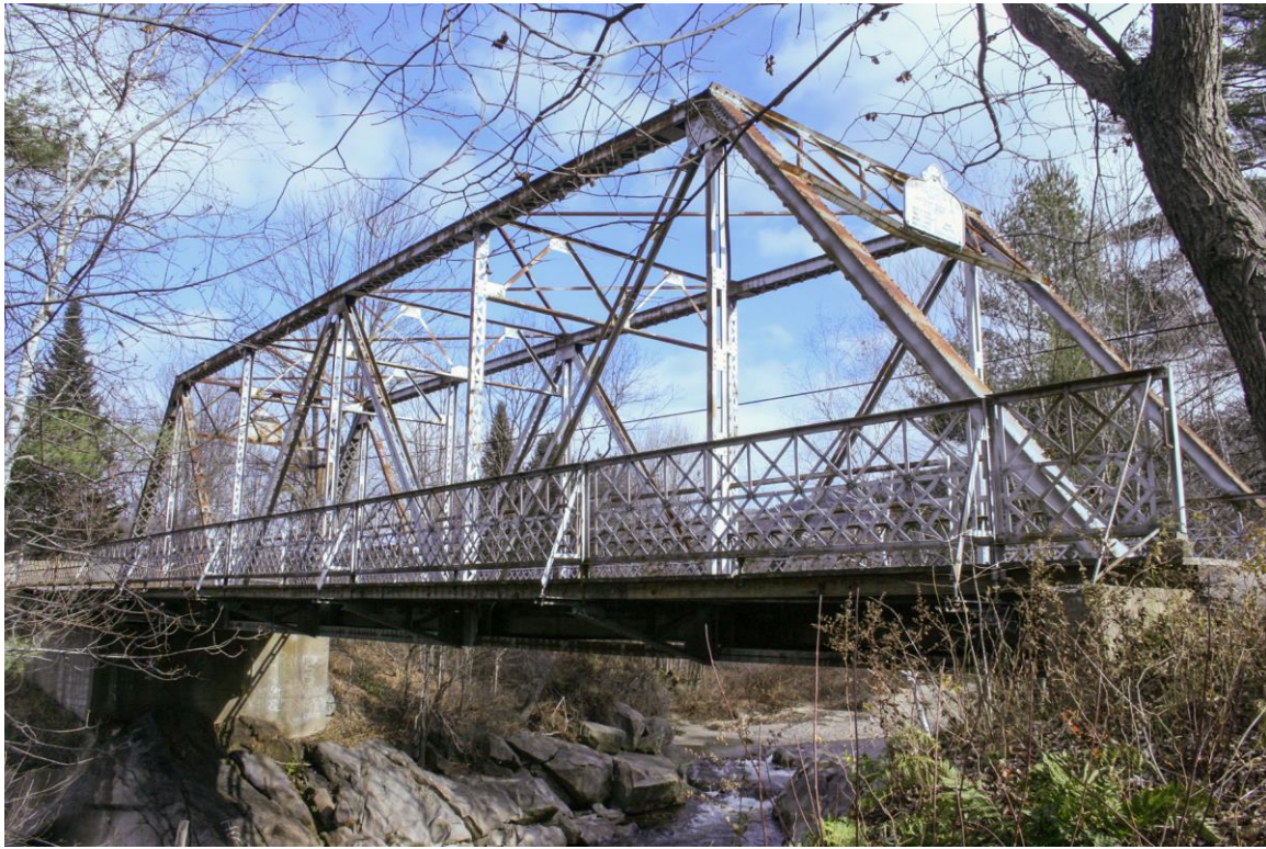
Photo # 4 description: Downstream (west) side of truss.
