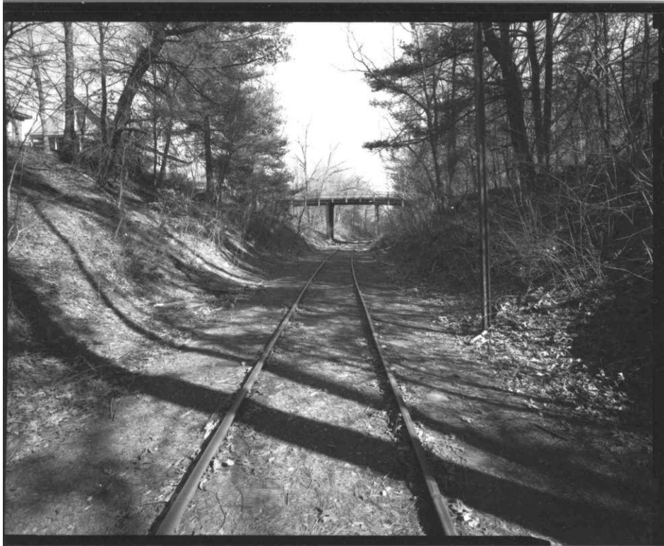
NH-715-3: West elevation and context from railroad tracks. Looking southeast.
