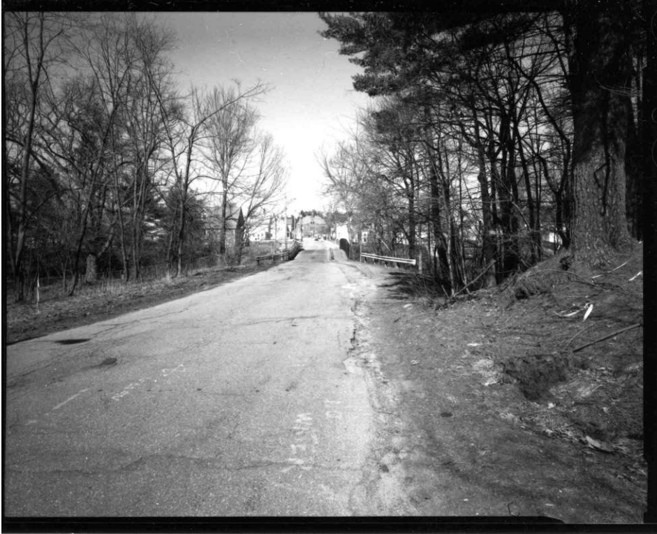
NH-715-1:View of bridge in context from Baldwin Street, south of bridge. Looking northeast.
