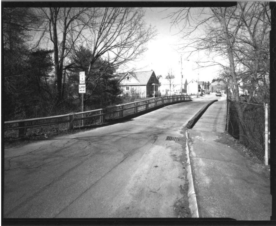
NH-715-5: Roadway deck and sidewalk. Looking northeast.
