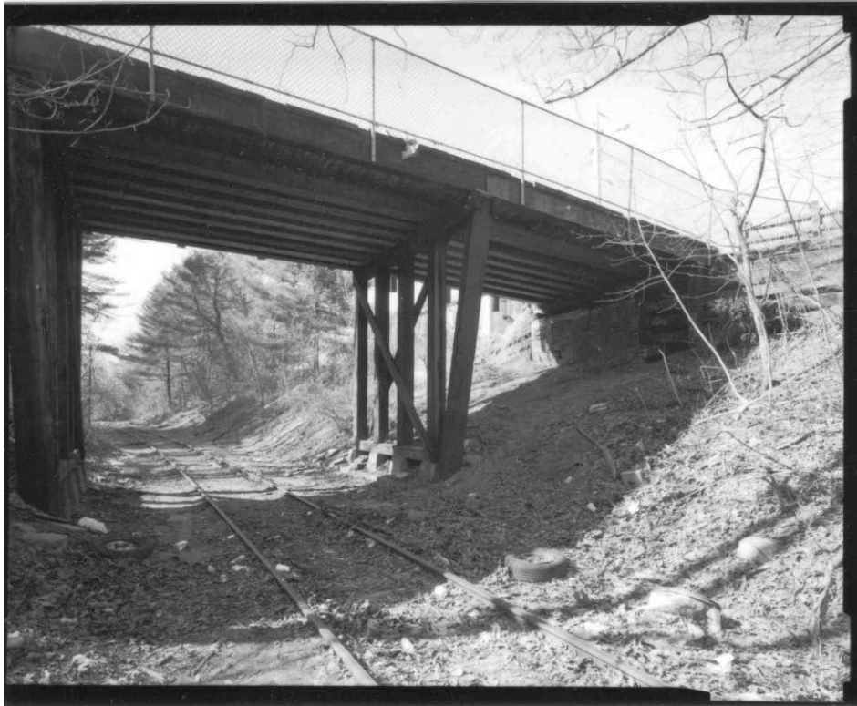
NH-715-6: North bent. Looking north.
