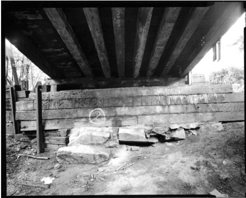
NH-715-10: South timber retaining wall (former pier). Looking southwest.
