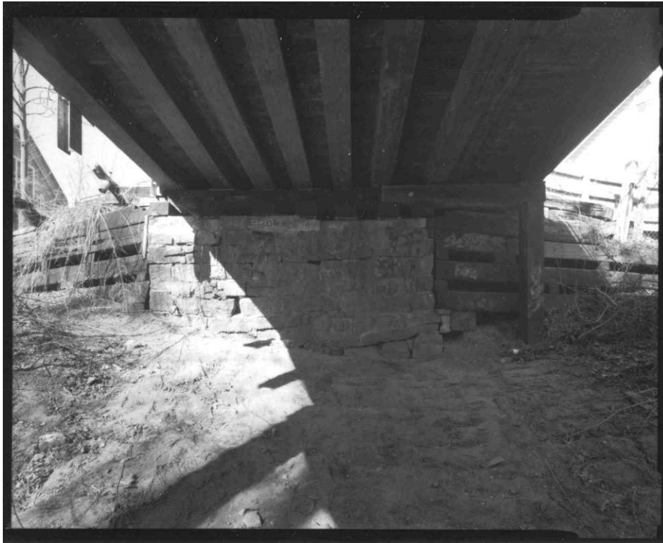
NH-715-7: North abutment and underside of deck. Looking northeast.
