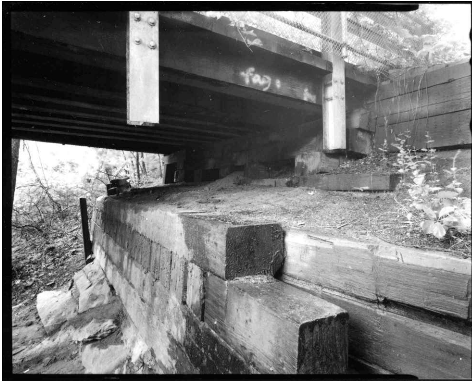
NH-715-11: Oblique view of south abutment. Looking southeast.
