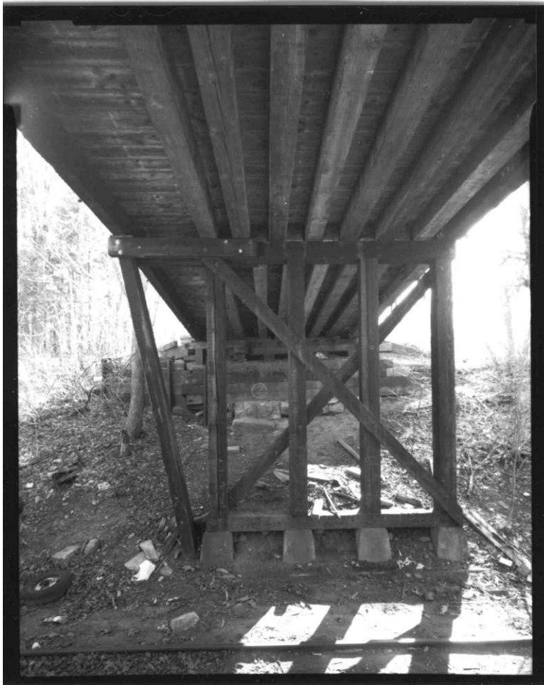
NH-715-8: South abutment, south bent and underside of deck. Looking southwest.
