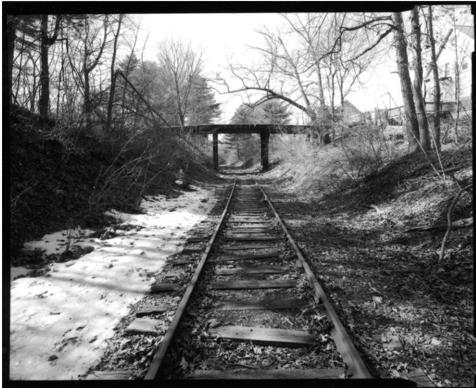
NH-715-2: East elevation and context from railroad tracks. Looking northwest.
