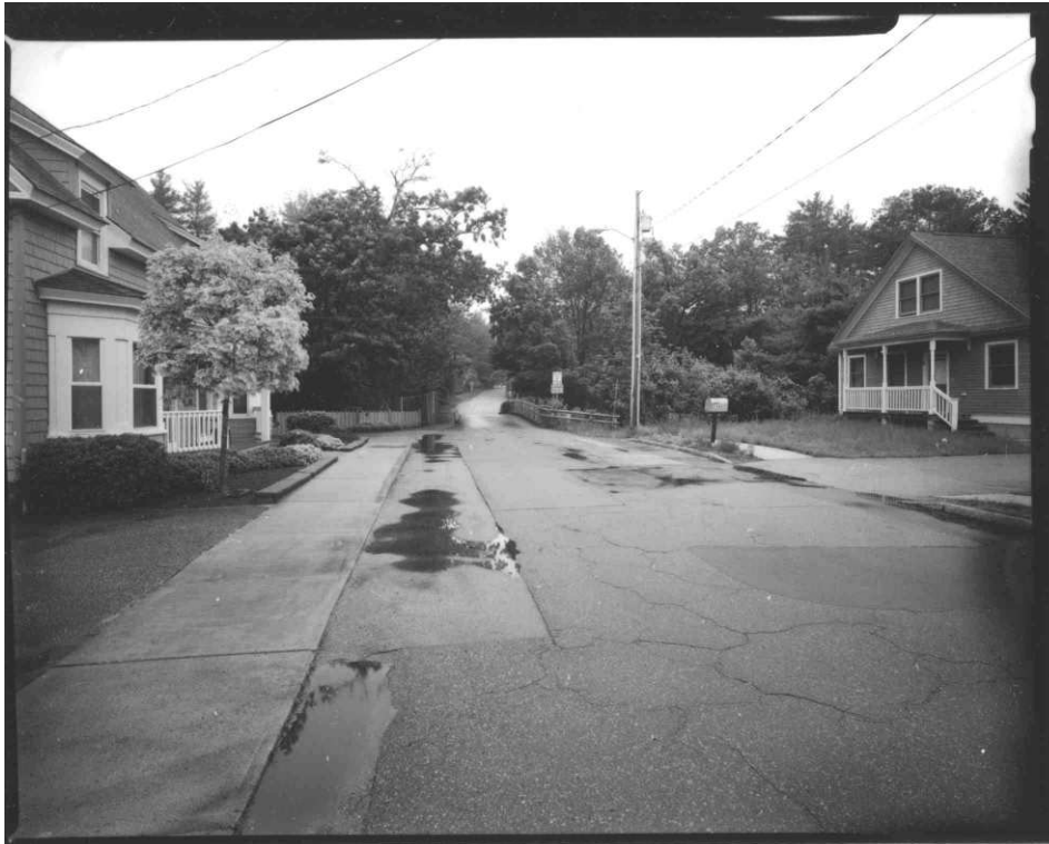
NH-715-9: View of bridge in context from Baldwin Street, north of bridge. Looking southwest.
