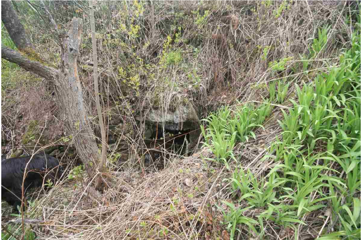
Photo # 79 description: Culvert No. 110.15, Lisbon. Stone box, 3-0, fieldstone. nd. Outlet.
