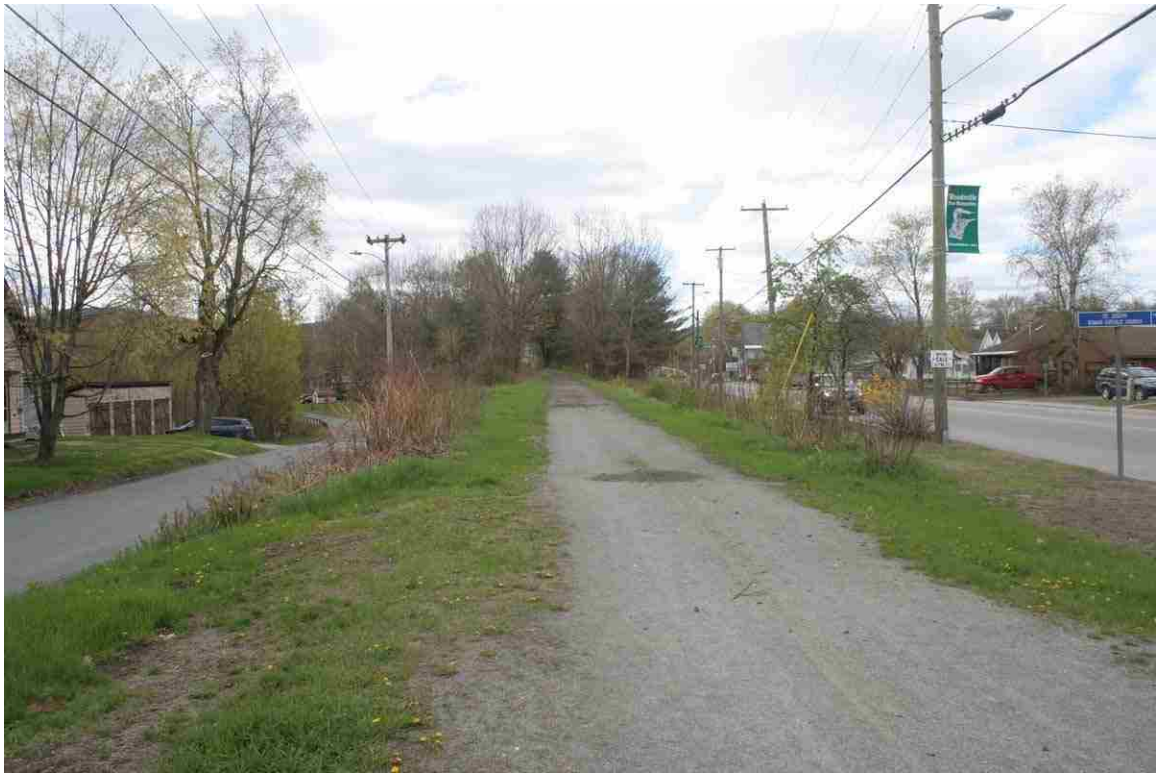
Photo # 11 description: Railbed (trail), Woodsville, character along Central St., right and Railroad St., left. mp 93.68.
