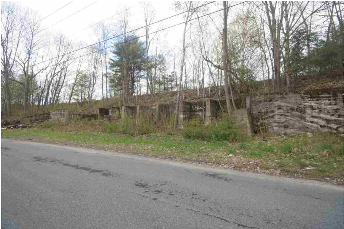
Photo # 12 description: C.E. Randall Coal Pockets, Mill St., Woodsville. Reinforced concrete. mp 93.70. c.1900.
