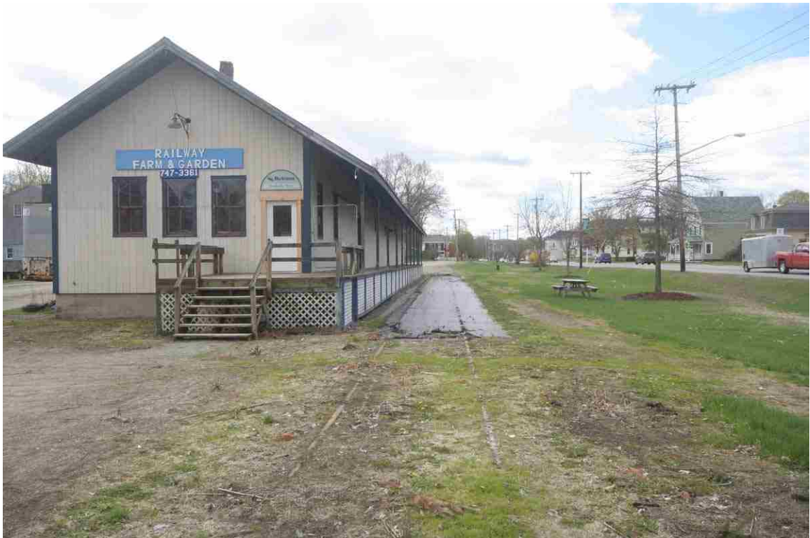
Photo # 10 description: Freight Building No. 2, Woodsville, north side, showing remaining track. mp 93.65. nd.
