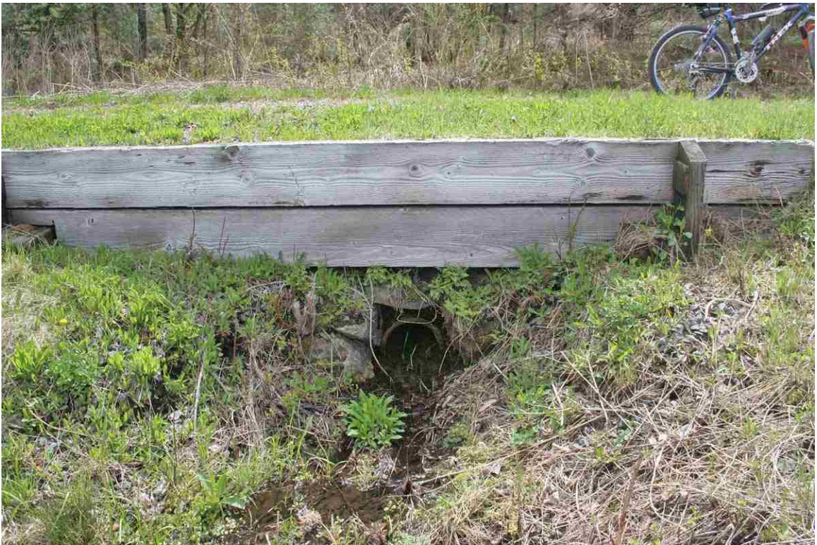
Photo # 50 description: Culvert No. 103.05, Landaff. Vitreous pipe, 1-0. nd. Outlet.
