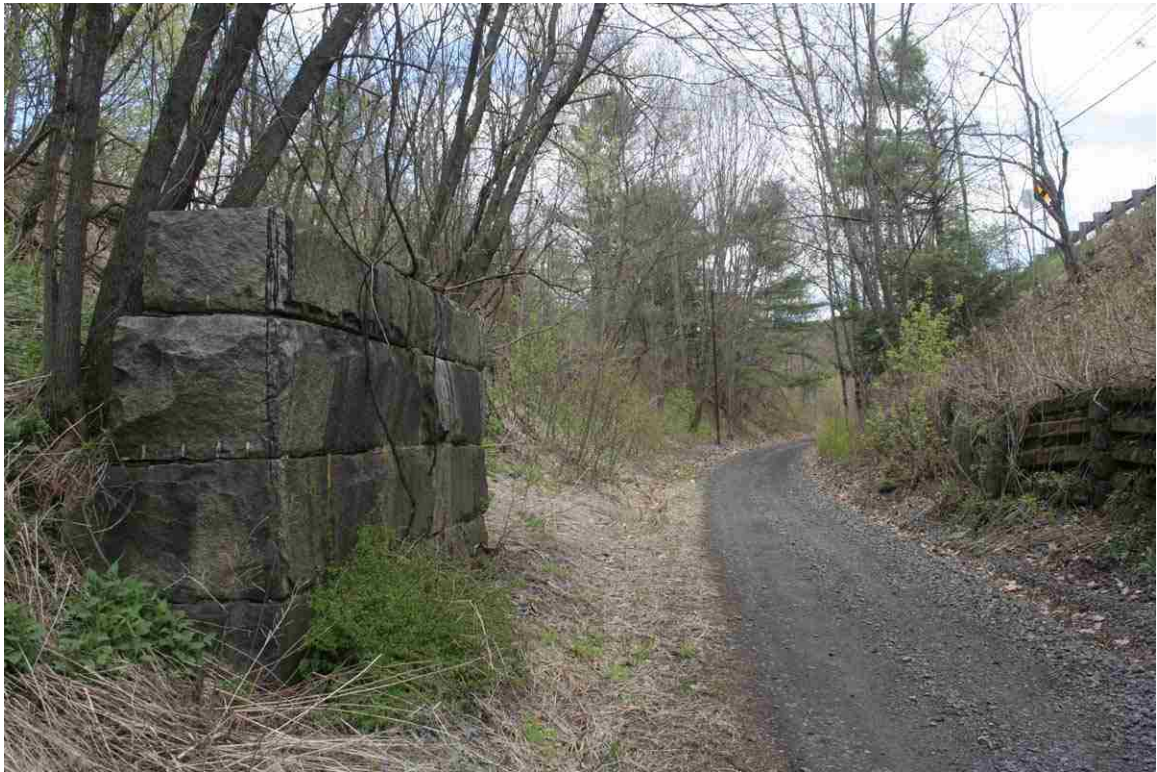
Photo # 43 description: Bridge 101.52, Bath. Detail of stonework, clearly by B&M. (3 of 3).
