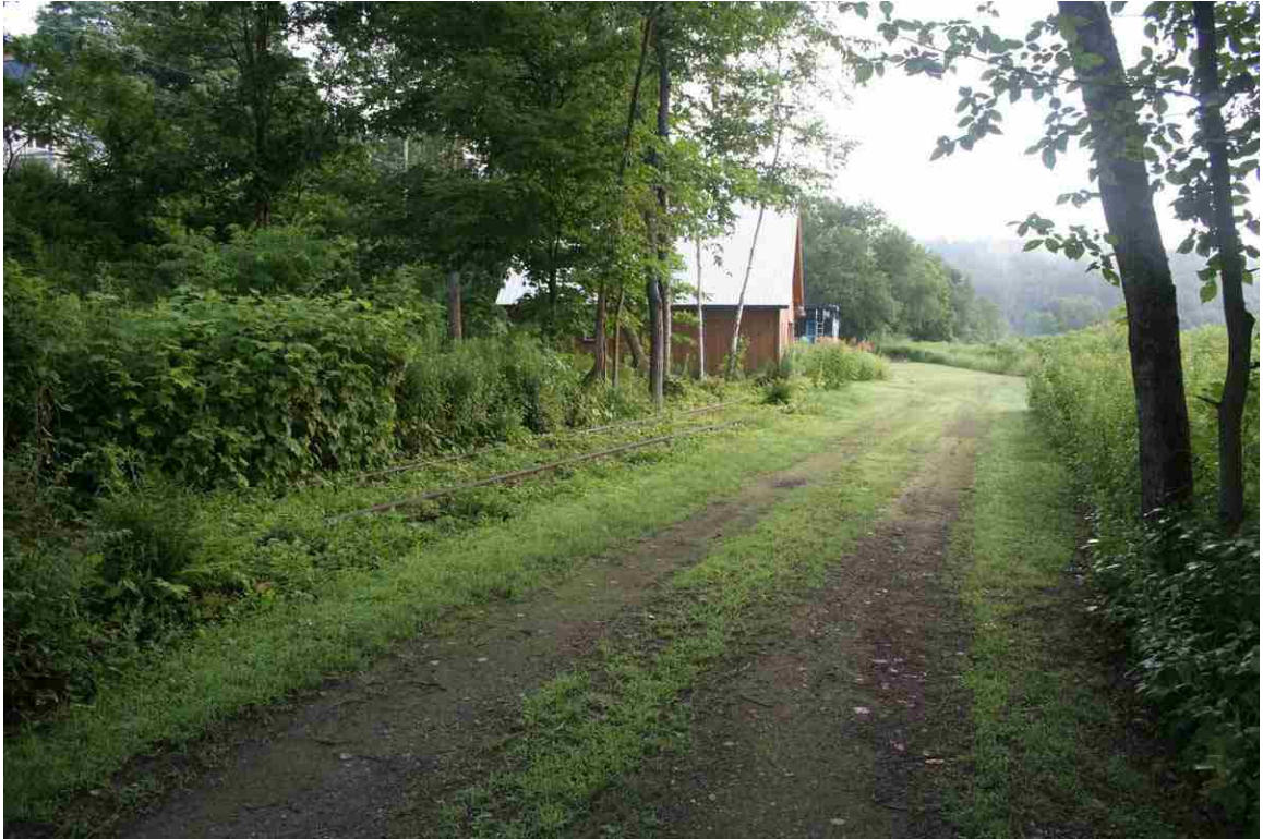
Photo # 33 description: Railbed, east of Bath Covered Bridge, showing siding track for Bath Station in weeds at left. mp ~ 98.33. nd.
