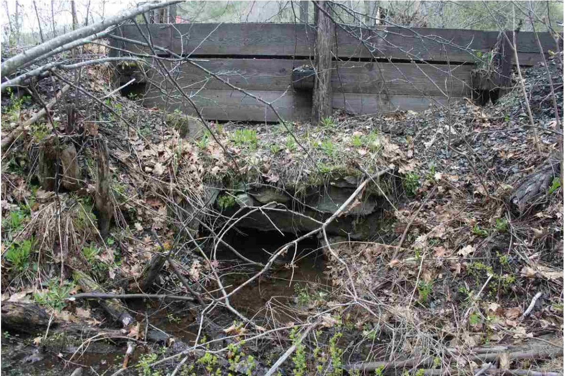
Photo # 53 description: Culvert No. 103.12, Landaff. Stone box, 3-0, fieldstone. nd. Outlet.
