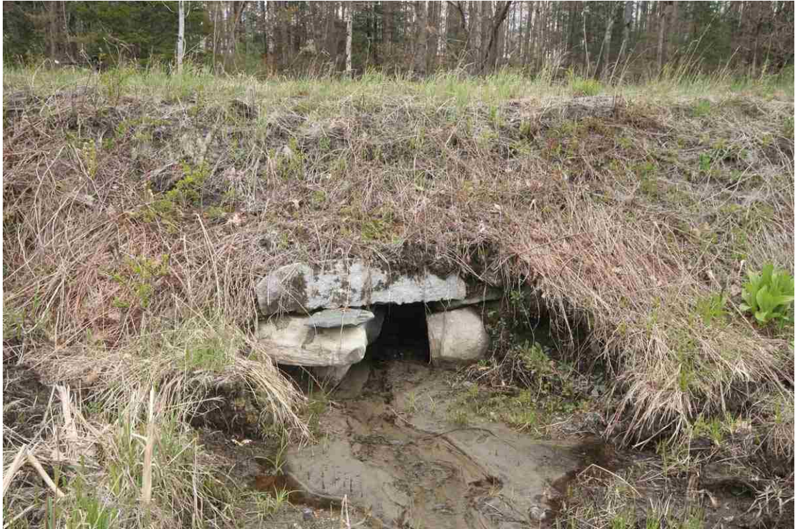
Photo # 85 description: Culvert No. 111.90, Littleton. Stone box, 3-0, fieldstone. Outlet. nd.
