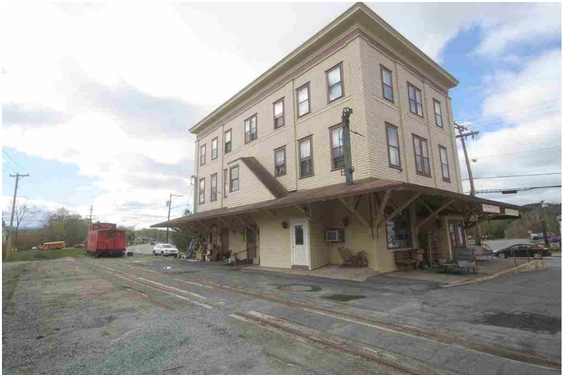
Photo # 5 description: Woodsville Station, Track side, with track remaining. mp 93.60. 1890, 1921.
