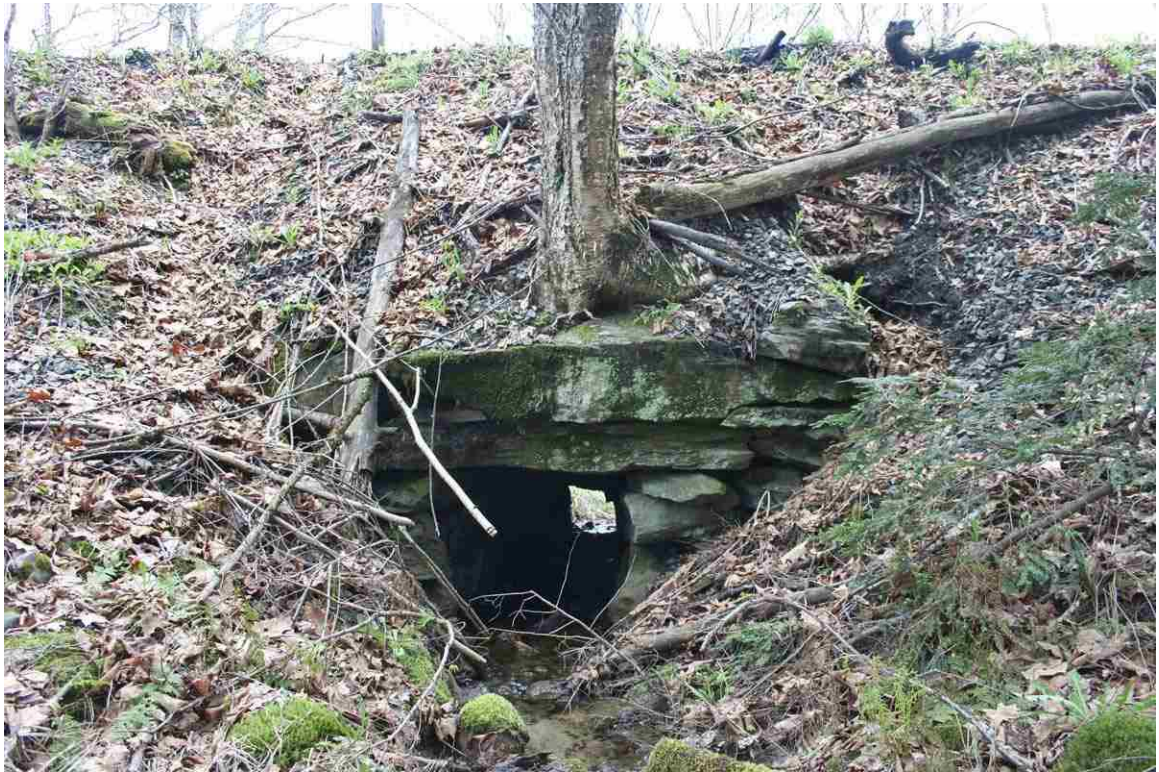
Photo # 47 description: Culvert No. 102.69, Landaff. Stone box, 3-6. nd. Inlet. (1 of 2).
