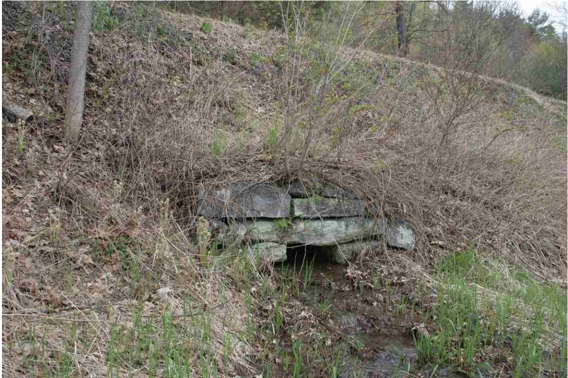
Photo # 39 description: Culvert No. 98.97, Bath. Stone box, 3-0. nd.
