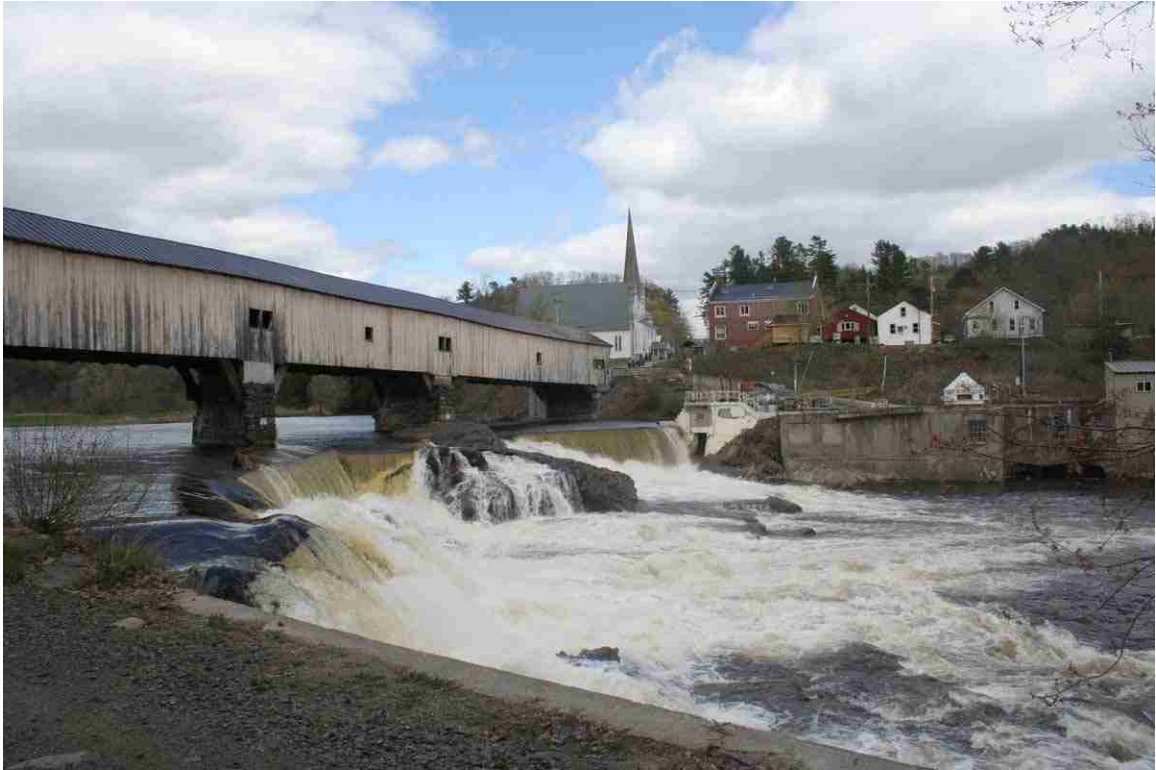
Photo # 31 description: Railbed in foreground at Bath Village. Concrete retaining wall, evidently built by railroad, supports railbed along edge of Ammonoosuc R. mp 98.33. nd.
