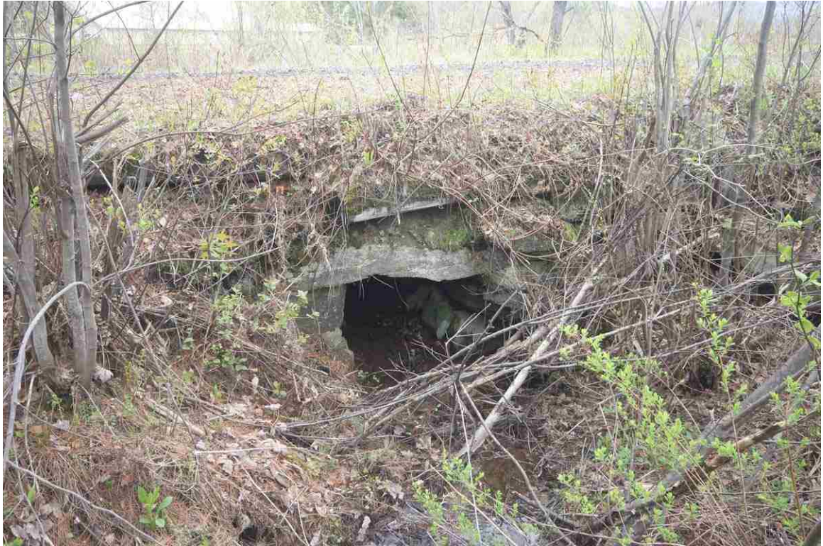
Photo # 81 description: Culvert No. 111.11, Littleton. Stone box, 3-0, fieldstone. nd. Inlet.
