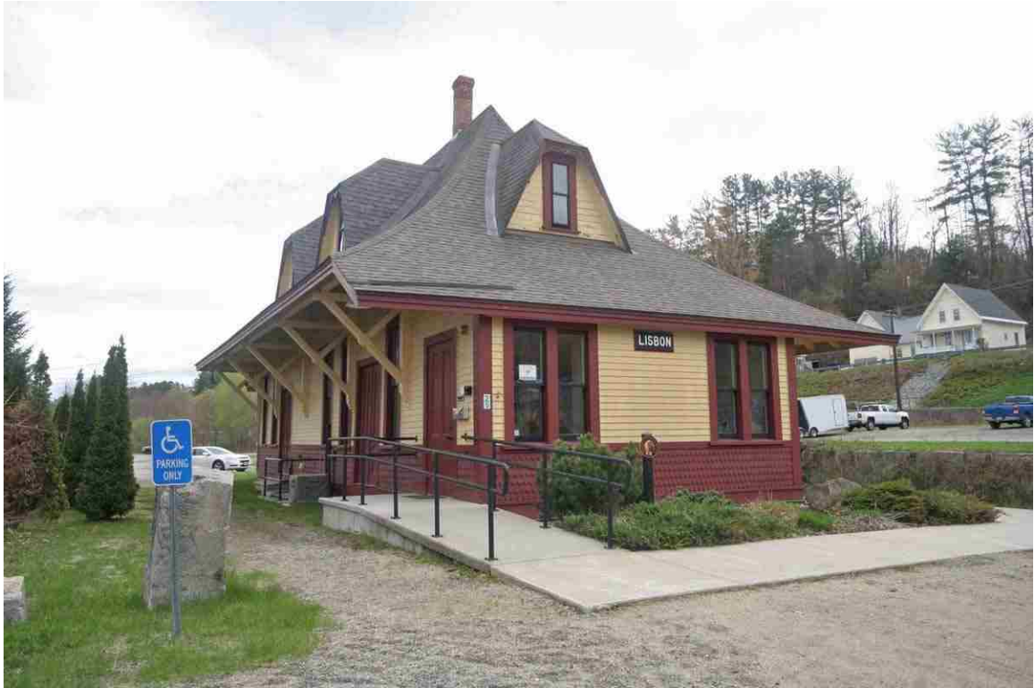
Photo # 57 description: Lisbon Station, North and west sides. mp 103.81. 1869. SR listed 2008. (2 of 2)
