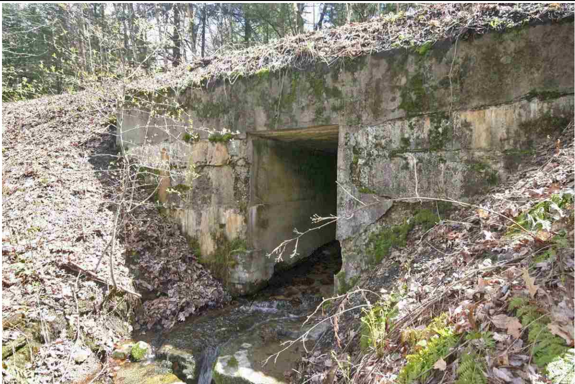
Photo # 22 description: Culvert 96.27, Bath. Railtop. Outlet. 1921. (2 of 2).
