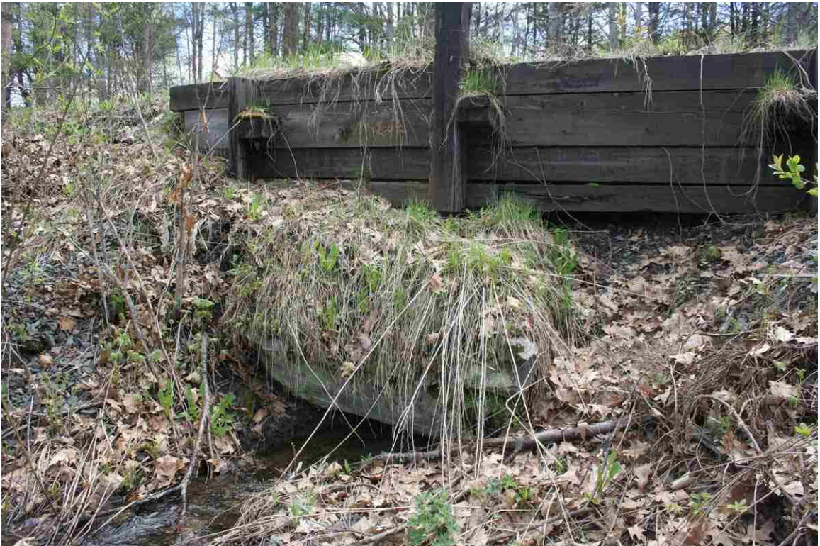
Photo # 54 description: Culvert No. 103.21, Landaff. Stone box, 3-0, fieldstone. nd. Outlet.
