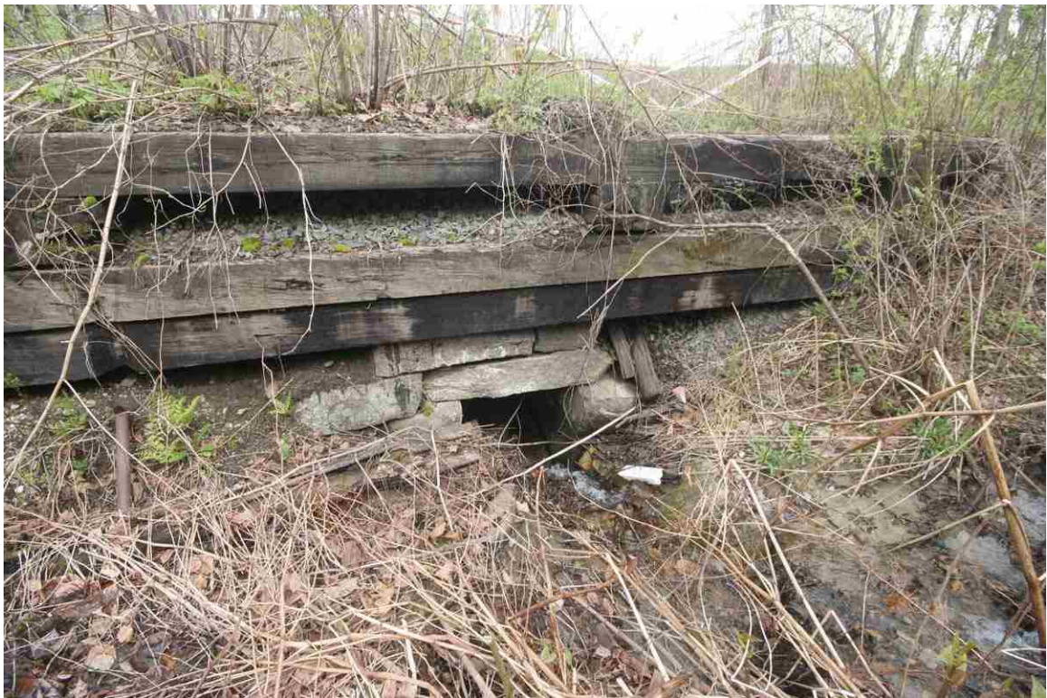
Photo # 58 description: Culvert No. 104.02, Lisbon. Stone box, 3-0, fieldstone. nd. Outlet.
