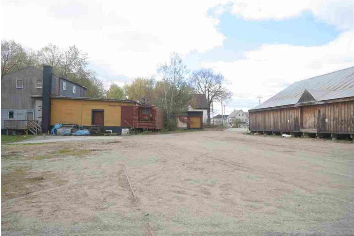
Photo # 9 description: Freight Building No. 3, Woodsville, north side. mp 93.65. nd. Note siding track and freight car remain. East side of Freight Building No. 2 at right.
