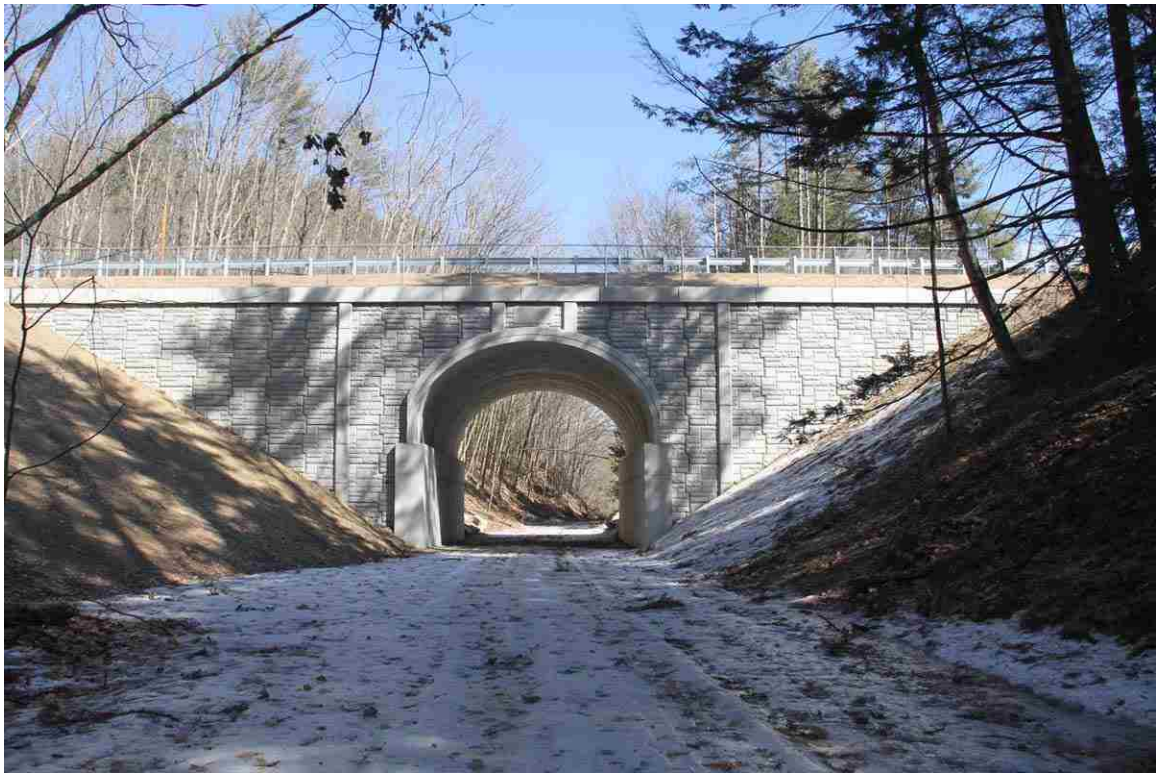
Photo # 13 description: Mill Street underpass, Woodsville. Precast reinforced concrete. mp 94.79. 2018.
