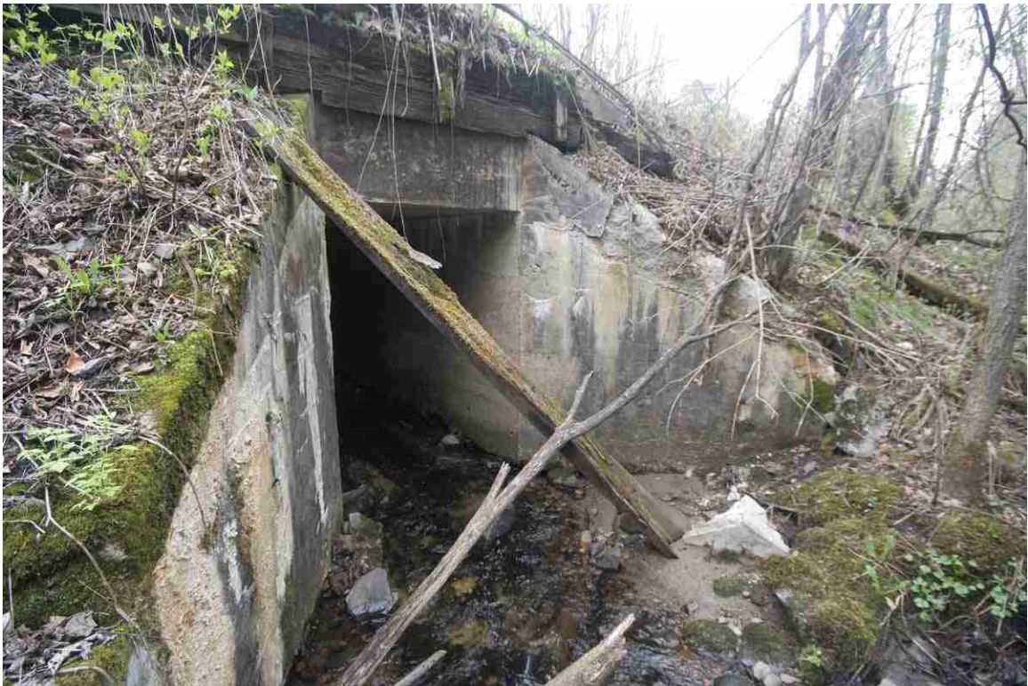
Photo # 70 description: Culvert No. 107.50, Landaff. Railtop concrete slab. 4-0. nd. Inlet. (2 of 2).
