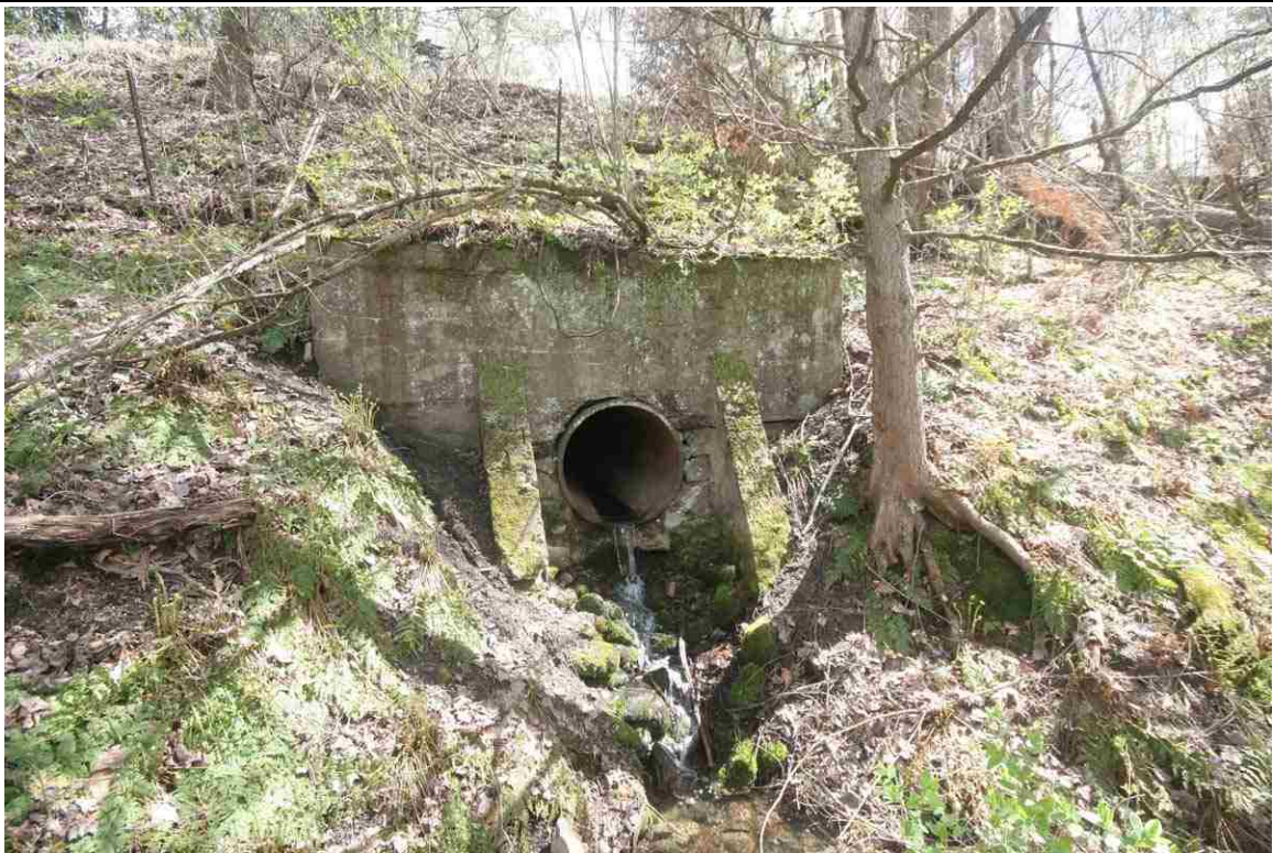
Photo # 20 description: Culvert No. 96.21, Bath. Cast iron pipe, 18", concrete headwalls. Outlet. 1924.
