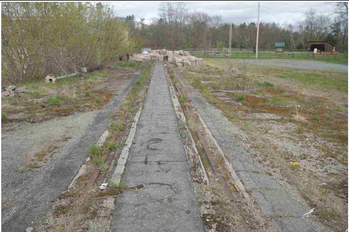
Photo # 4 description: Railroad Park, Woodsville. Railbed with track remaining west of Station. mp 93.60. nd (no date, date unknown).
