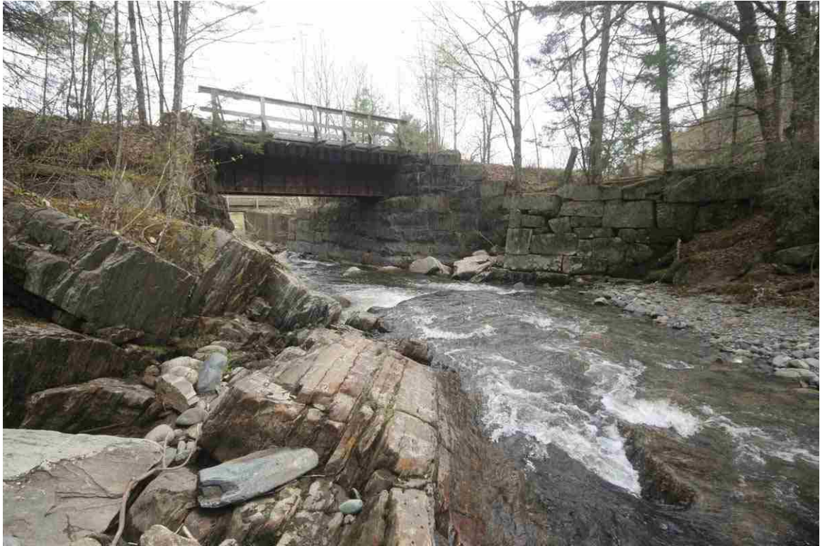
Photo # 67 description: Bridge 106.43, over Sugar Hill Brook, Lisbon. Steel deck plate girder, 21'-4" span. 1914. Upstream side. (2 of 2).
