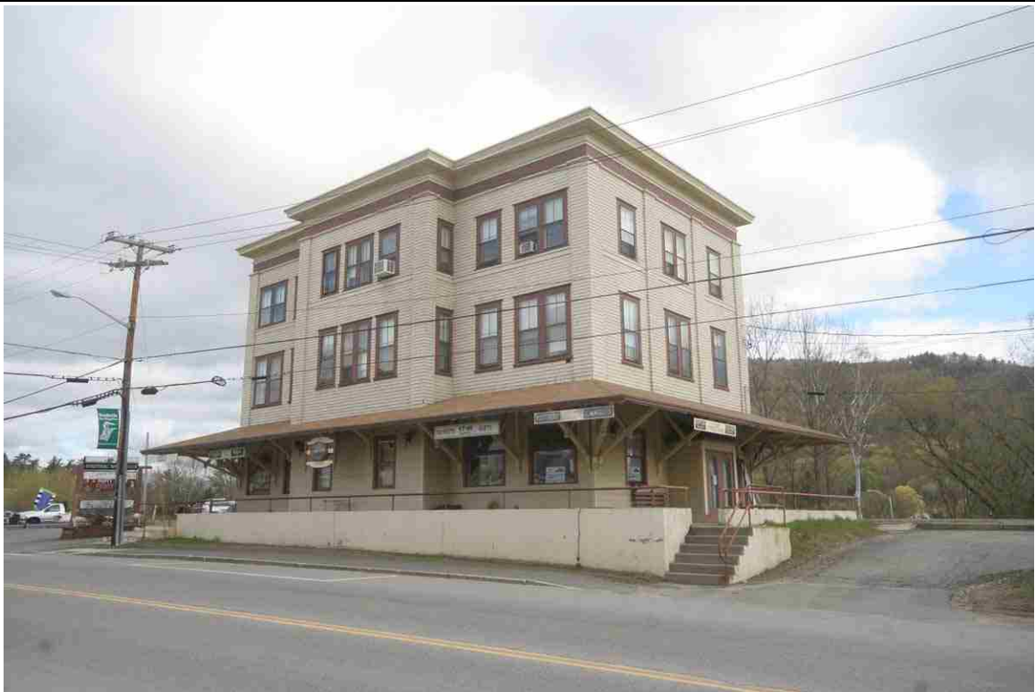
Photo # 6 description: Woodsville Station. Street side, with track remaining. mp 93.60. 1890, 1921.
