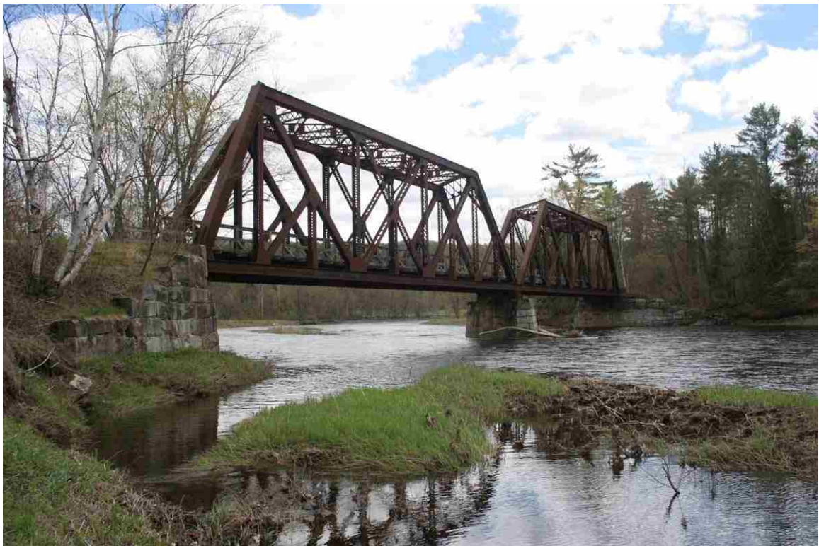
Photo # 40 description: Bridge No. 100.23 over Ammonoosuc R., Bath. Riveted 2-span thru-truss, 265'. 1911.
