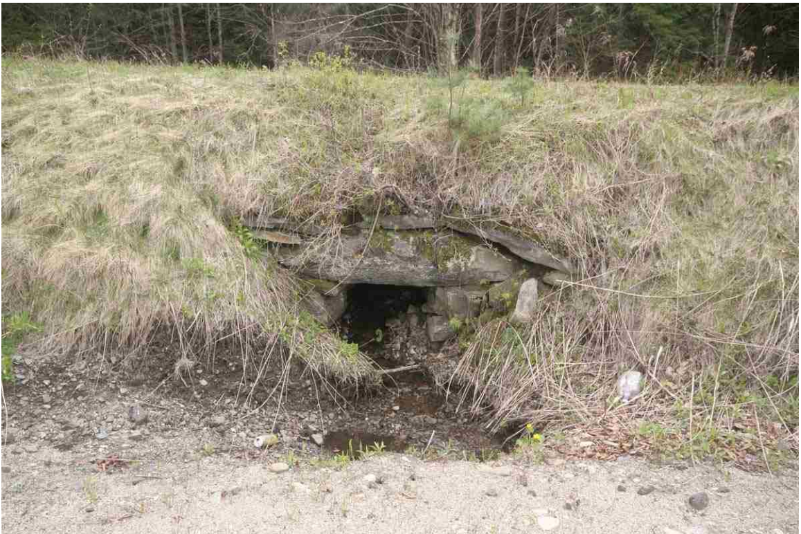
Photo # 68 description: Culvert No. 107.14, Lisbon. Stone box, 3-0, Fieldstone. nd. Outlet.
