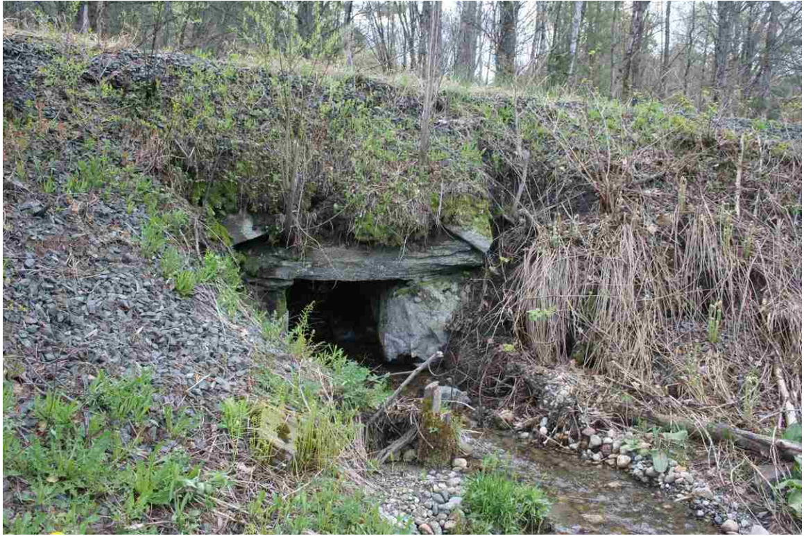
Photo # 51 description: Culvert No. 103.08, Landaff. Stone box, 2-6, fieldstone. nd. Outlet. (1 of 2)
