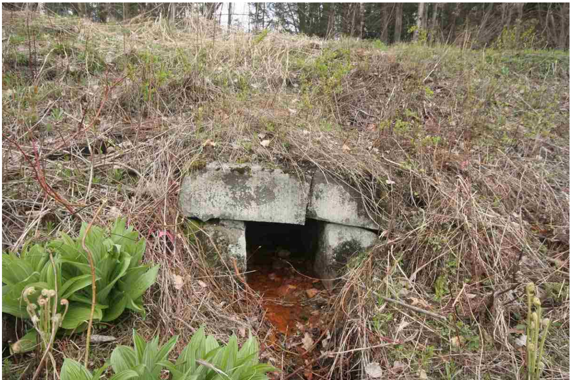
Photo # 86 description: Culvert No. 111.98, Littleton. Stone box, 2-6, quarry stone. Outlet. nd.
