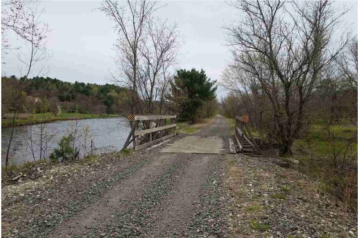
Photo # 59 description: Bridge 104.49 over Pearl Lake Brook, Lisbon. Steel deck plate girder, 22'-7" span. 1921. West approach. (1 of 3).
