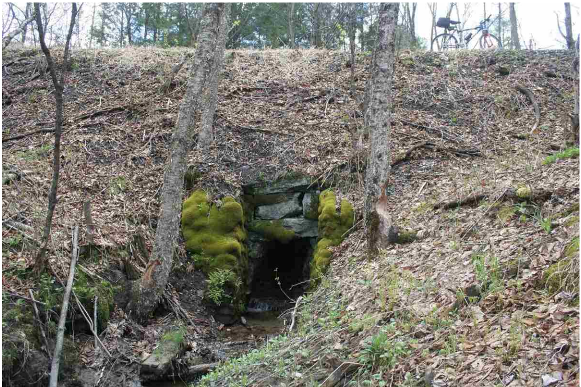
Photo # 48 description: Culvert No. 102.69, Landaff. Stone box, 3-6. nd. Deeply buried (14'-6"). Outlet. (2 of 2).
