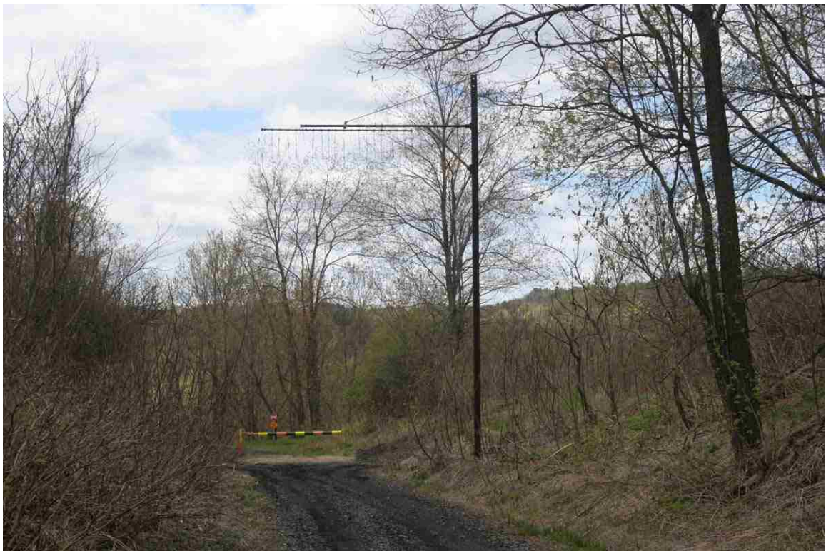
Photo # 44 description: Tell Tale, Bath. Steel poles with hanging chains to indicate clearance of overhead bridge 101.52 remain about 400 feet east and west of bridge crossing. West pole shown.
