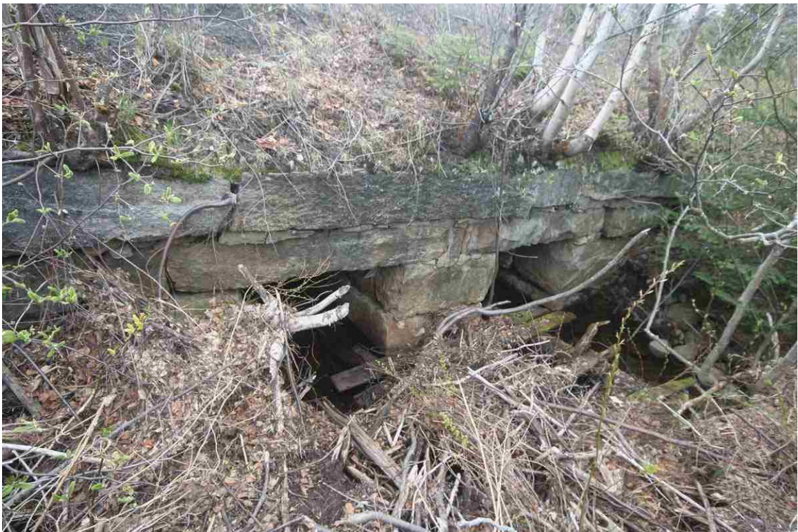
Photo # 48 description: Culvert 140.21, Randolph. Inlet. (2 of 2).
