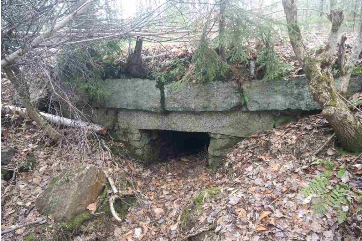
Photo # 59 description: Culvert 142.33, Randolph. Stone box, 36", mixed split quarry & fieldstone. nd.
