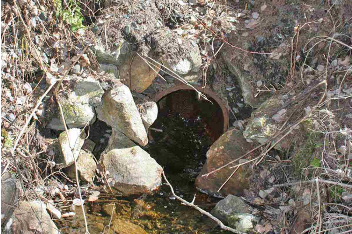
Photo # 13 description: Culvert 132.85, Jefferson. Cast iron pipe, 18"; rubble rip rap. 1898.
