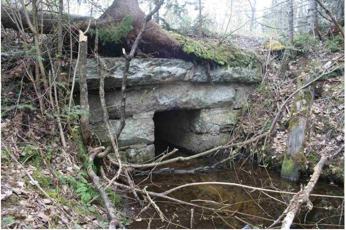
Photo # 17 description: Culvert 133.51, unnamed stream, Jefferson. Stone box, 36". nd.
