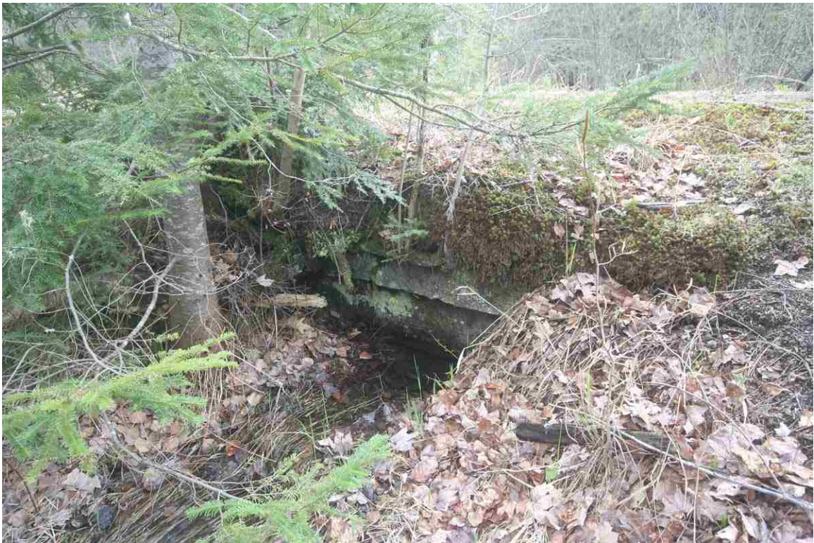
Photo # 108 description: Culvert 147.62, Gorham. Stone box, 24", mixed split quarry & fieldstone. nd.
