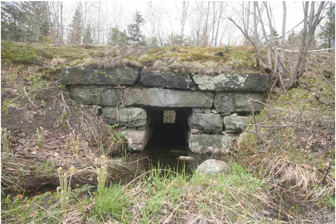
Photo # 72 description: Culvert 143.57, Randolph. Stone box, 36", quarry stone. nd.
