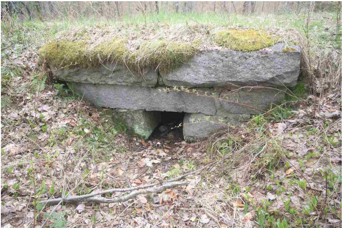
Photo # 42 description: Culvert 138.67, Randolph. Stone box, 30", quarry-split stone. nd.
