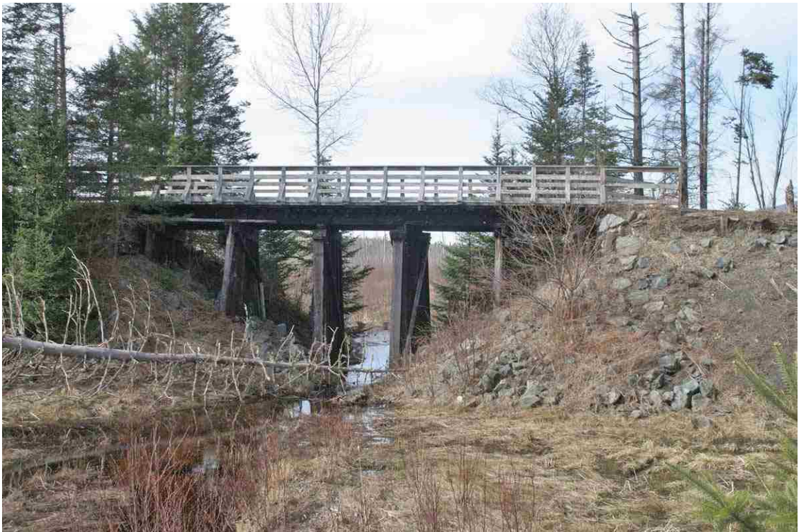
Photo # 12 description: Bridge 132.61 over Stanley Slide Brook, Jefferson. Framed pile trestle, 51', 7-spans. 1926.
