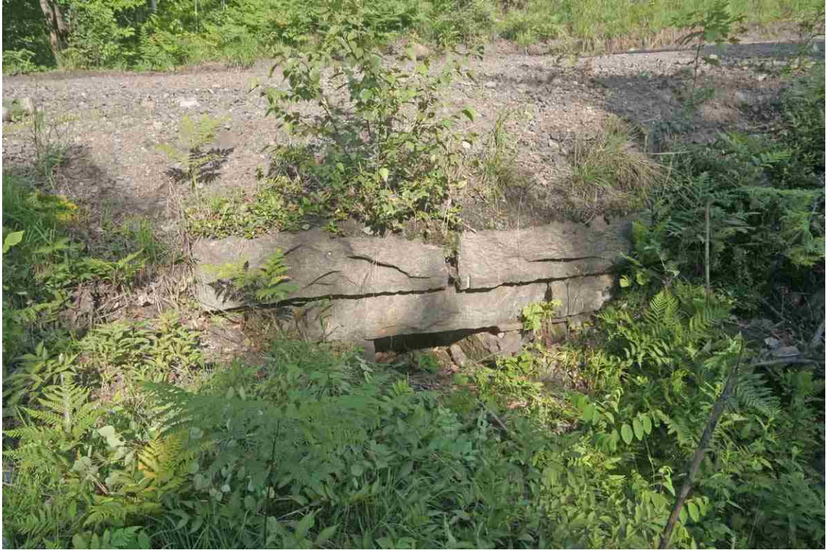
Photo # 123 description: Culvert 150.44, Gorham. Stone box, 36", quarry stone. nd.
