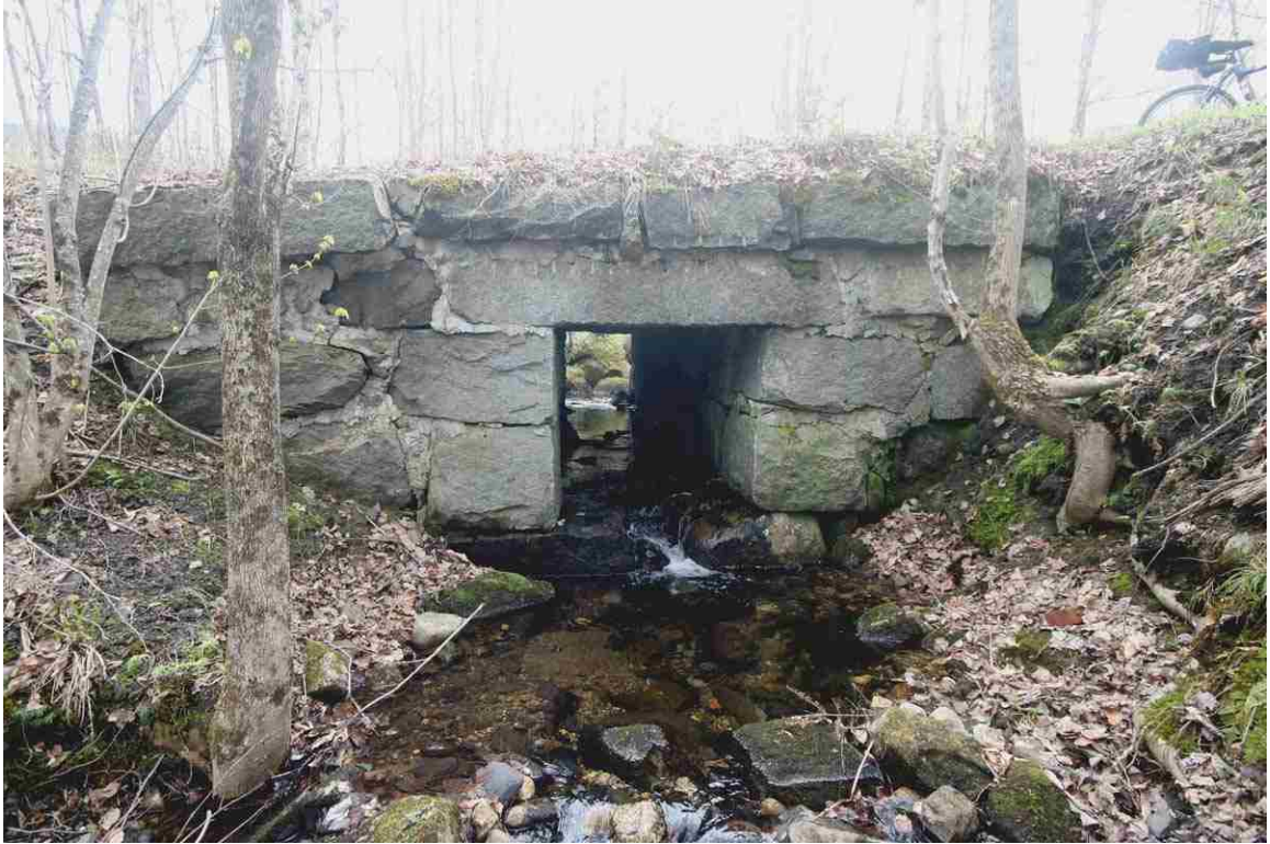
Photo # 71 description: Culvert 143.41, Randolph. Stone box, 48", split quarry stone. nd.
