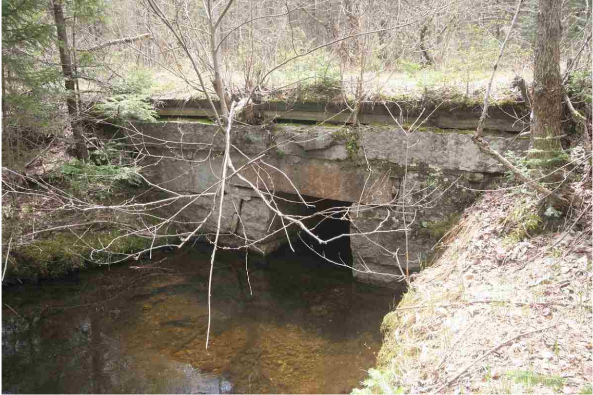
Photo # 79 description: Culvert 144.70, Randolph. Stone box, 48", split quarry stone. nd.
