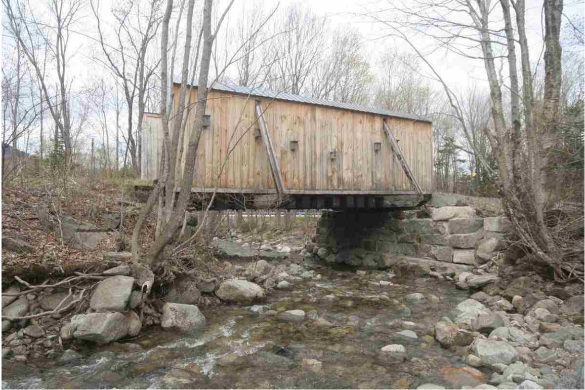
Photo # 67 description: Bridge 143.06 over Snyder Brook, Randolph. Upstream side. Note siding recently replaced. US2 paralleling RR ROW 150' north, just visible under bridge. (2 of 3).
