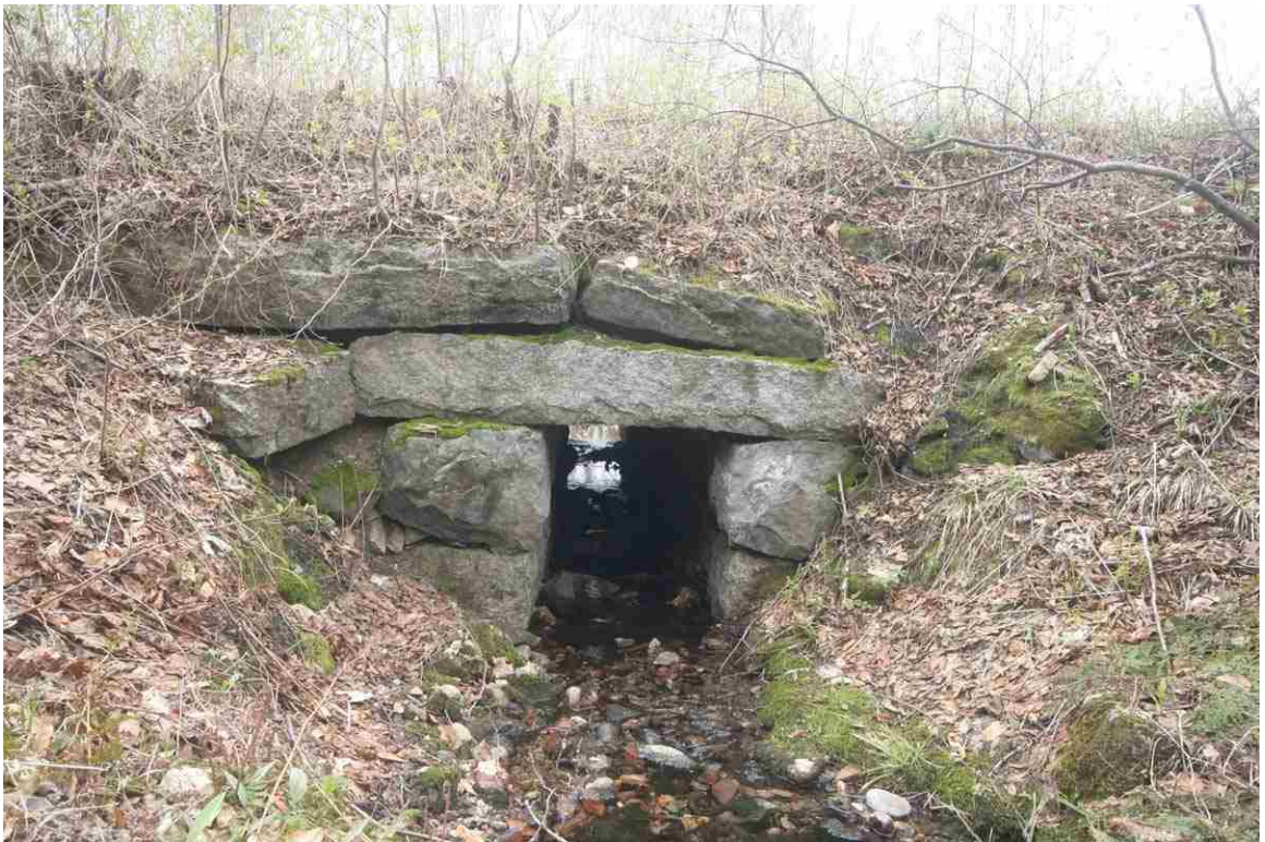
Photo # 74 description: Culvert 143.77, Randolph. Stone box, 36", mixed split quarry & fieldstone. nd.
