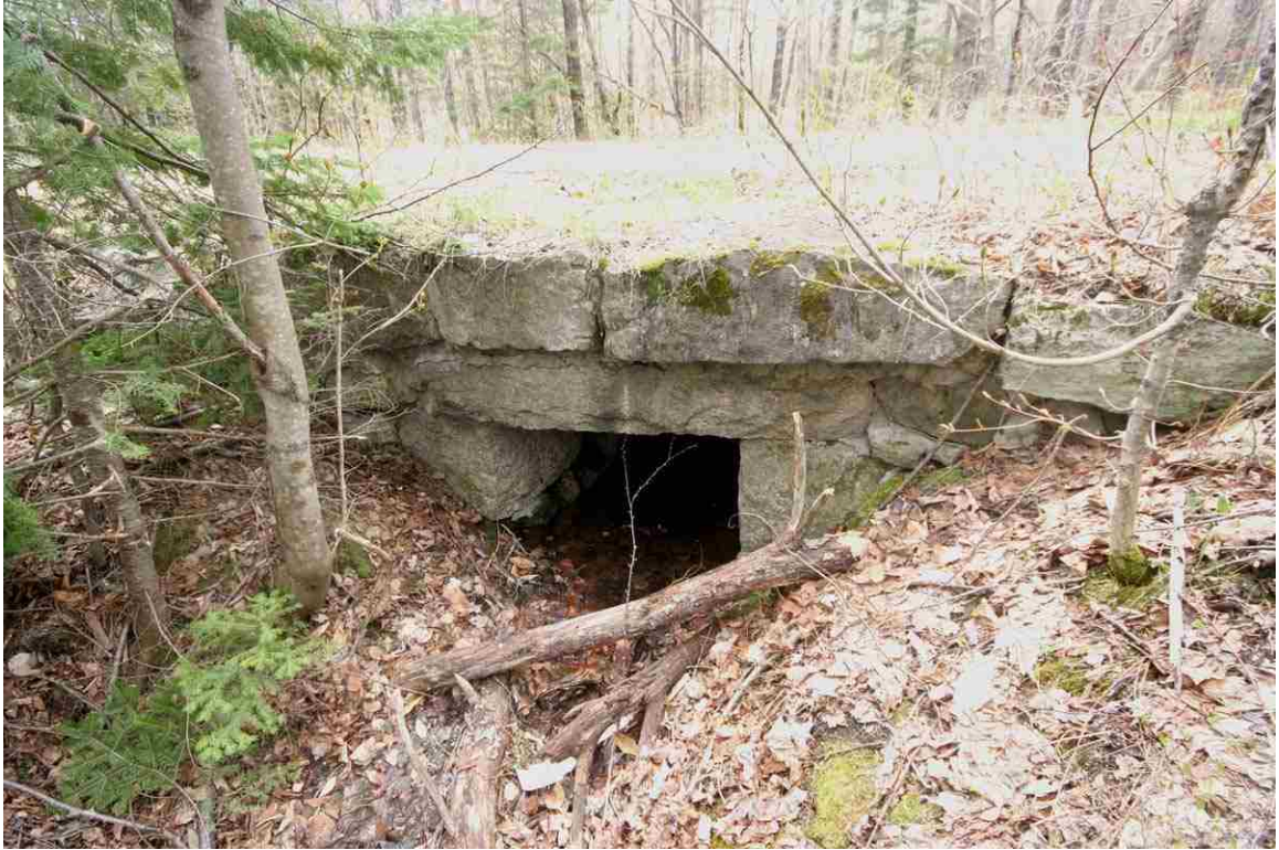
Photo # 77 description: Culvert 144.21, Randolph. Stone box, 48", quarry stone. nd.
