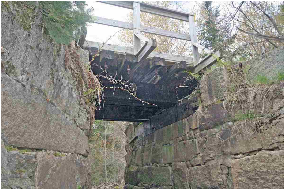
Photo # 20 description: Bridge 133.80, underside, showing two massive treated timber stringers. (2 of 2).
