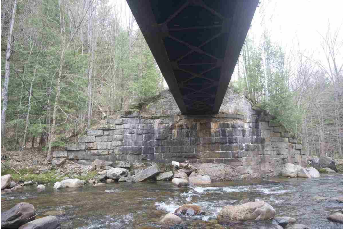
Photo # 105 description: Bridge 146.80, Gorham, "Moose River Bridge No. 3." East abutment.
