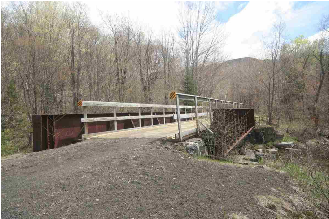
Photo # 86 description: Bridge 145.43, Gorham, "Moose River Bridge No. 1." Steel thru plate girder, 49' span, on stone abutments. 1917 (erection date). (1 of 3).
