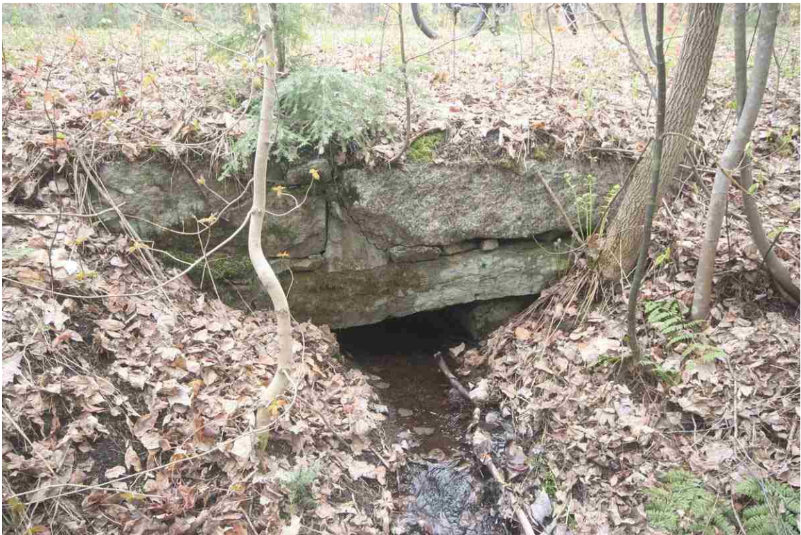
Photo # 70 description: Culvert 143.33, Randolph. Stone box, 30", mixed split quarry & fieldstone. nd.
