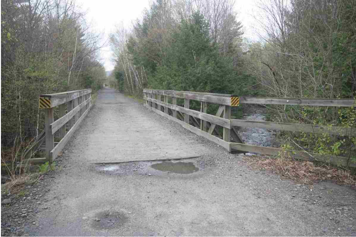
Photo # 111 description: Bridge 148.81, over Moose Brook, Gorham. I-beam stringers on stone (1) and concrete (1) abutments. nd. Stringers replaced 40' span wood pony Howe truss built 1918. (1 of 4).
