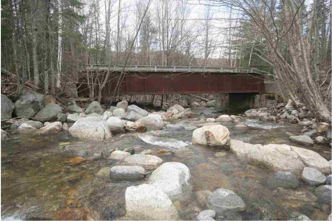
Photo # 61 description: Bridge 142.39 over Cold Brook, Randolph. Upstream side. (2 of 4).
