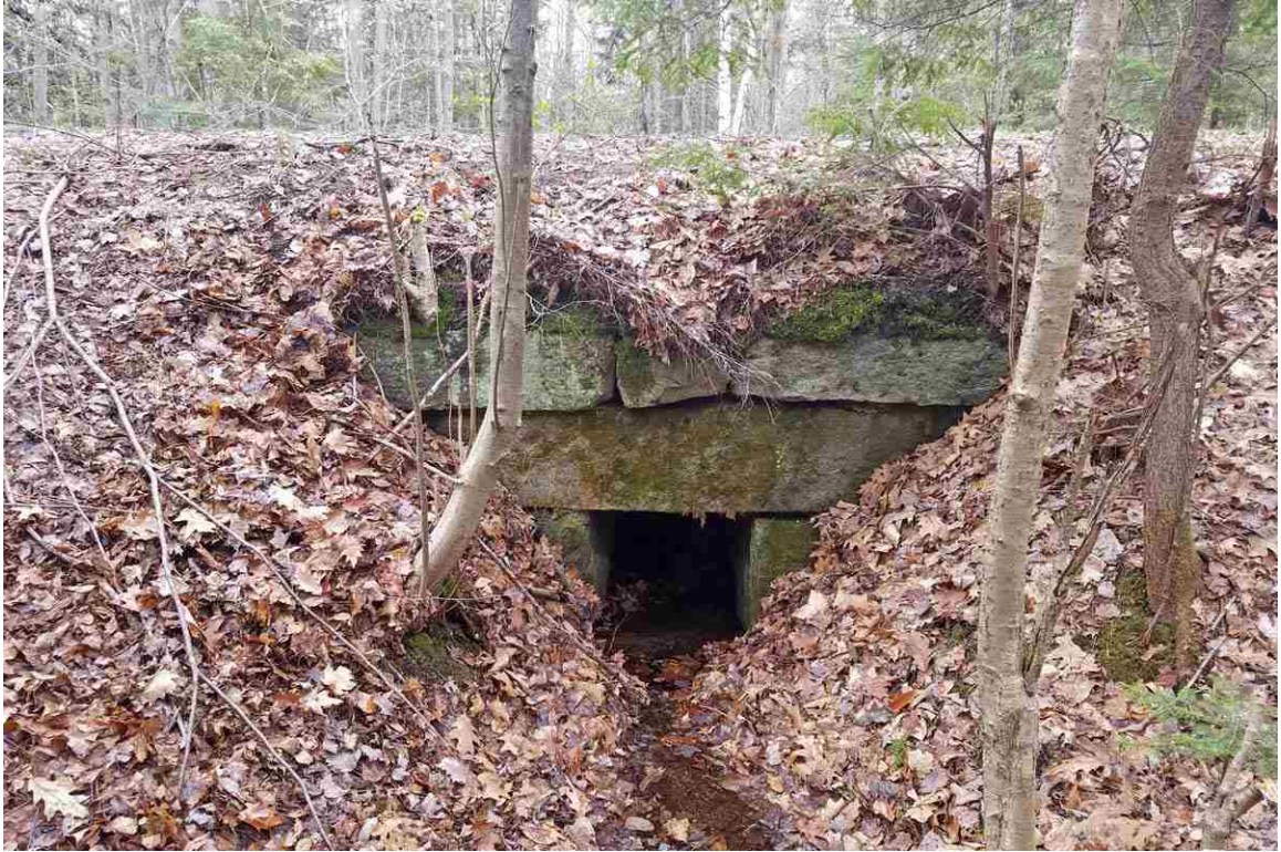
Photo # 109 description: Culvert 147.84, Gorham. Stone box, 36", quarry stone. nd.
