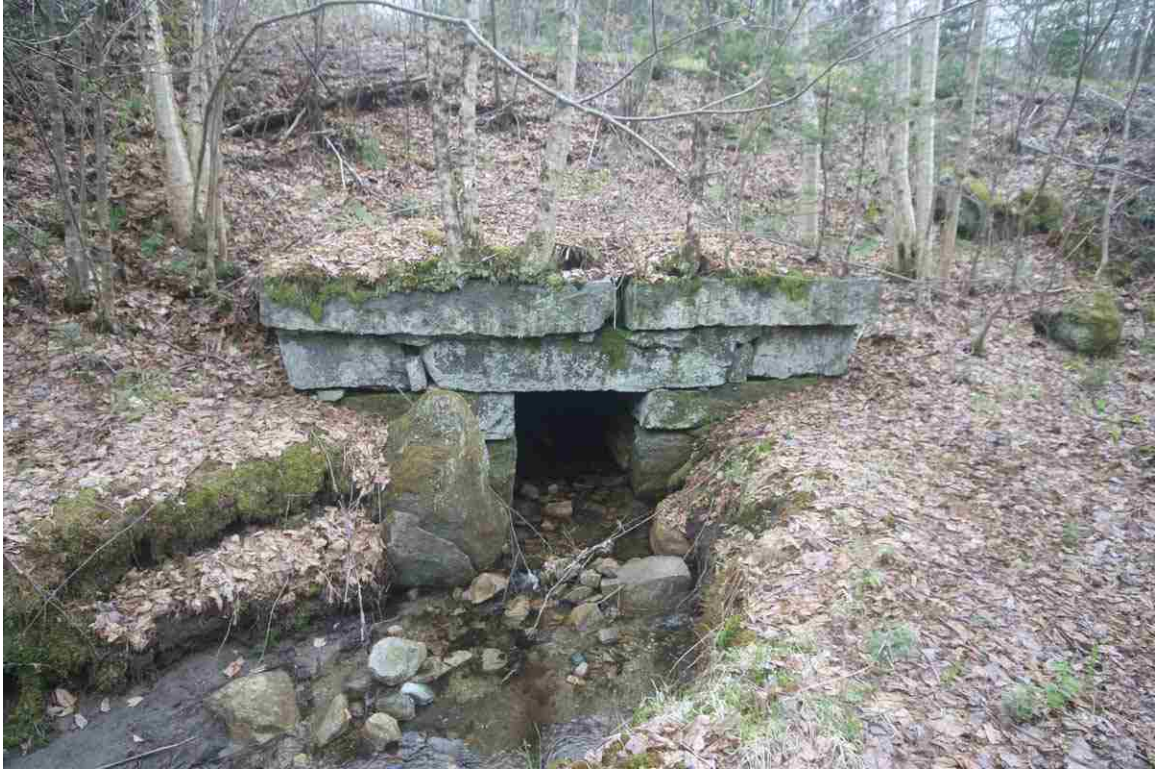
Photo # 39 description: Culvert 138.21, Randolph. Stone box, 30", quarry-split stone. nd.
