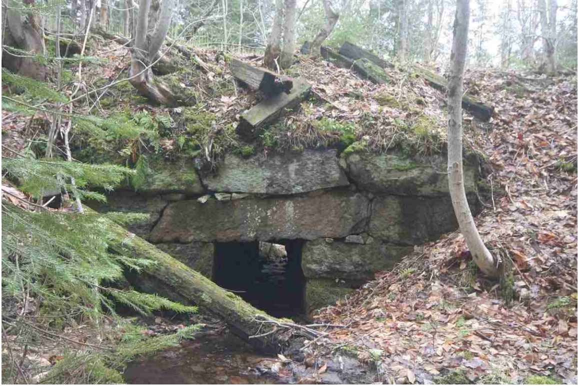
Photo # 107 description: Culvert 147.15, Gorham. Stone box, 36", mixed split quarry & fieldstone. nd.
