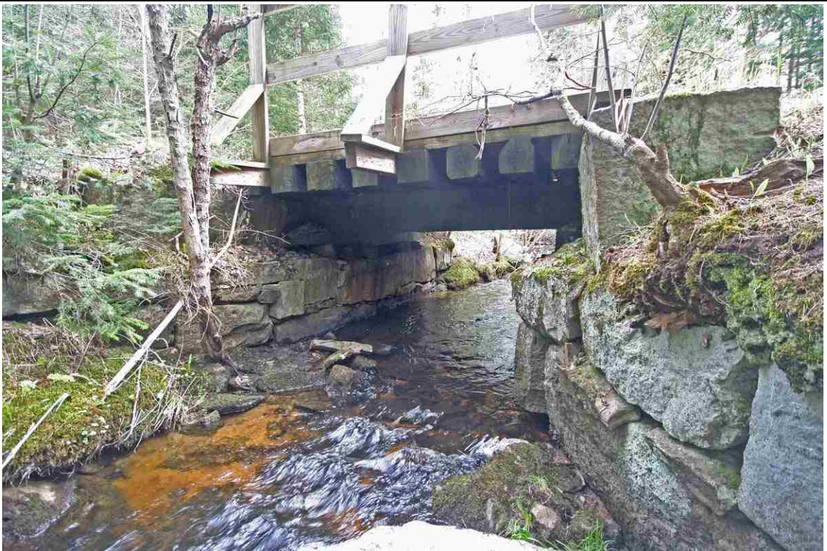
Photo # 18 description: Bridge 133.56 over Red Brook, Jefferson Wood stringer, 8' span. 1926.
