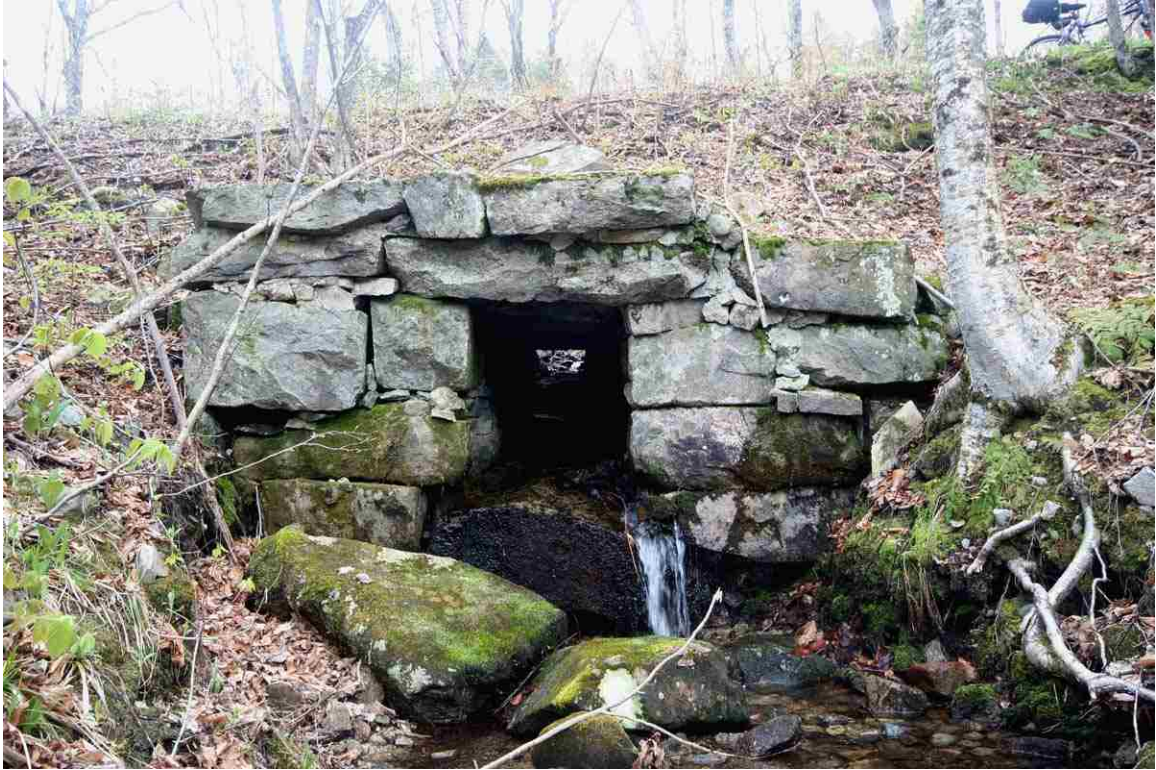
Photo # 53 description: Culvert 141.70, Randolph. Stone box, 36", mixed split quarry & fieldstone. nd.
