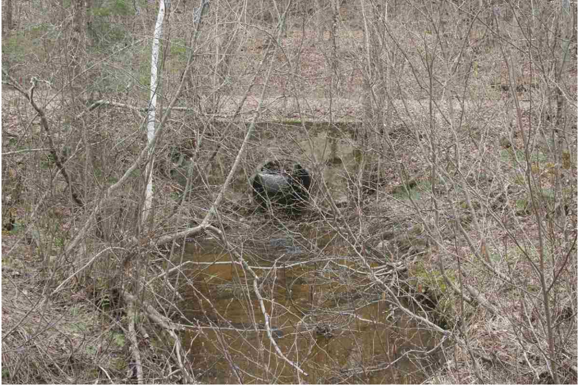
Photo # 29 description: Culvert 135.74, Jefferson. Concrete pipe, 53", concrete headwalls. nd.
