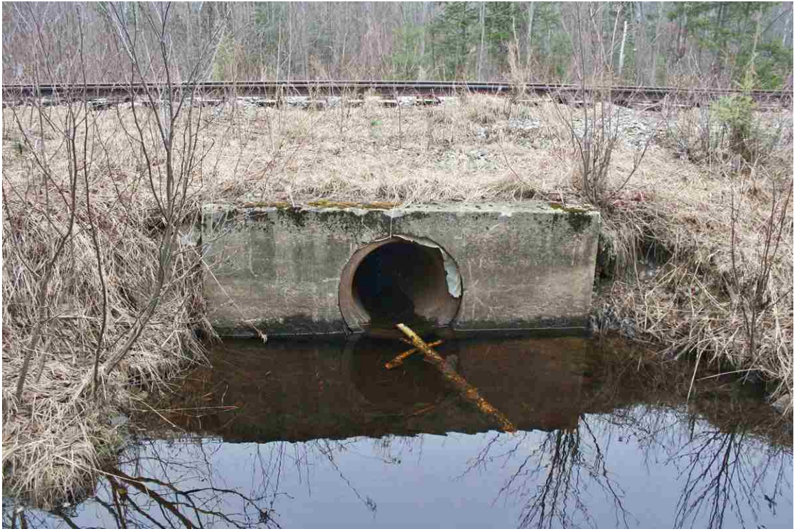
Photo # 7 description: Culvert 129.94, Jefferson. Cast iron pipe, 36"; concrete headwalls. 1929.
