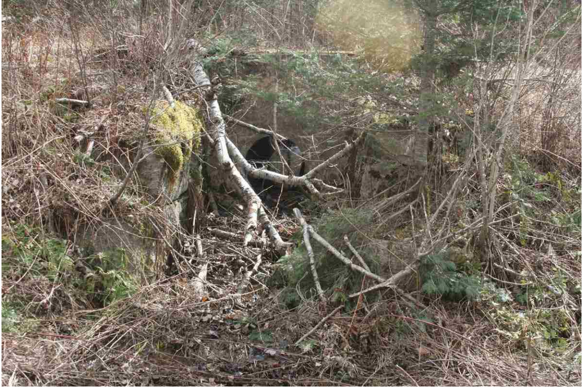
Photo # 35 description: Culvert 137.68, Jefferson. Concrete pipe, 24", with concrete head walls. 1931.
