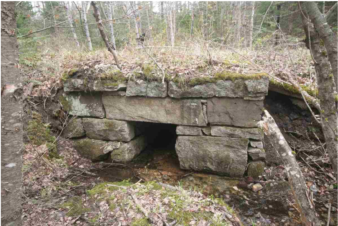
Photo # 82 description: Culvert 144.96, Randolph. Stone box, 36", mixed split quarry & fieldstone. nd.
