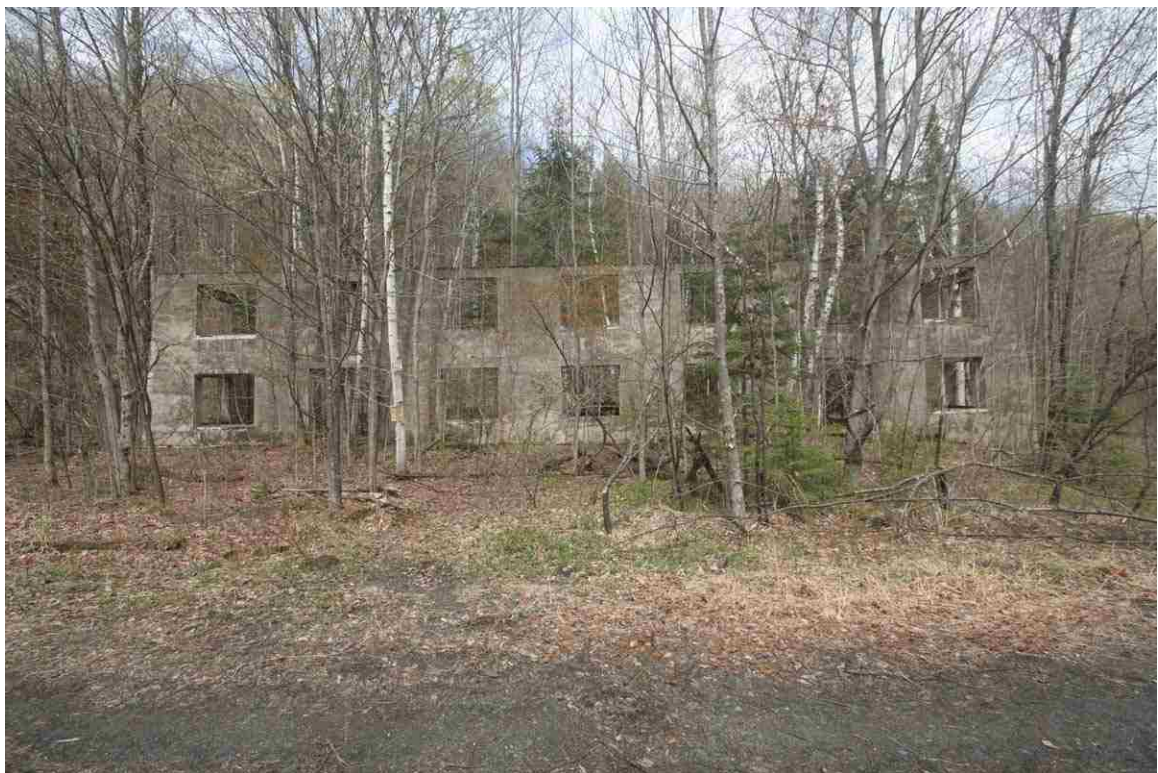
Photo # 96 description: Spring Water Works building at mp. 145.73 (Moose River Bridge No. 2). Reinforced concrete walls; roof gone. nd.
