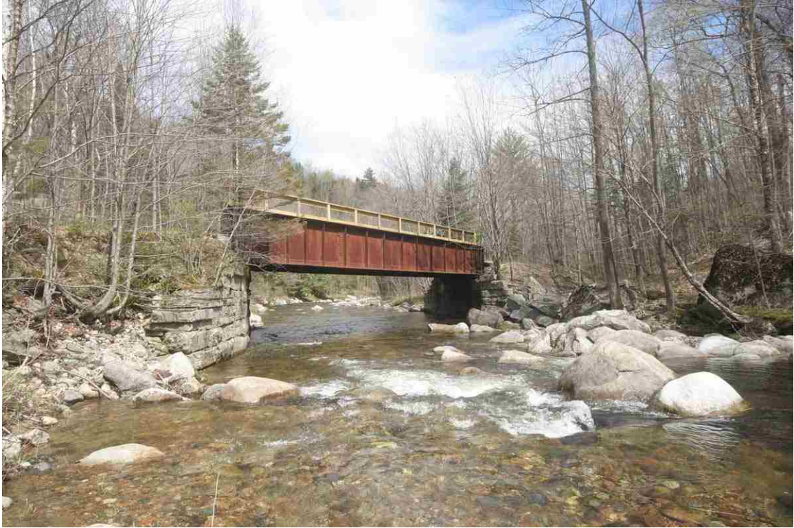
Photo # 93 description: Bridge 145.73, Gorham, "Moose River Bridge No. 2." Upstream side. (2 of 4).
