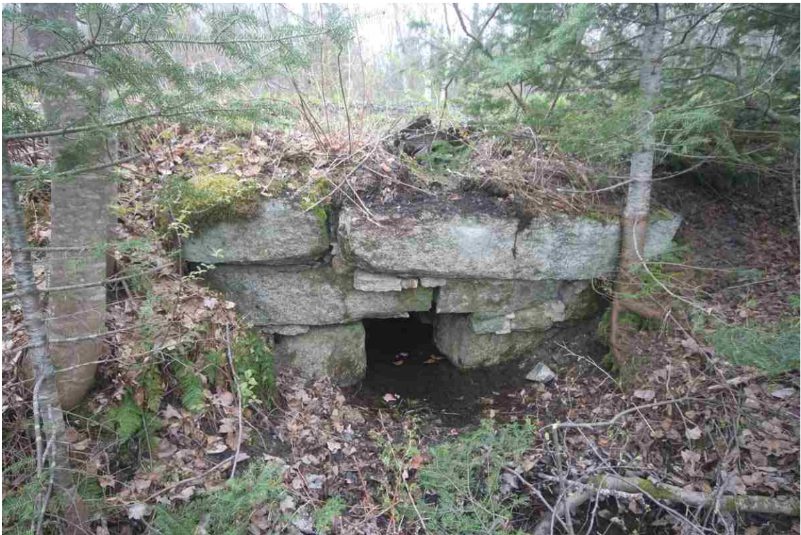
Photo # 38 description: Culvert 138.02, Randolph. Stone box, 30", quarry-split stone. nd.
