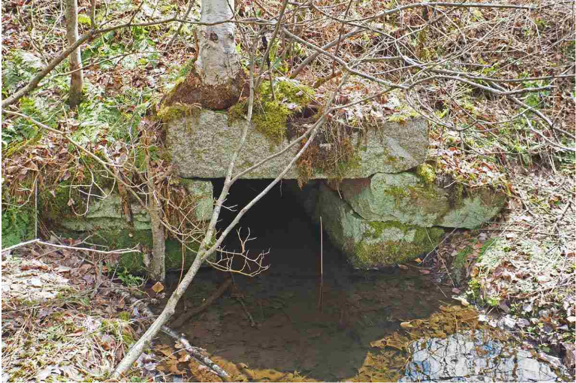
Photo #33 description: Culvert 137.53, Jefferson. Stone box, 60", quarry-split stone. Inlet. 1924. (1 of 2).
