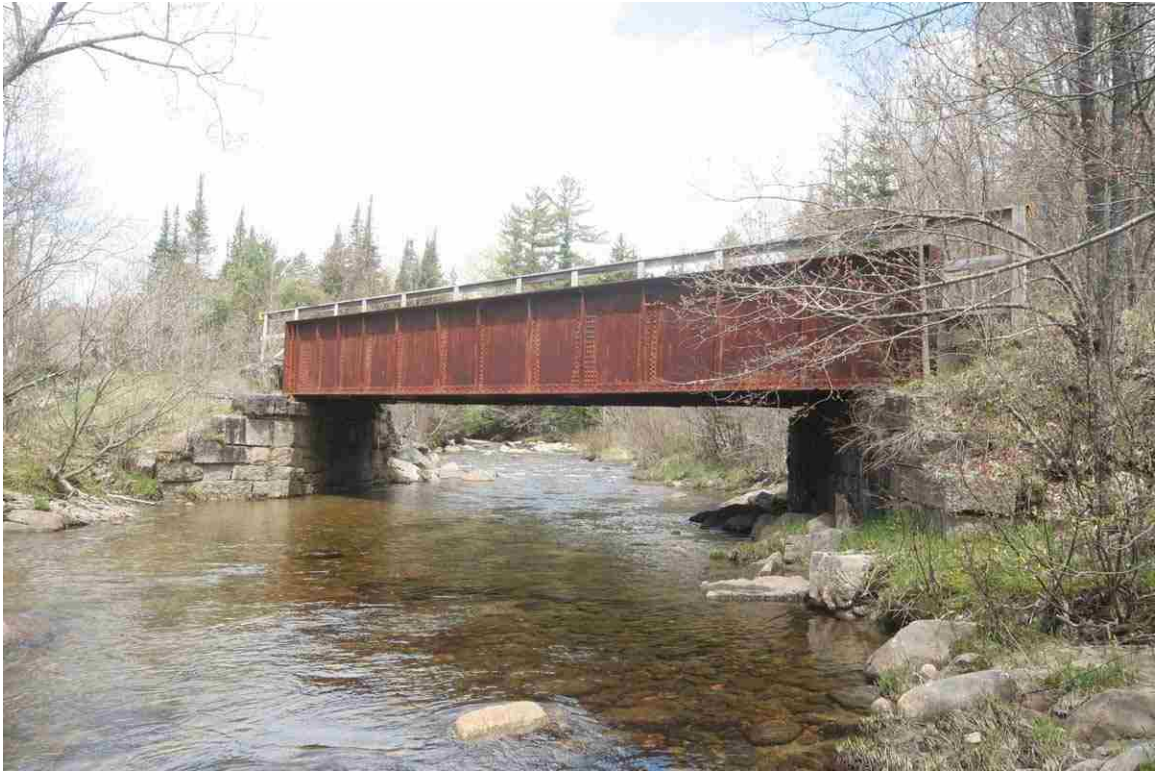
Photo # 87 description: Bridge 145.43, Gorham, "Moose River Bridge No. 1." (2 of 3). Upstream side.
