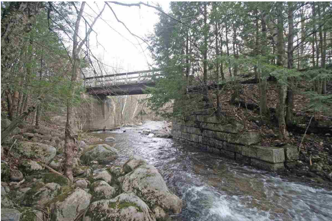
Photo # 112 description: Bridge 148.81, over Moose Brook, Gorham. Upstream side. (2 of 4).
