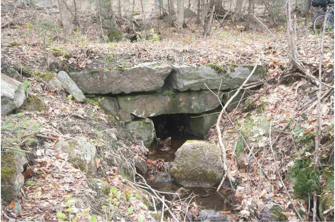
Photo # 55 description: Culvert 142.07, Randolph. Stone box, 30", mixed split quarry & fieldstone. nd.
