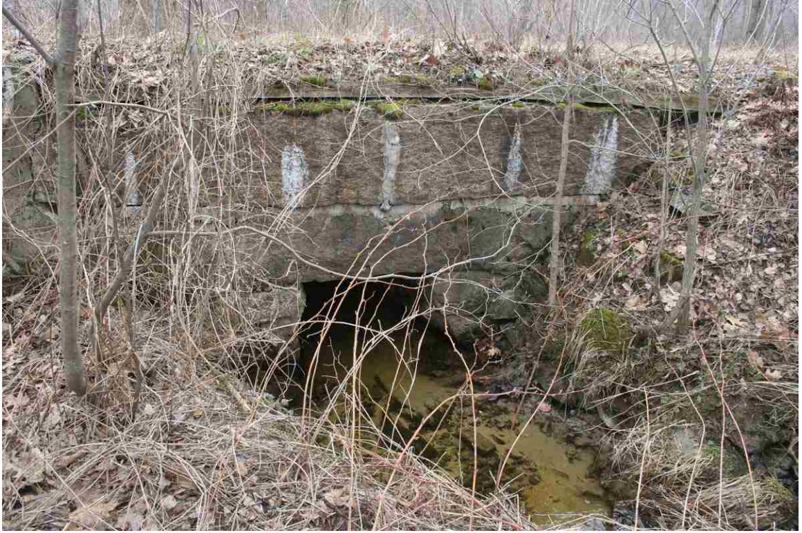
Photo # 27 description: Culvert 135.08, Jefferson. Stone box, 36". (2 of 3).
