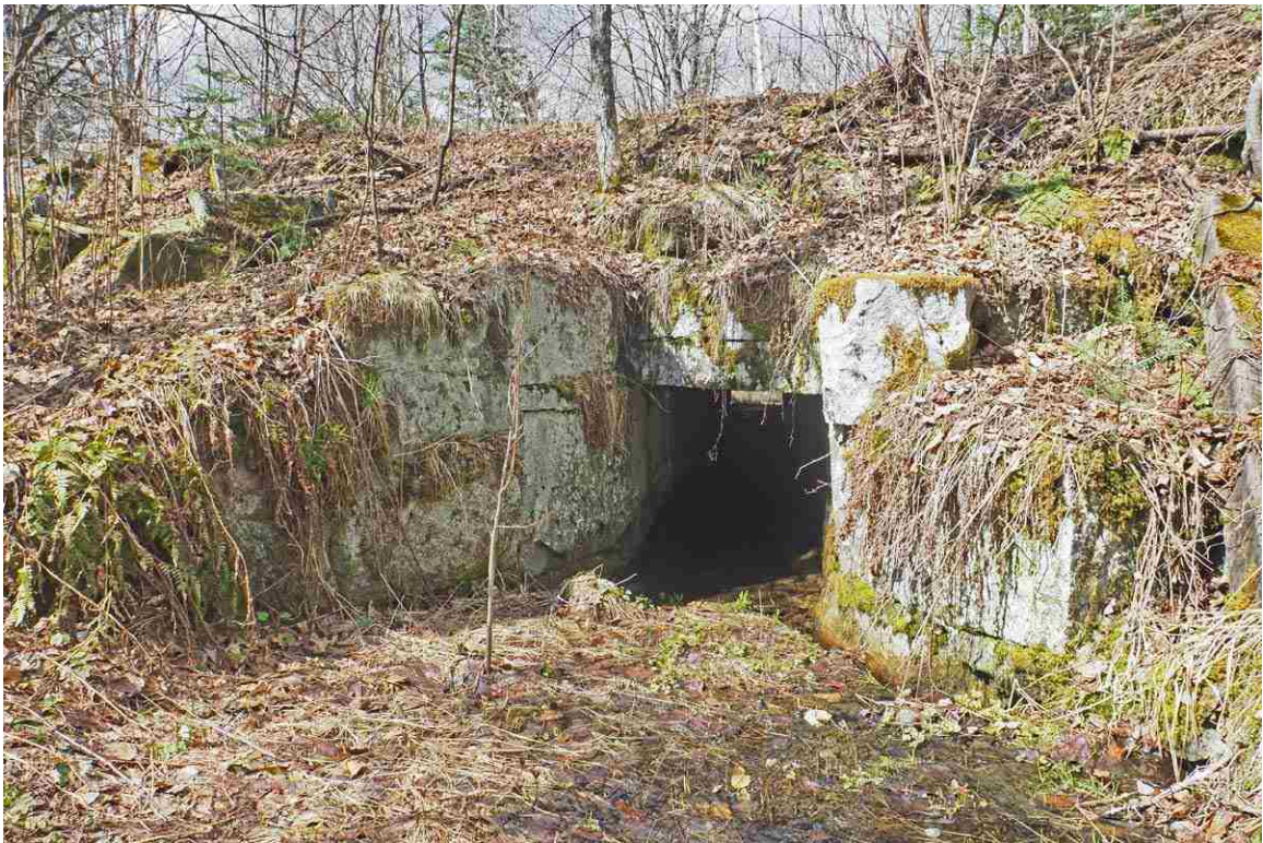
Photo # 34 description: Culvert 137.53, Jefferson. Outlet, showing bevel wing headwall. (2 of 2).
