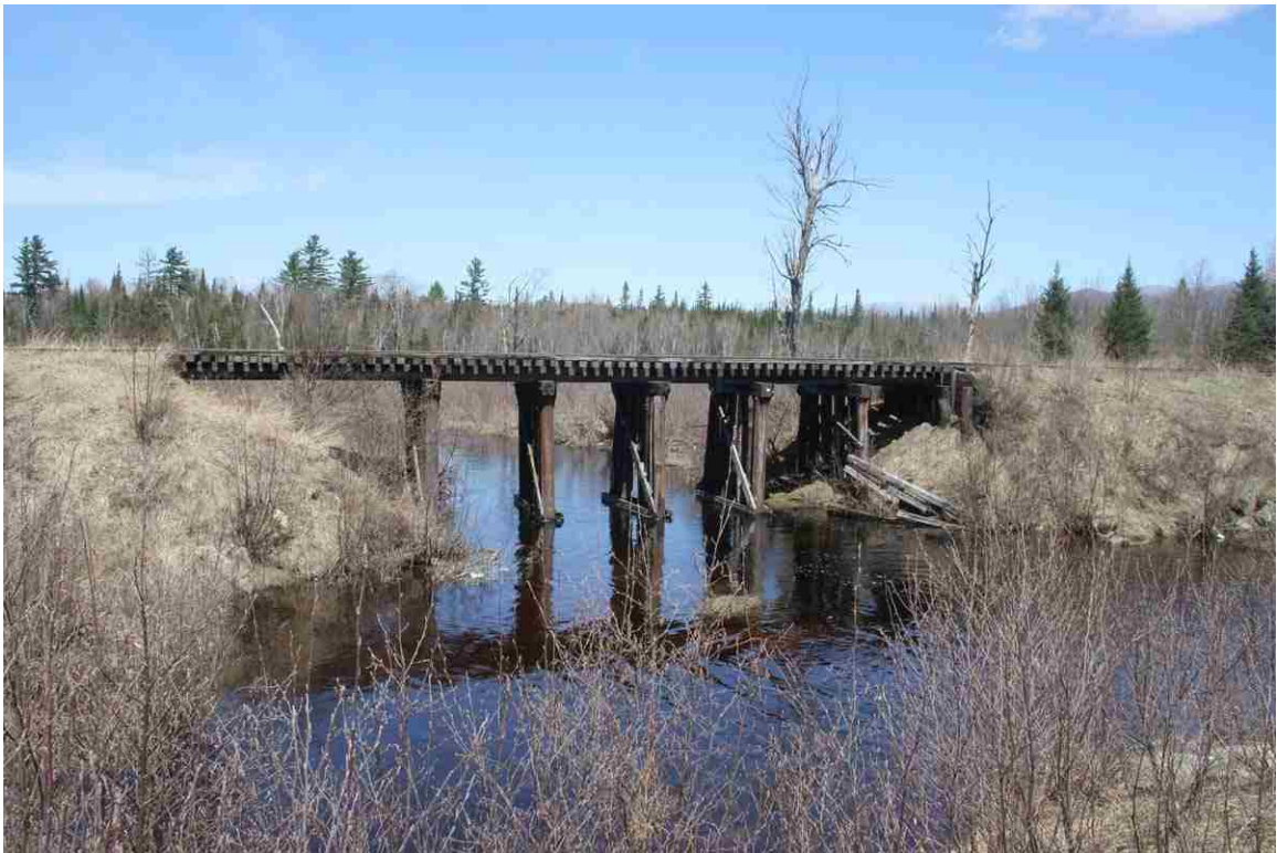
Photo # 4 description: Bridge 128.36 over Carroll Stream, Whitefield. Framed pile trestle, 68', 7-spans. 1926, 1943.
