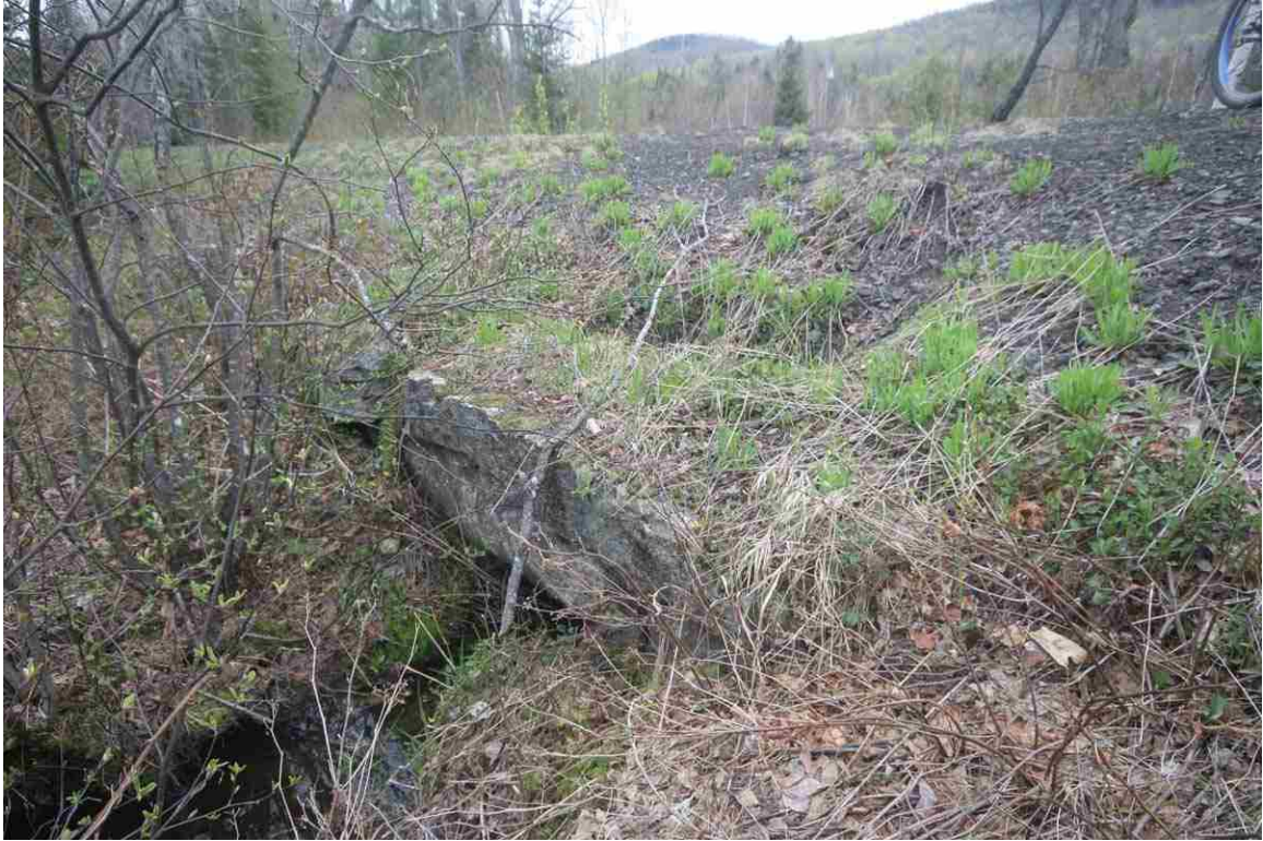
Photo # 37 description: Culvert 137.98, Jefferson. Stone box, 30", field-split stone. nd.
