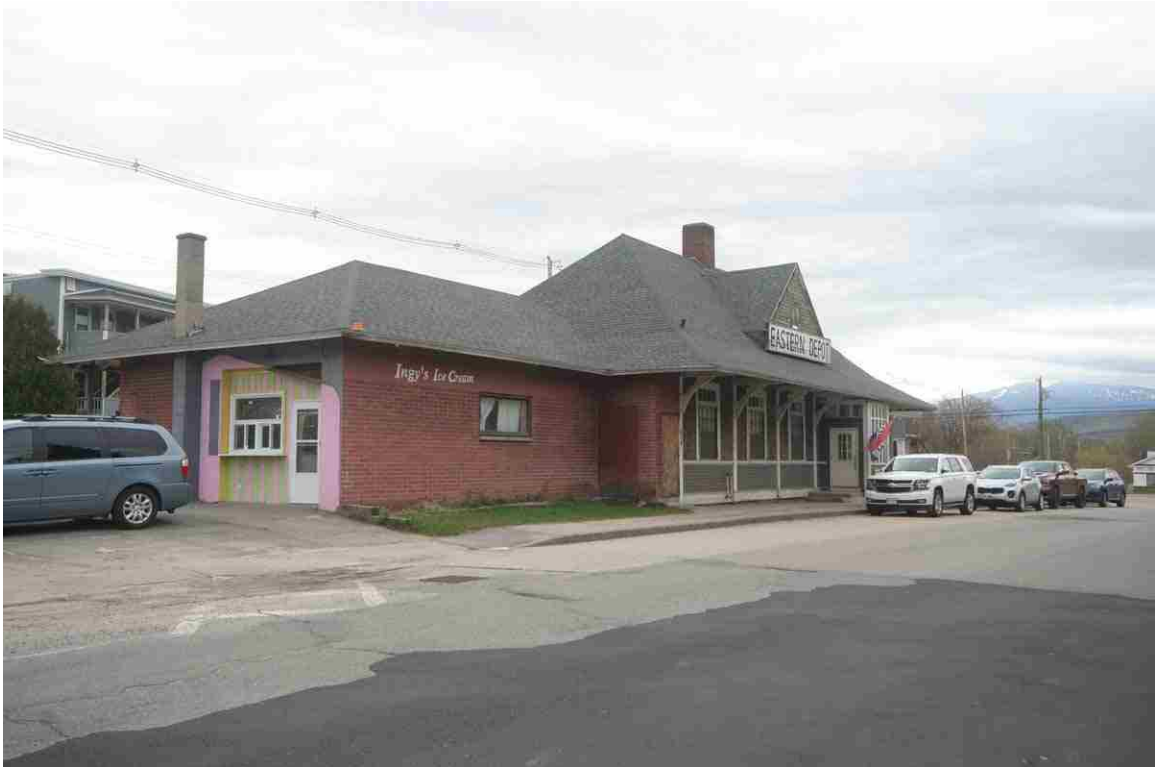
Photo # 134 description: B&M Berlin Station, mp 154.25. Unity Street (west) side. (2 of 2).
