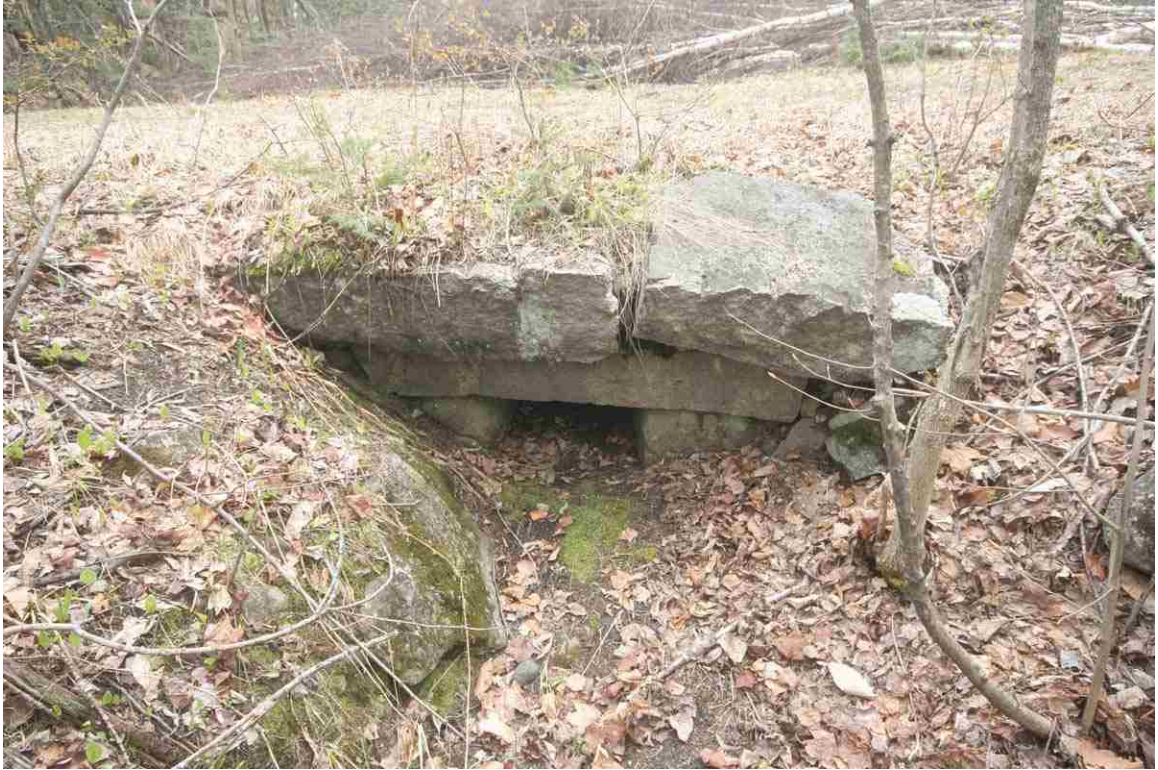
Photo # 65 description: Culvert 142.70, Randolph. Stone box, 36", split quarry stone. nd..
