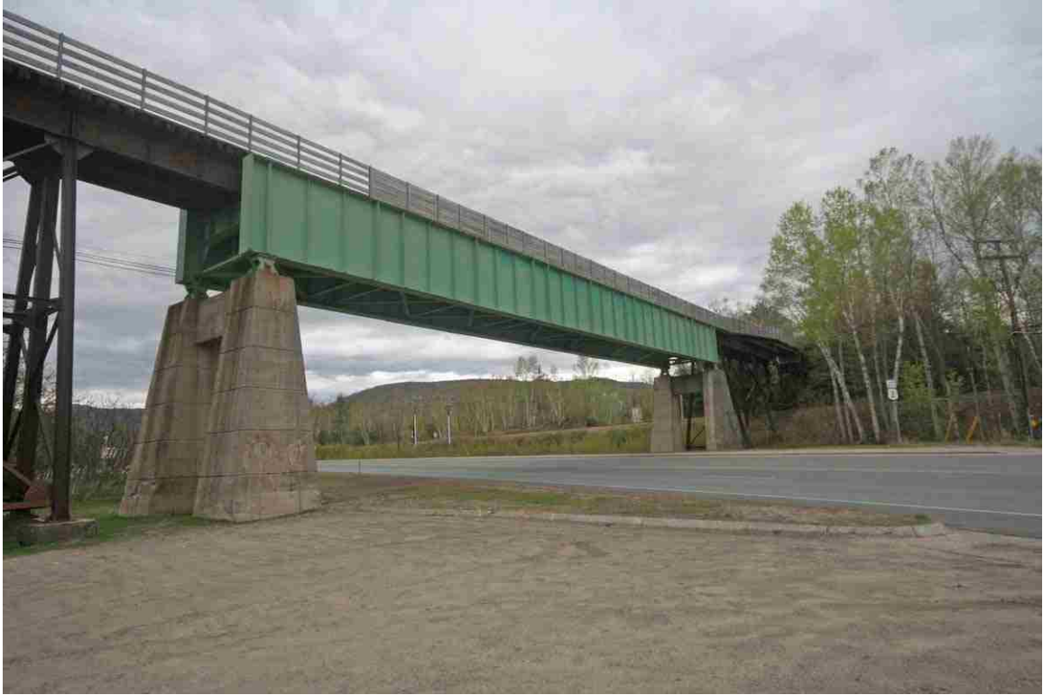
Photo # 117 description: Bridge 149.21, over A&SLRR, NH16, Androscoggin R., Gorham. Deck plate girder span over NH16 highway, carried on concrete piers.
