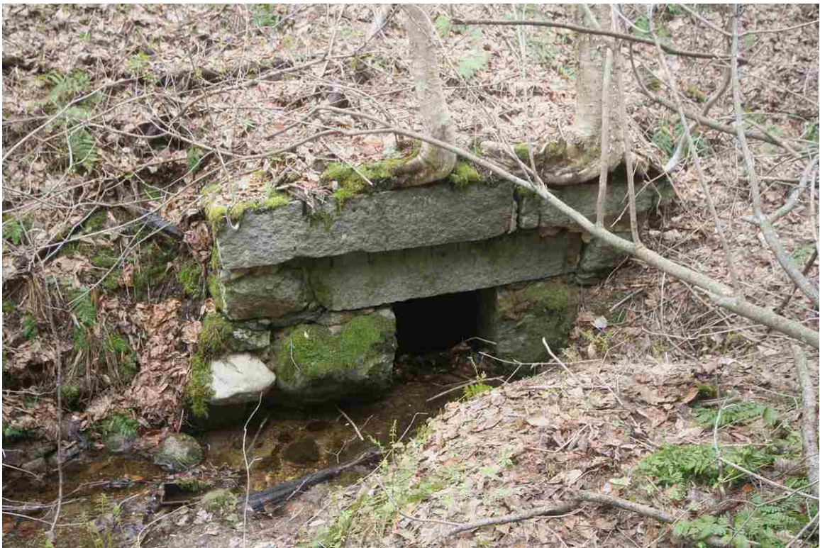
Photo # 100 description: Culvert 146.17, Gorham. Stone box, 30", mixed split quarry & fieldstone. nd.
