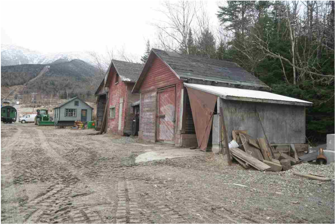
Photo # 101 description: Mt. Washington Cog Railway Base Station, shop buildings. (4 of 6). Cog railway at far left.
