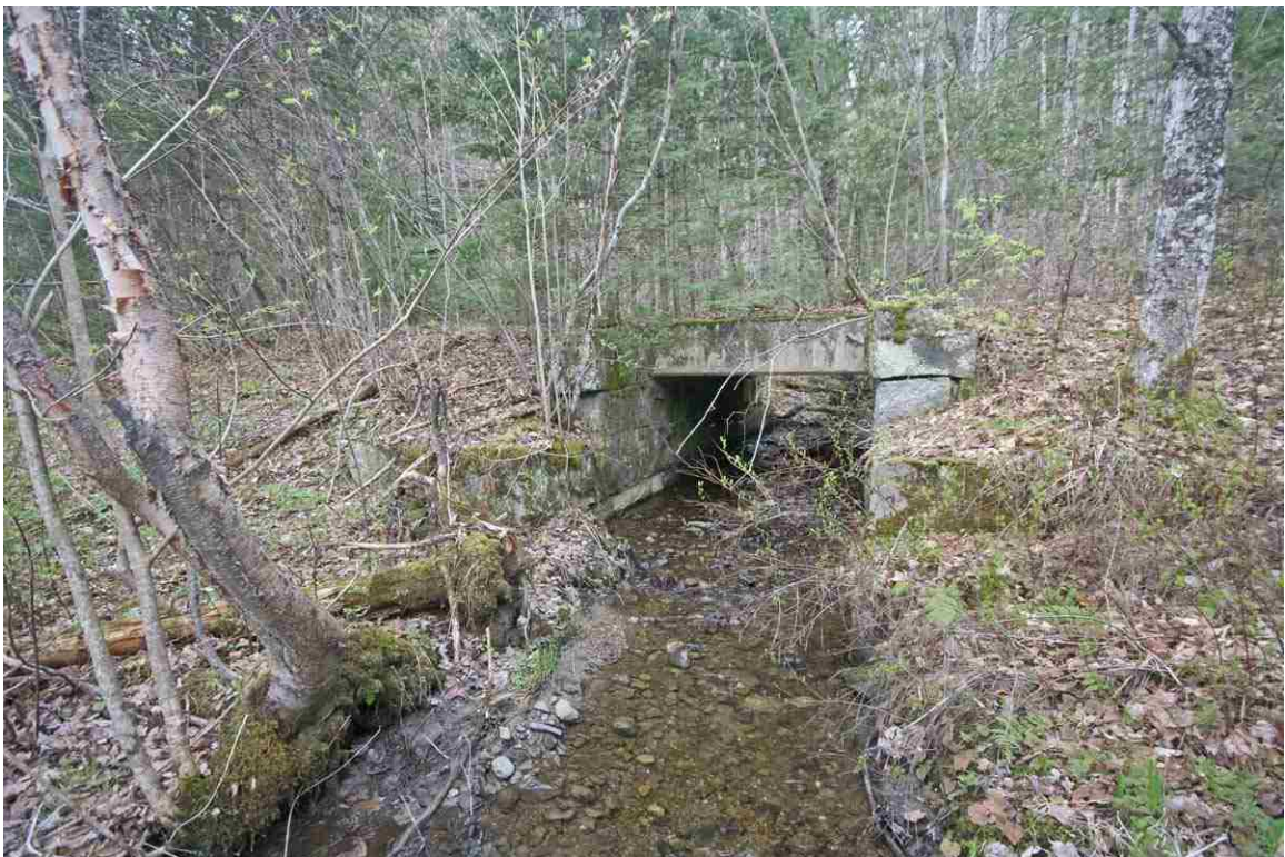
Photo # 30 description: Bridge 126.06, over unnamed stream, Bethlehem. Concrete slab on stone abutments. Downstream side. (2 of 2).
