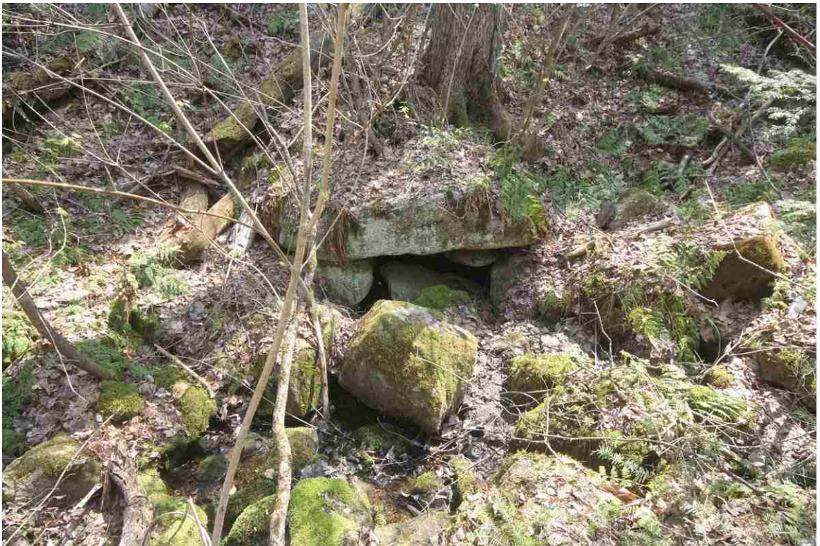
Photo # 16 description: Culvert mp~122.60, Bethlehem. Stone box, ~24". Halfway between McCann Road and Wilderness Road.
