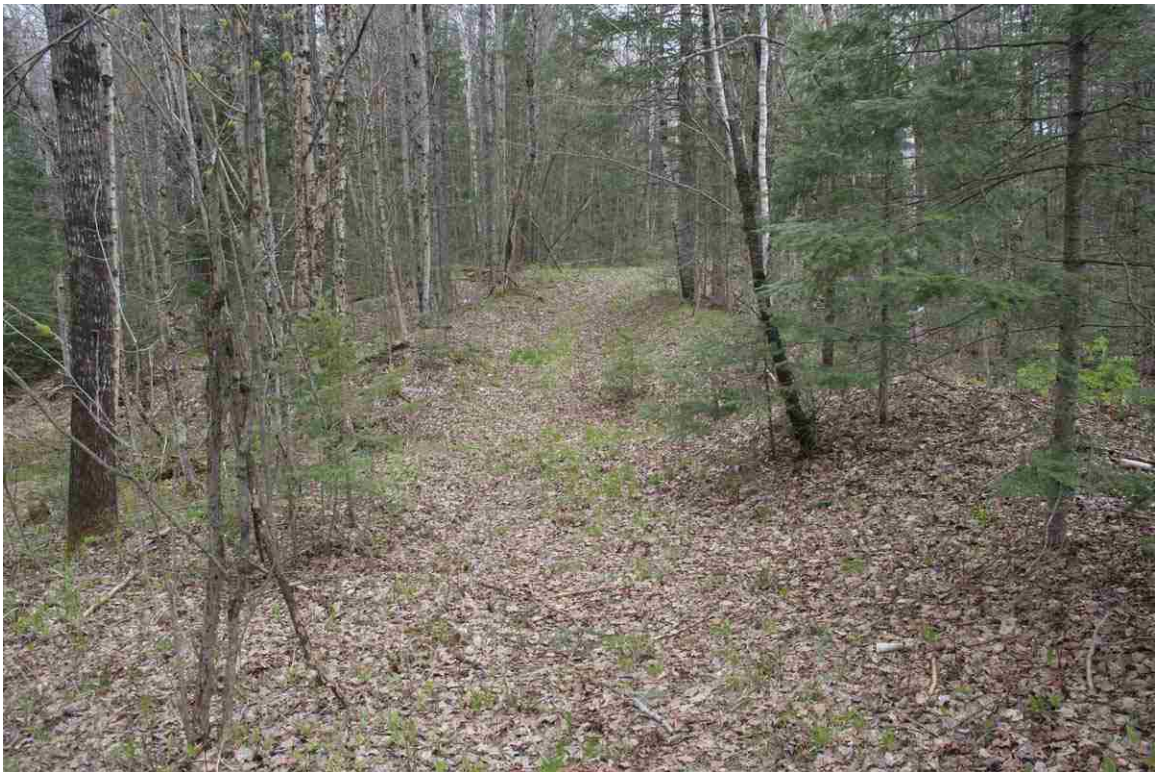
Photo # 24 description: ROW, mp~125.20, Bethlehem. Bed washed out in places.
