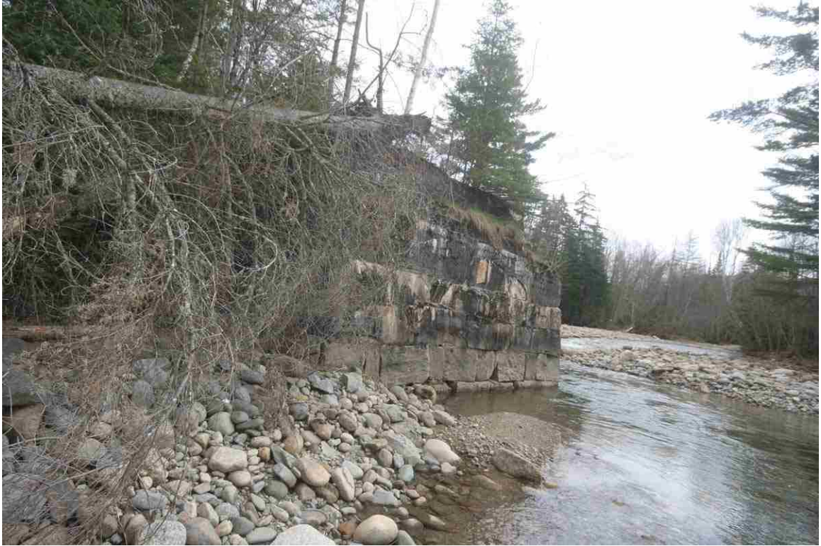
Photo # 37 description: Little River Bridge, Carroll. East abutment, north side. (2 of 4).
