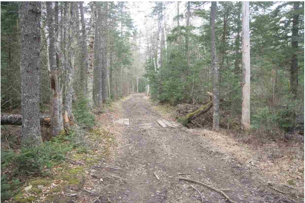
Photo # 84 description: Condition of ROW, maintained as trail. New plank span possibly replaced pipe culvert, vicinity of mp~136.02, Crawfords Purchase.
