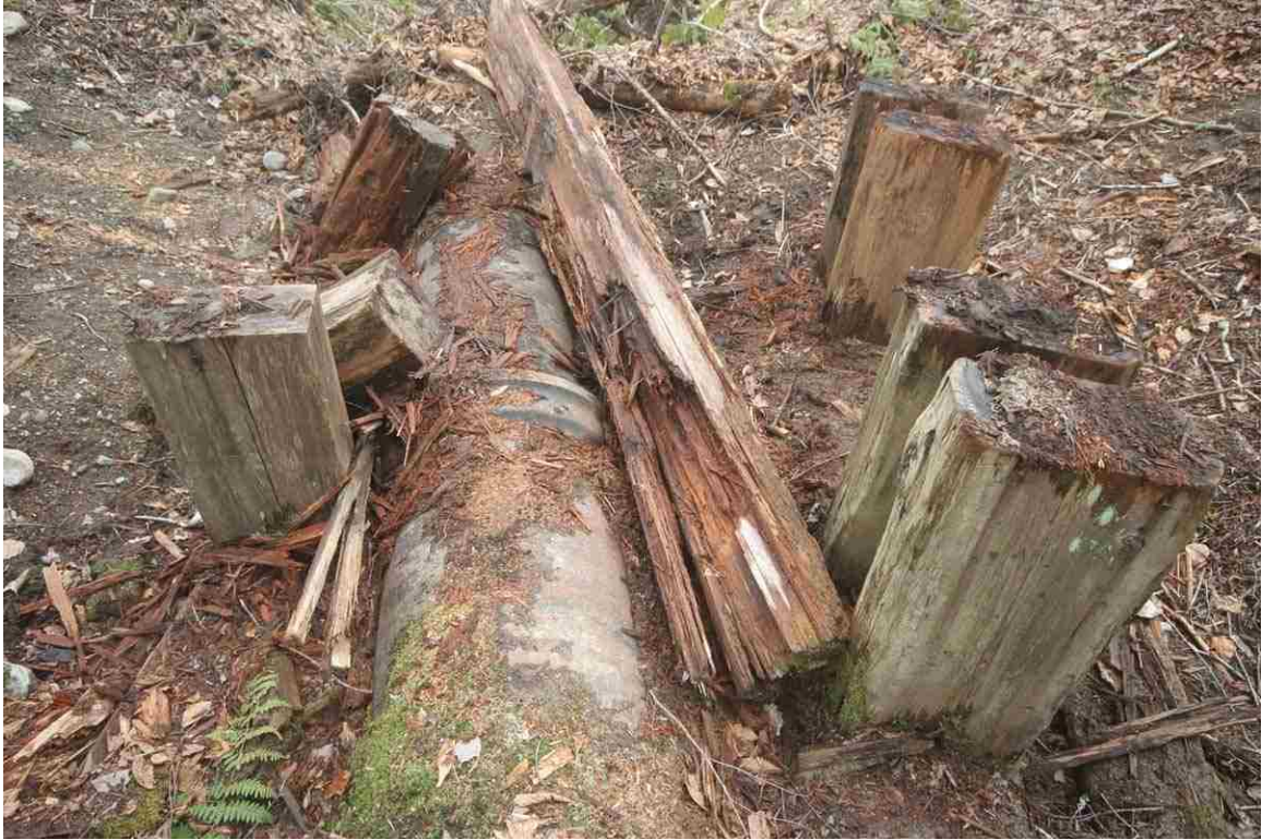
Photo # 89 description: Culvert 138.23, Crawfords Purchase. Detail of pipe placement between timber piles to prevent lateral movement of the pipe.
