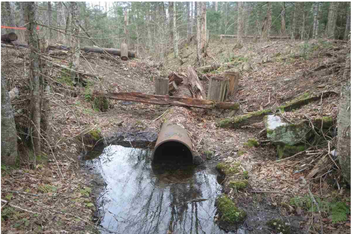
Photo # 88 description: Culvert 138.23, Crawfords Purchase. Detail of outlet end. (2 of 3).
