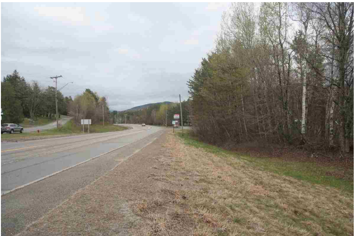
Photo # 58 description: Remnant of ROW railbed, mp~129.85. Opposite view of Photo 57. ROW railbed remnant at right merges into US302, reappears on north side of highway about 1 mile east.
