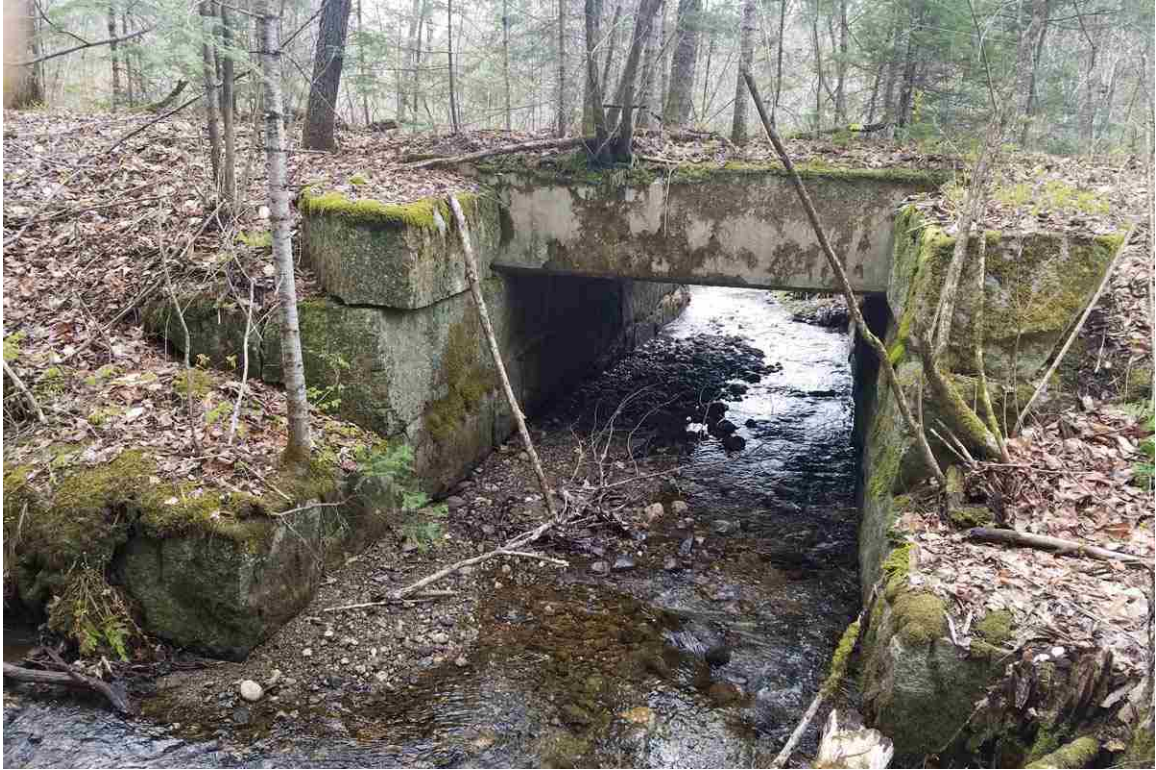
Photo # 29 description: Bridge 126.06 over unnamed stream, Bethlehem. Concrete slab on stone abutments. ~10' span. nd. Upstream side. (1 of 2).
