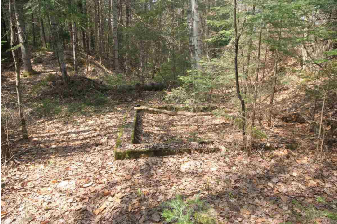
Photo # 11 description: Abandoned ROW. mp~121.36, Bethlehem. Concrete foundation alongside ROW.
