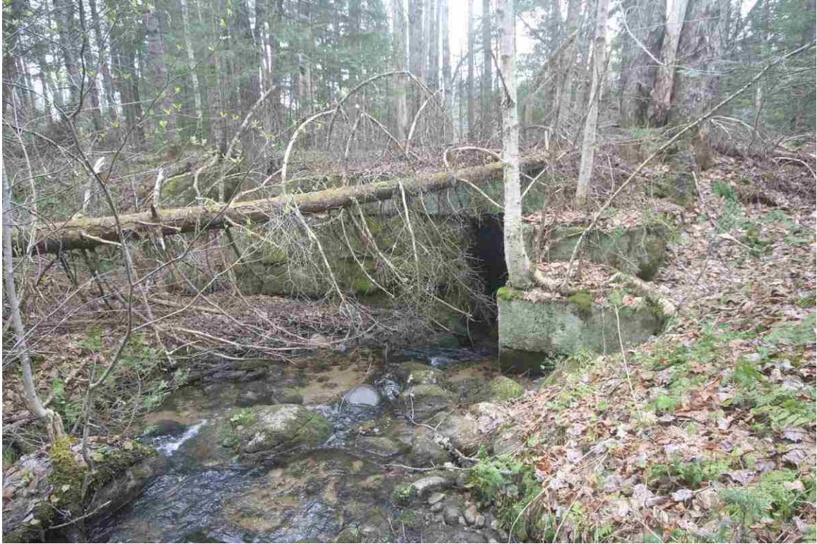
Photo # 33 description: Culvert 126.50, Bethlehem. Downstream side. (2 of 2).
