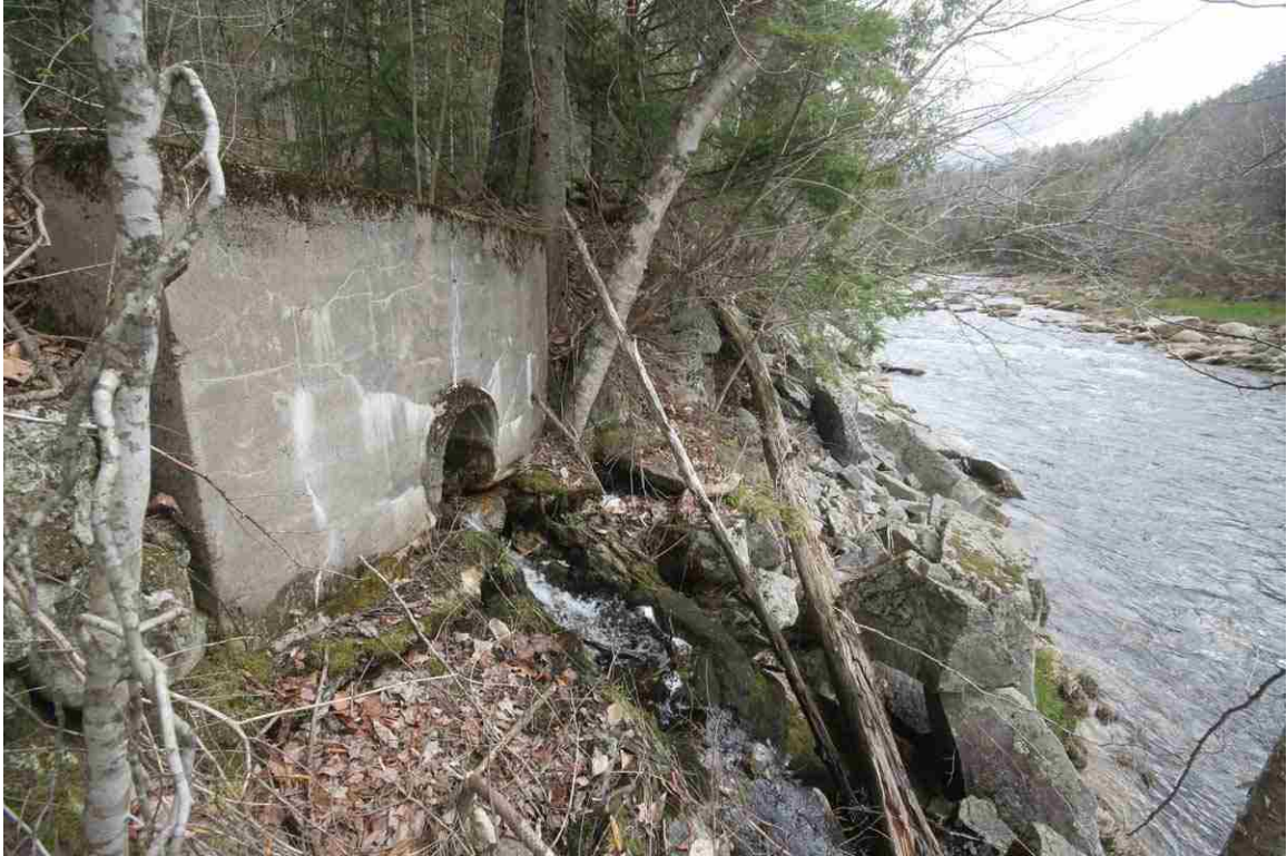
Photo # 27 description: Culvert 125.50, Bethlehem. Akron pipe, 18", in concrete headwalls. Outlet at edge of Ammonoosuc R. (2 of 2).
