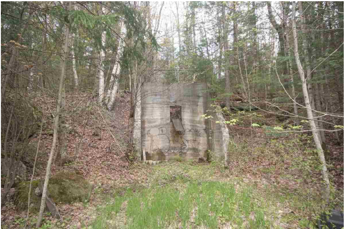
Photo # 4 description: Concrete buttressed wall against ROW along Wing Road, Bethlehem; mp~121.14. Metal chute suggests purpose was for offloading coal or other bulk material into a truck. (1 of 3)
