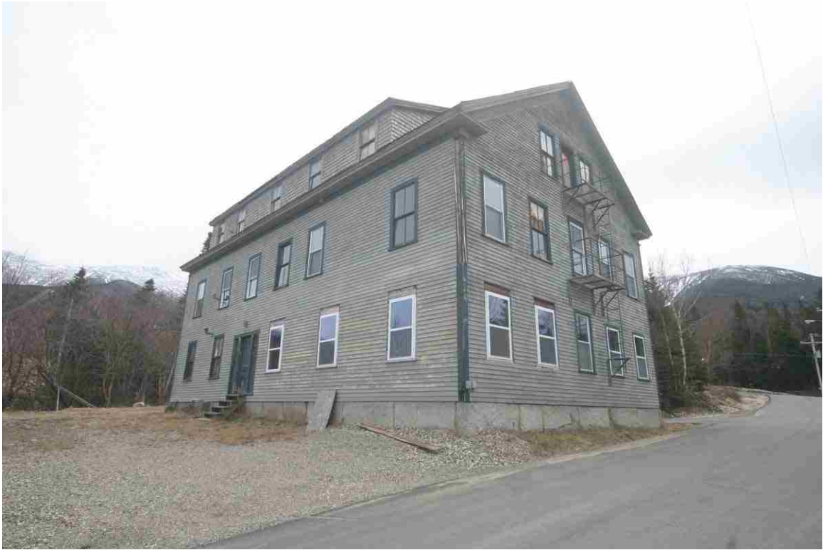
Photo # 97 description: Mt. Washington Cog Railway Base Station, housing building. North and west side. (2 of 2).
