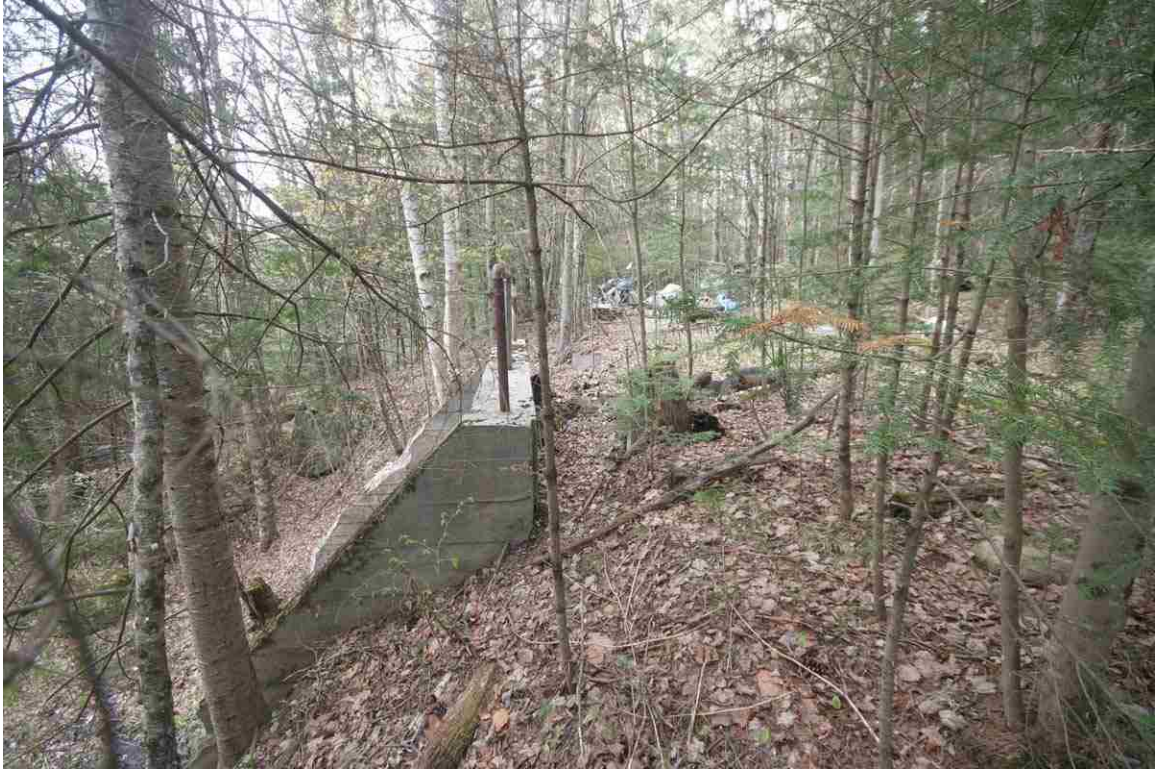
Photo # 5 description: Concrete buttressed wall with chute, (2 of 3). View of overgrown ROW at right.
