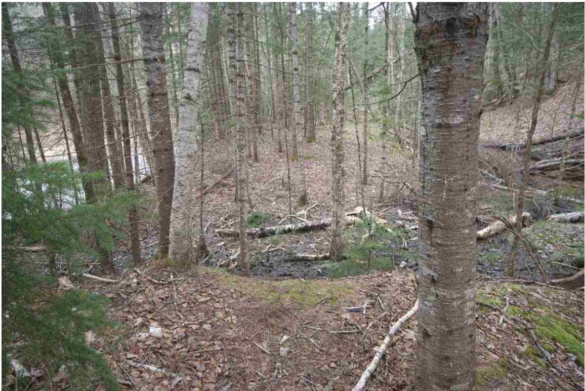
Photo # 28 description: ROW, mp 125.74, Bethlehem. Location of 30" cast iron pipe culvert completely washed out leaving deep gully in ROW.
