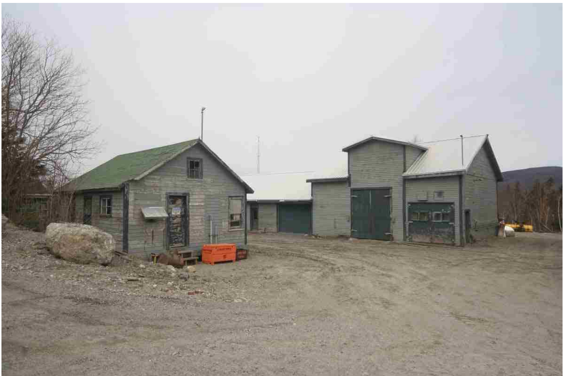
Photo # 98 description: Mt. Washington Cog Railway Base Station, shop buildings. Included for documentation purposes and association with the Mt. Washington Branch. (1 of 6).
