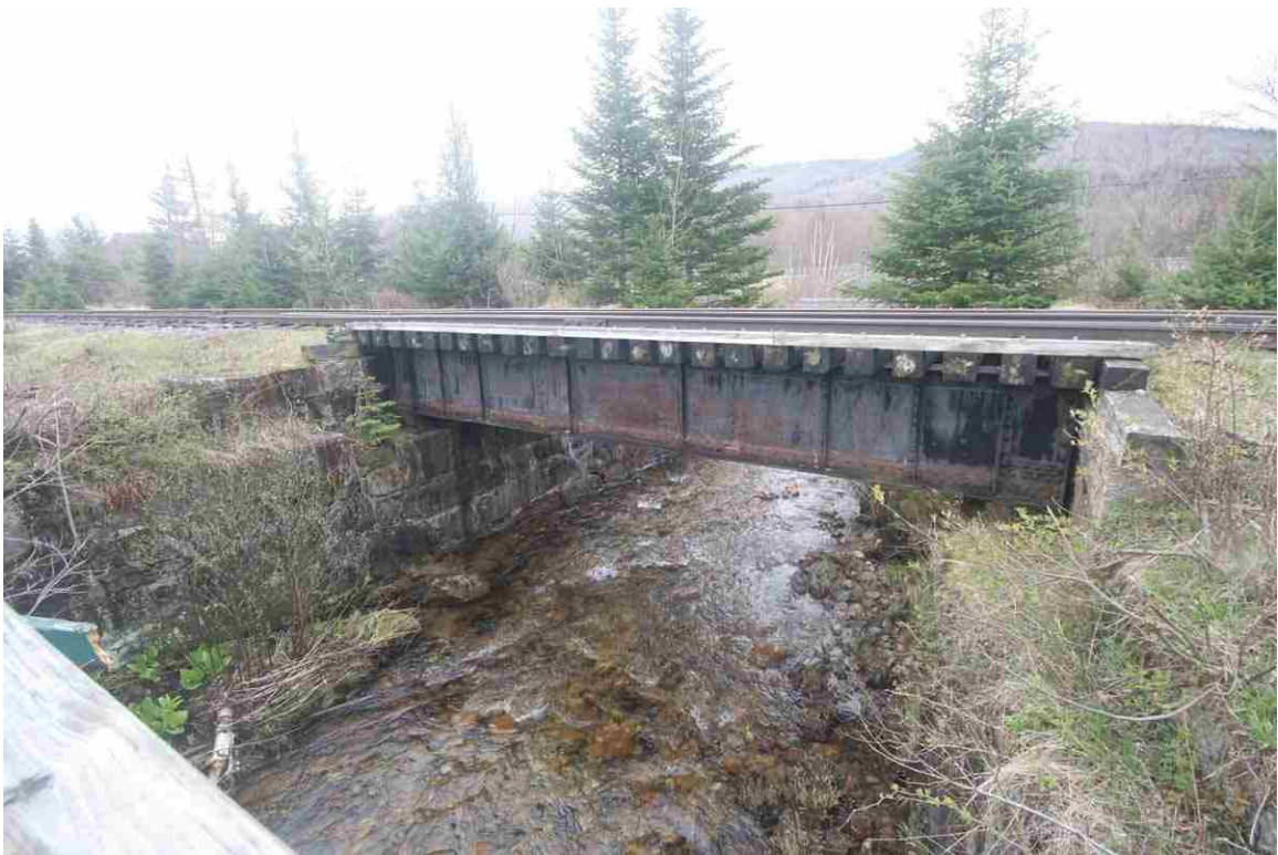
Photo # 68 description: Former MC Cherry Mtn. Brook bridge, north side. BC&M bridge was on the south side. The tracks ran side by side in this area. (2 of 3).
