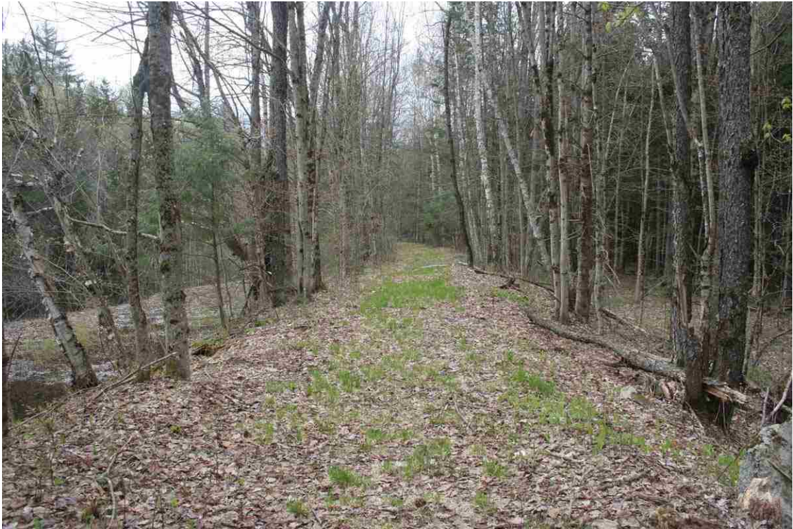
Photo # 23 description: Abandoned ROW, mp~125.15, Bethlehem. Raised bed with numerous deep washouts evidently locations of culverts. ~ 2000' east of Pierce Bridge.
