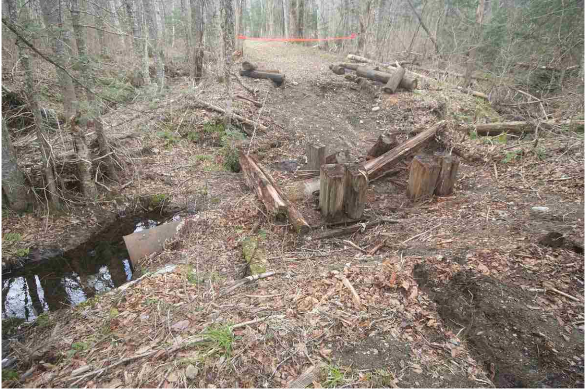
Photo # 87 description: Culvert 138.23, Crawfords Purchase. 24" cast iron pipe on timber frame. Note reliving piles that carried stringer span over solid fill. Washed out. nd. (1 of 3).
