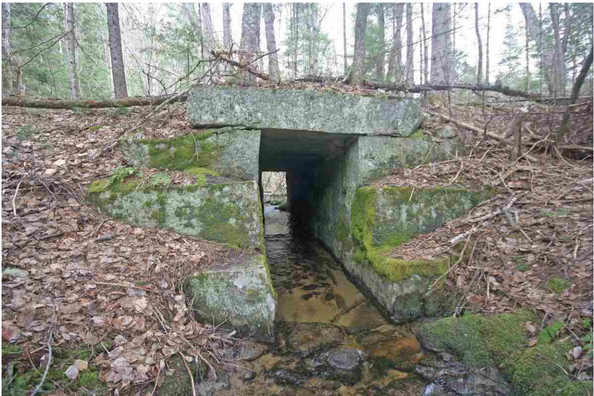
Photo # 32 description: Culvert 126.50, Bethlehem. Stone box, 48" x 60" high, quarry split. Upstream side. (1 of 2).
