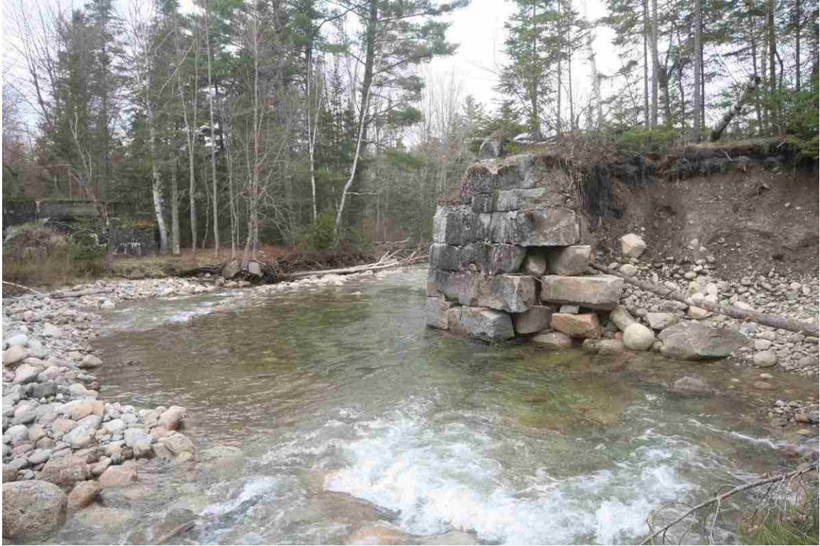
Photo # 39 description: Little River Bridge, Carroll. East abutment, detail of south side; west abutment visible at left. (4 of 4).
