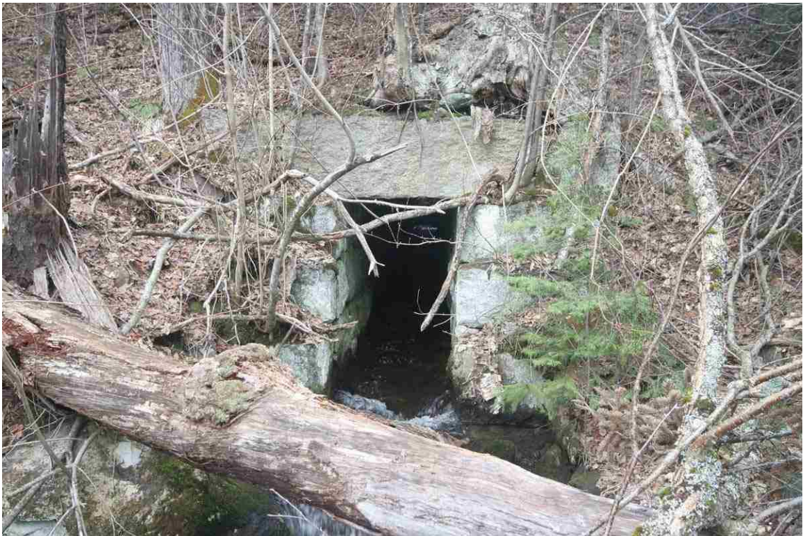
Photo # 60 description: Culvert 133.07, Carroll. Stone box, 6' x 8'. Impressive size with deep cover, in good condition. nd.
