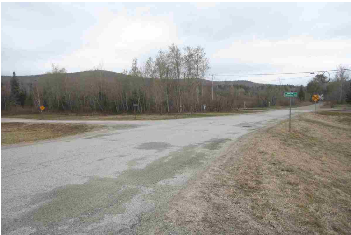
Photo # 66 description: Former ROW crossing Old Cherry Mountain Road, Carroll, on south side of MC crossing, visible in distance. mp~133.71.
