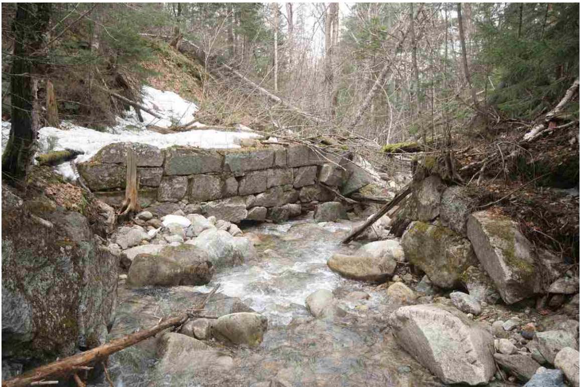
Photo # 94 description: Location of frame trestle bridge over Franklin Brook, Crawfords Purchase, mp~140.76, 400' east of Cog Railway shops. West stone abutment carried frame bent. (1 of 2).
