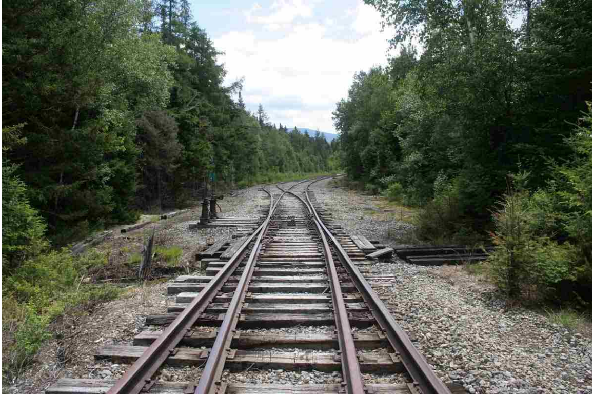
Photo # 75 description: Switch, mp 134.02 and cattle pass. (2 of 2).
