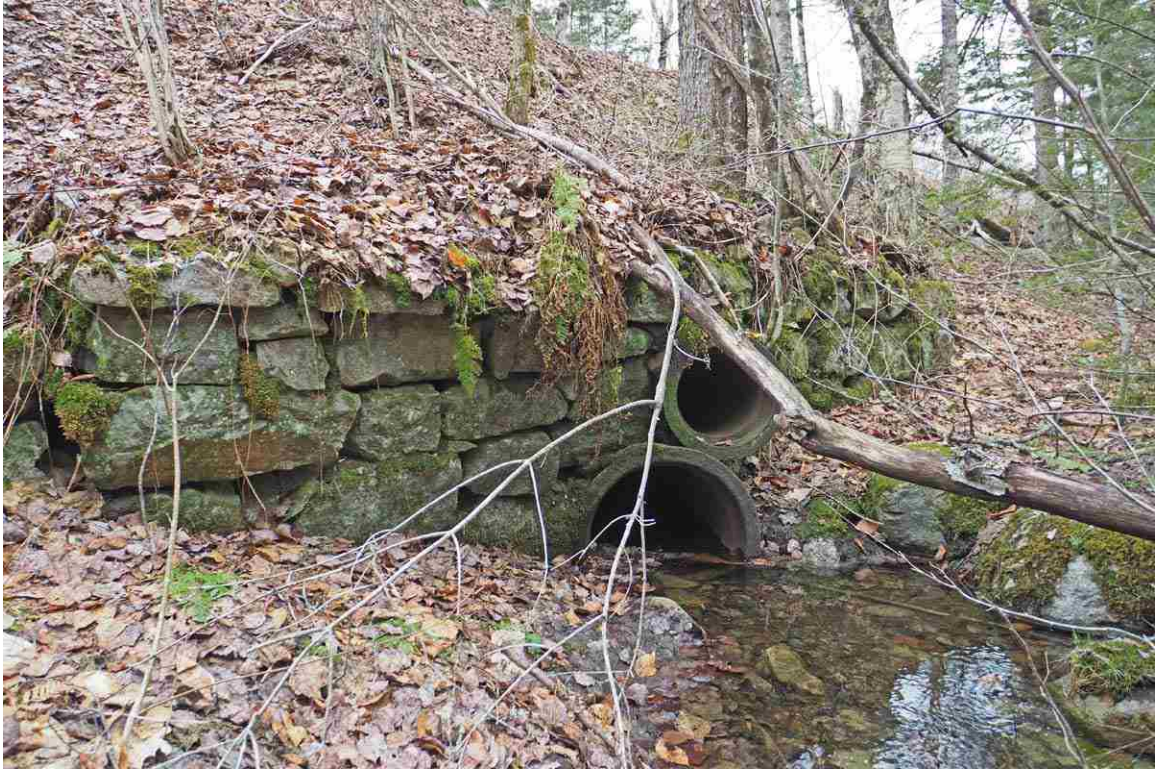
Photo # 59 description: Culvert 132.55, Carroll. Former stone box fitted with 2 pipes. nd.
