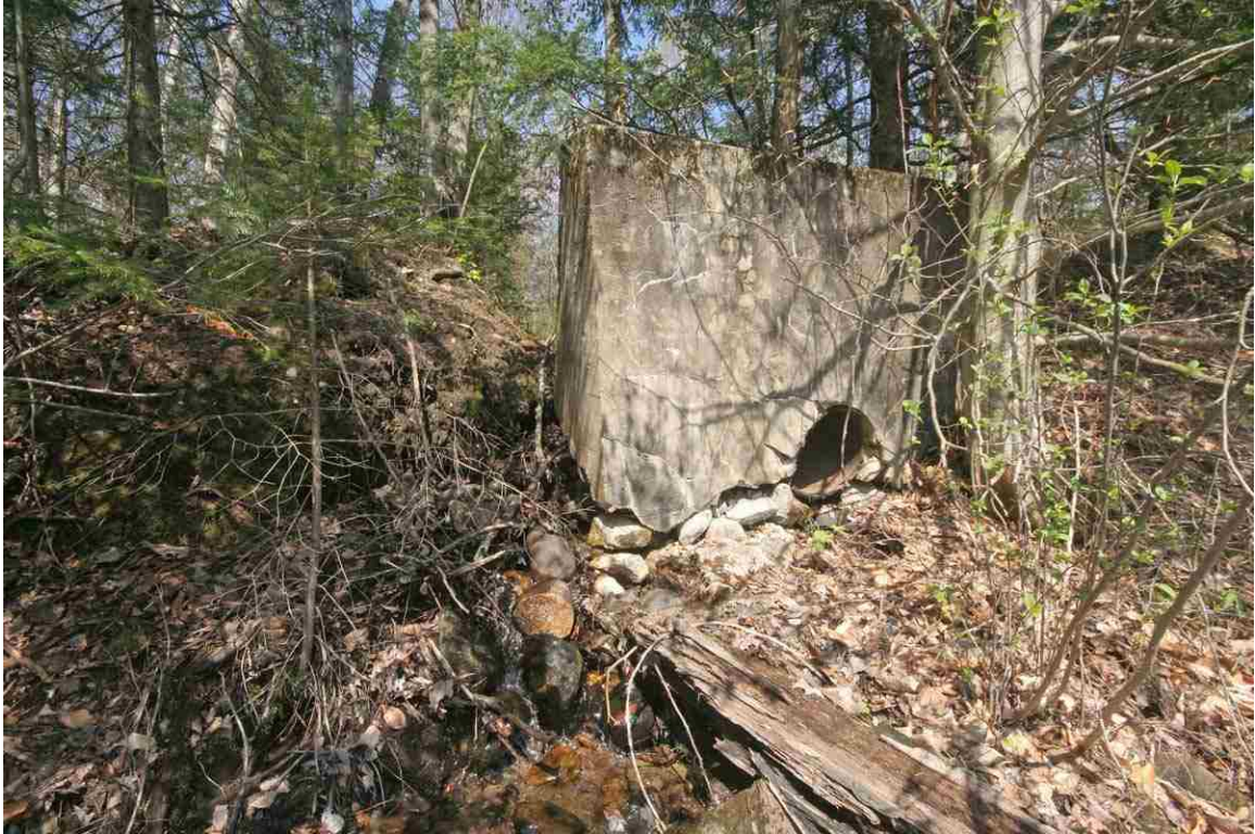
Photo # 19 description: Culvert mp~123.60, Bethlehem. (2 of 2). Concrete headwall at edge of Ammonoosuc R.
