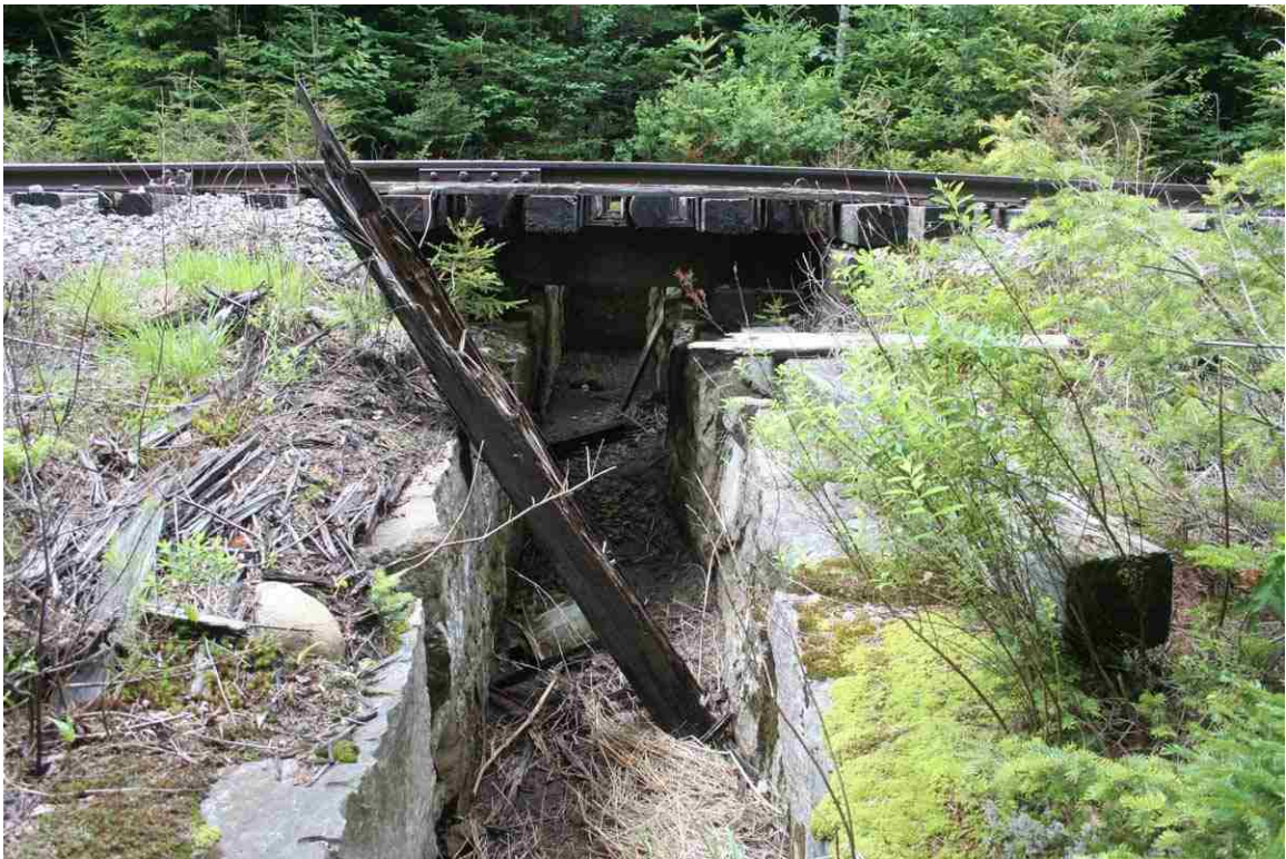
Photo # 76 description: Cattle pass, mp 134.02, Carroll. Wood stringer, 4' span. nd. North end. (1 of 3).
