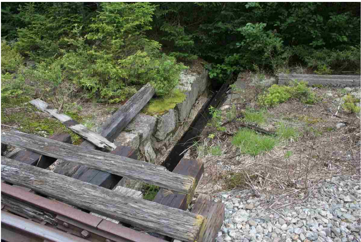
Photo # 78 description: Cattle pass, mp 134.02, Carroll. South end. (3 of 3).
