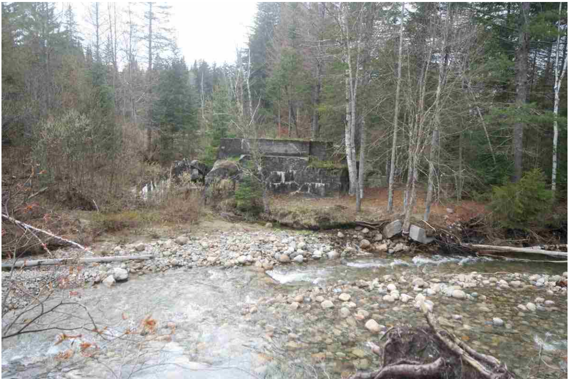
Photo # 38 description: Little River Bridge, Carroll. West abutment, view from east bank. (3 of 4).
