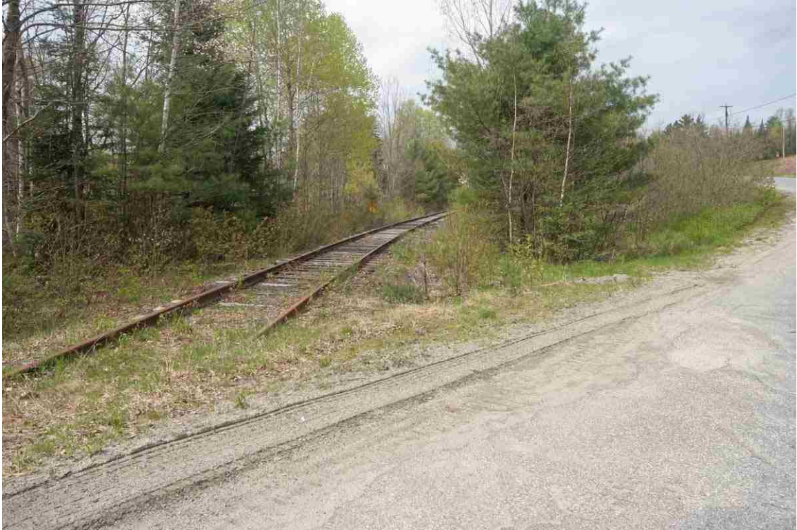
Photo # 1 description: Wing Road Crossing of Berlin Branch, Bethlehem. mp 120.70. Start of abandoned Mt. Washington Branch. Junction tracks removed. Branch line ran south along Wing Road.
