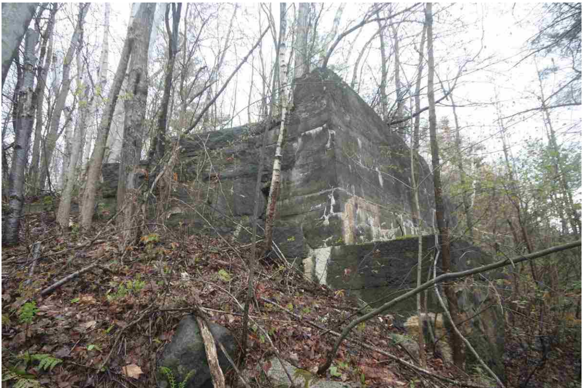
Photo # 56 description: Abutment of stone and concrete is all that remains of Bridge 129.80, evidently a timber trestle across Ammonoosuc R. floodplain, north of river and south of US302. Carroll. nd.
