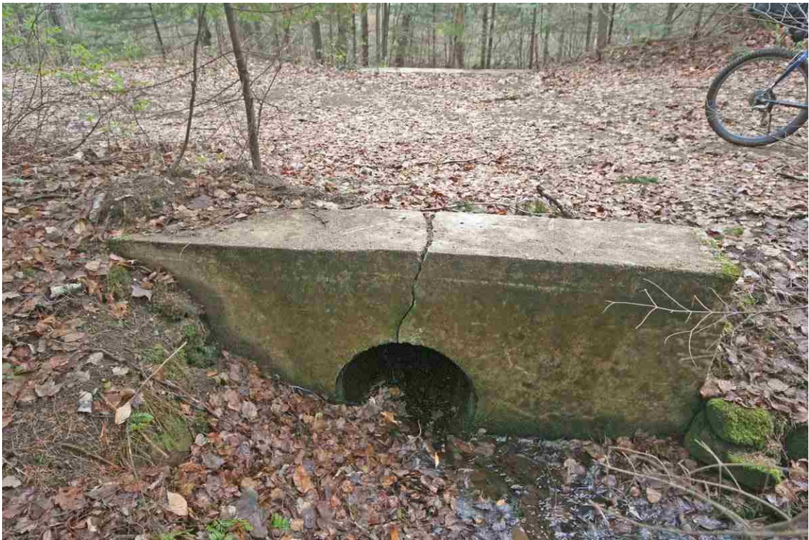
Photo # 46 description: Culvert 129.34, Carroll. Cast iron pipe, 24", with concrete headwalls.
