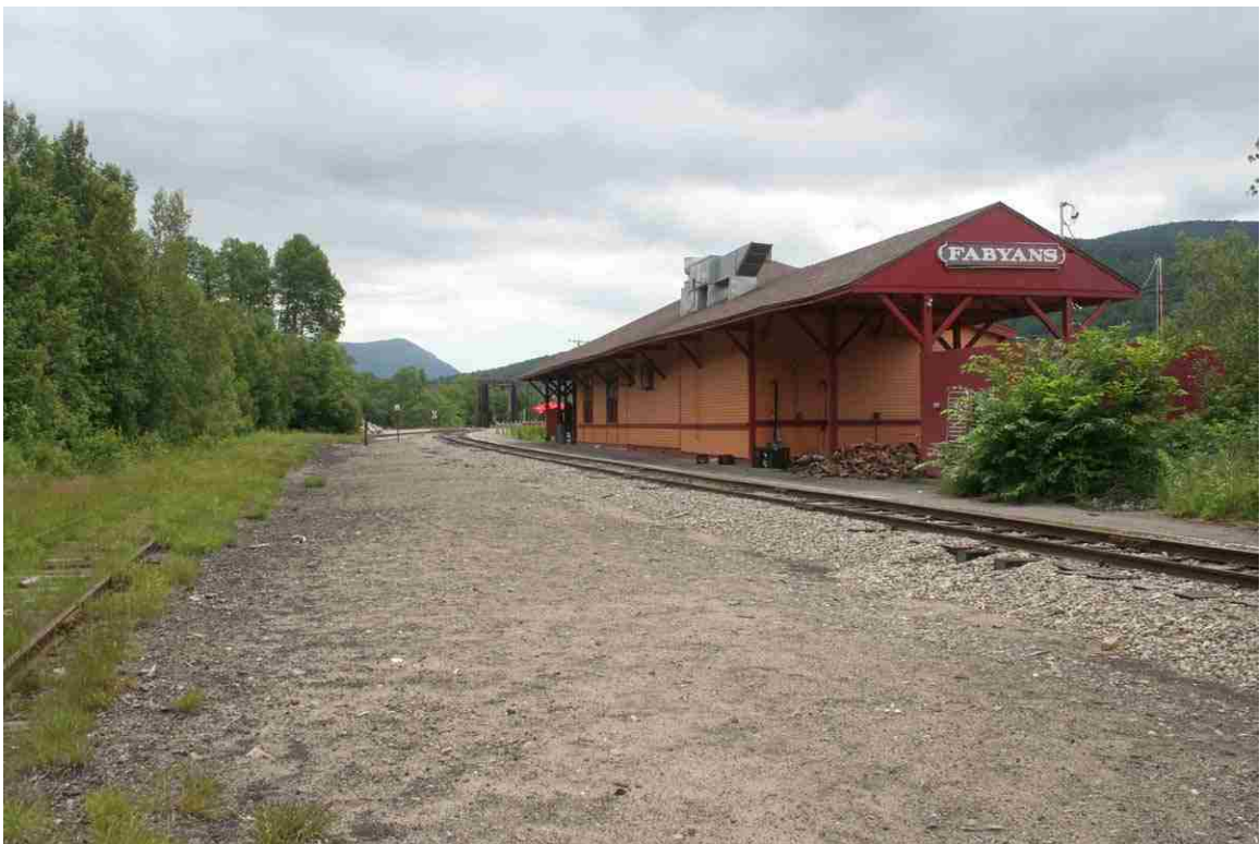
Photo # 80 description: Fabyans Station, mp 134.20, Carroll. North side facing tracks. (2 of 2).
