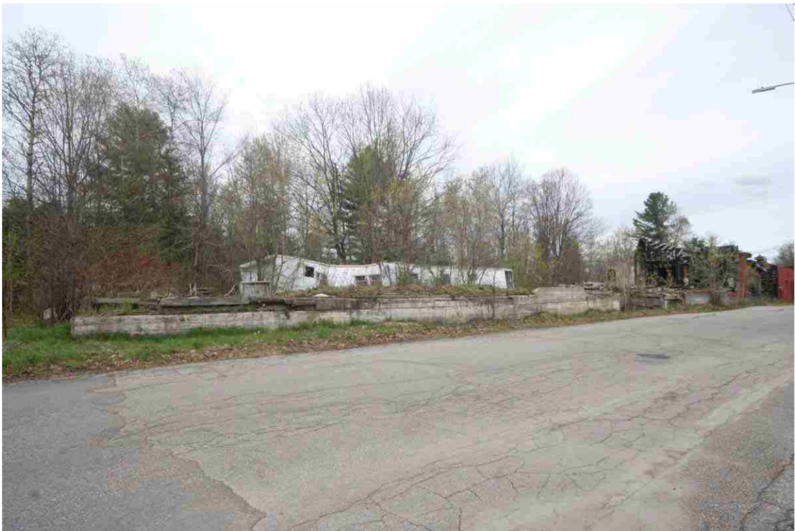
Photo # 50 description: Concrete block foundation of demolished railroad associated building on Depot St., Lancaster. ~mp 136.75. Possibly remains of B&M Depot? More research needed.
