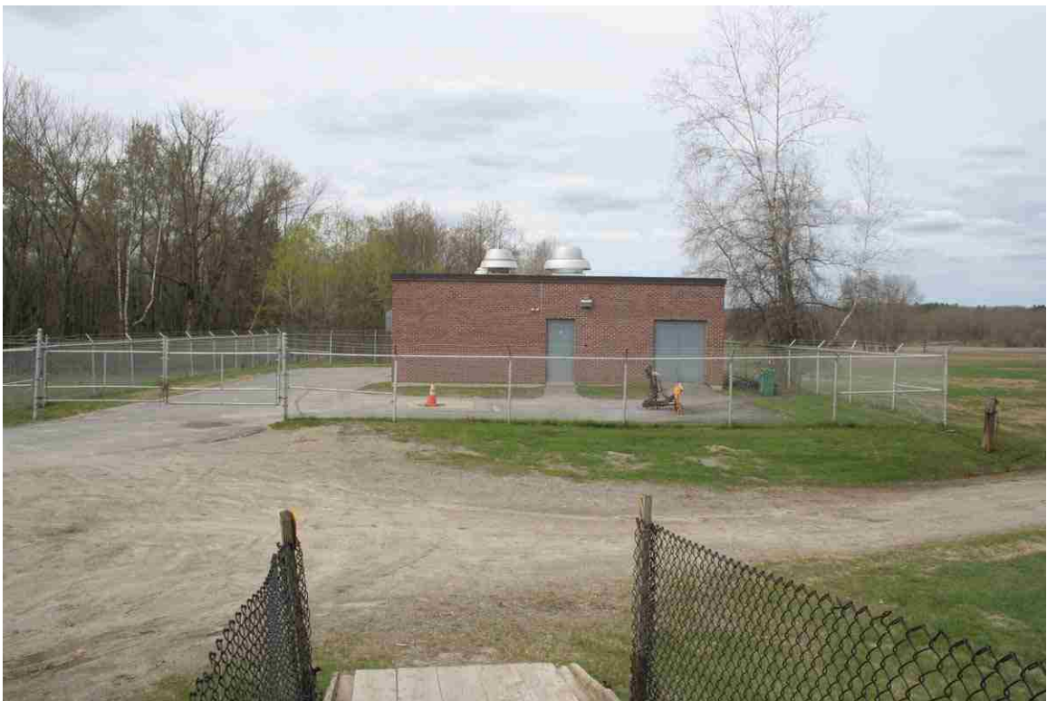
Photo # 38 description: Lancaster Water Treatment plant built on ROW at foot of Heath St. on Israel R. ~mp 136.00. (2 of 2). Photo from Israel R. snowmobile bridge built next to ROW crossing.
