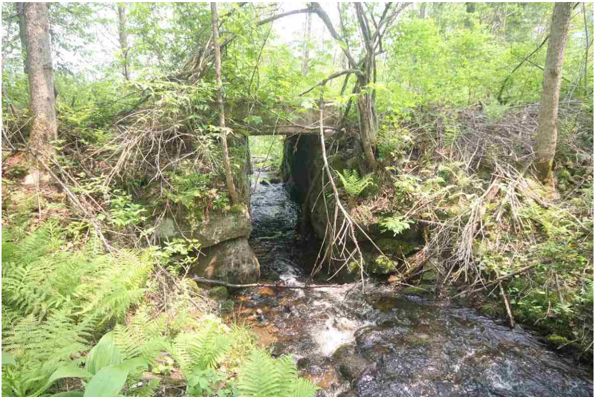
Photo # 3 description: Bridge 126.81. Upstream side. (2 of 2).
