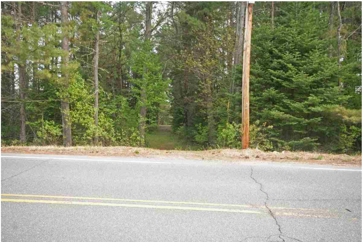
Photo # 27 description: ROW/Trail looking north at Whitefield Road, NH142, Dalton, mp~130.1. ROW ends, becomes private property but trail continues in rough condition.
