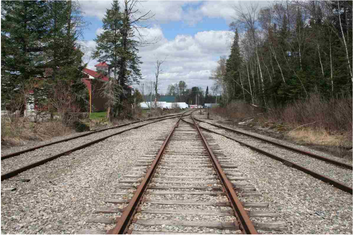
Photo # 59 description: MC lines approaching Coos Junction, Lancaster. Line runs behind commercial/industrial buildings along east side of Summer Street.
