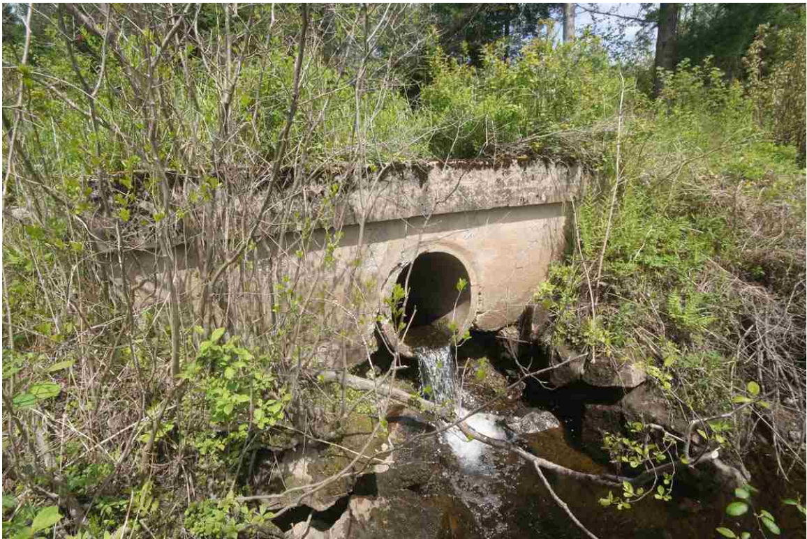
Photo # 21 description: Culvert 128.90, Dalton. Akron pipe, 30" with concrete headwalls. nd.
