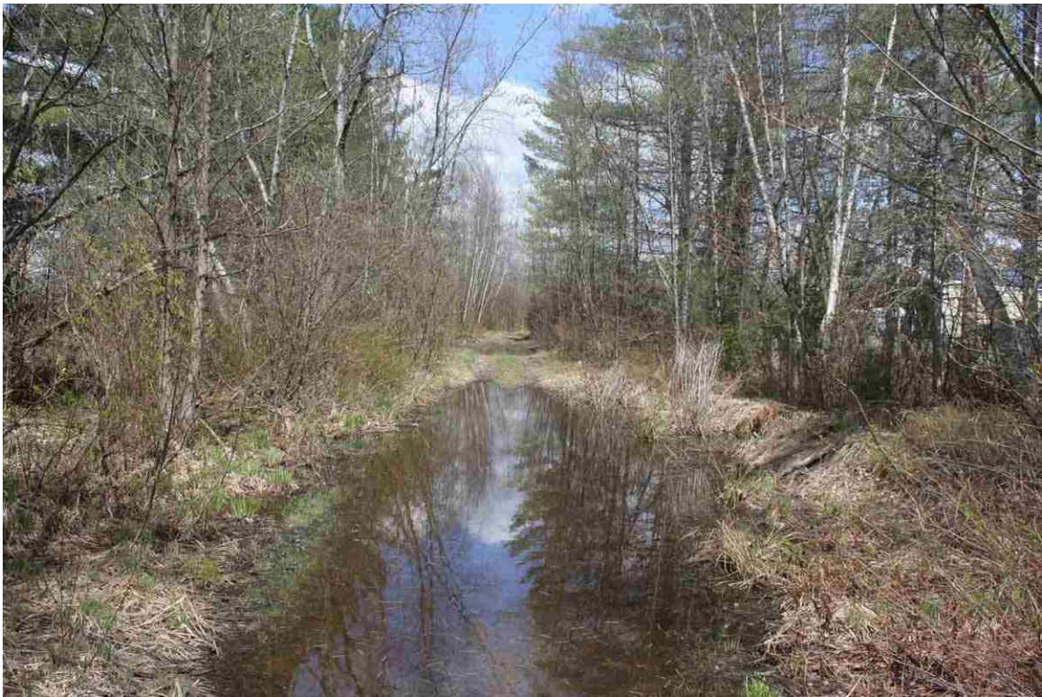
Photo # 58 description: Character of ROW approaching Coos Junction, running behind industrial/commercial buildings along west side of Summer St., Lancaster. mp~137.25.
