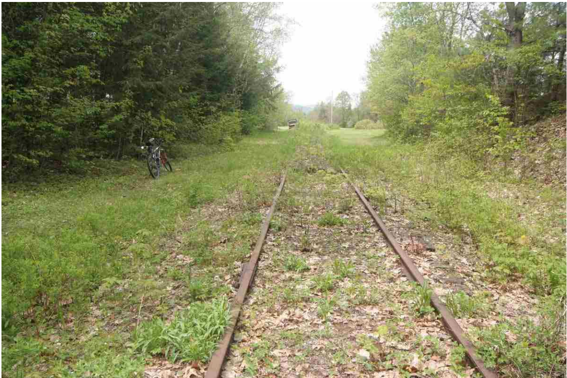
Photo # 16 description: Scotts Junction, view south. Extant MC tracks in foreground; bicycle is parked on slightly raised bed of B&M ROW just before it crosses the MC line. (2 of 2).
